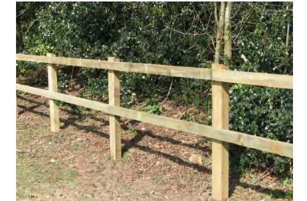
TIMBER POST AND RAIL FENCING
