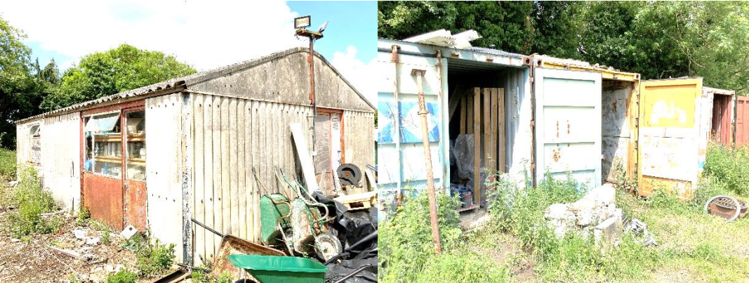
Corrugated asbestos sheet building to be demolished (left) and shipping containers (right)
