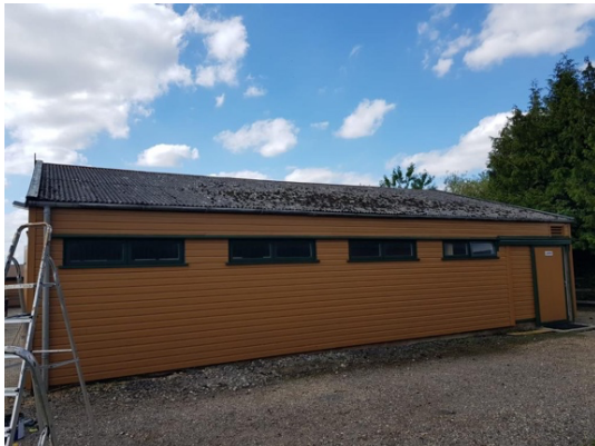
Existing Building windows.
