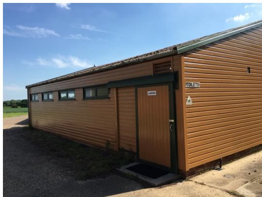
Existing Building exterior.
