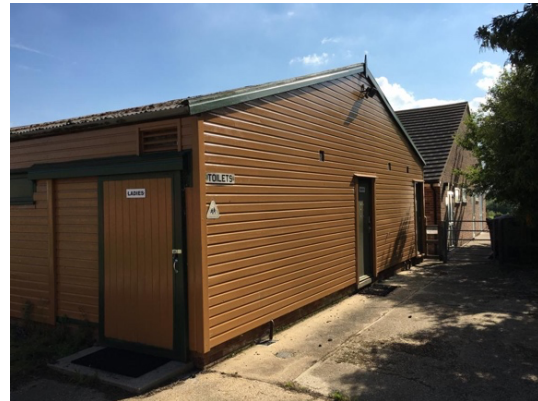
Existing Building toilet doors.
