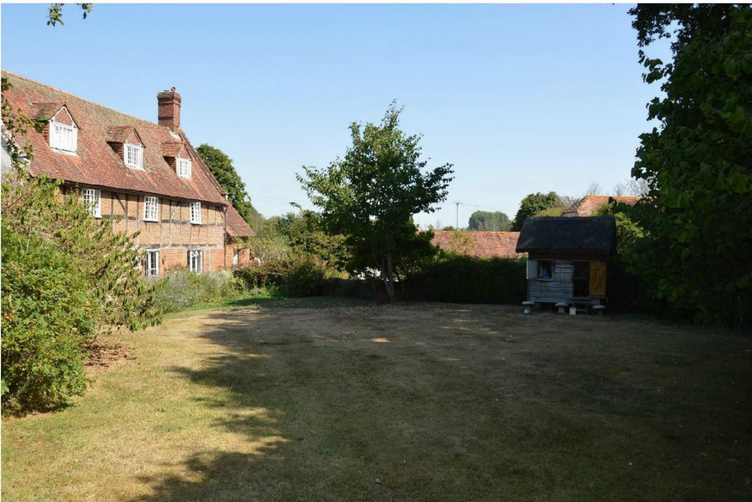
Plate 4. Short mown grass where the extension will be built.
