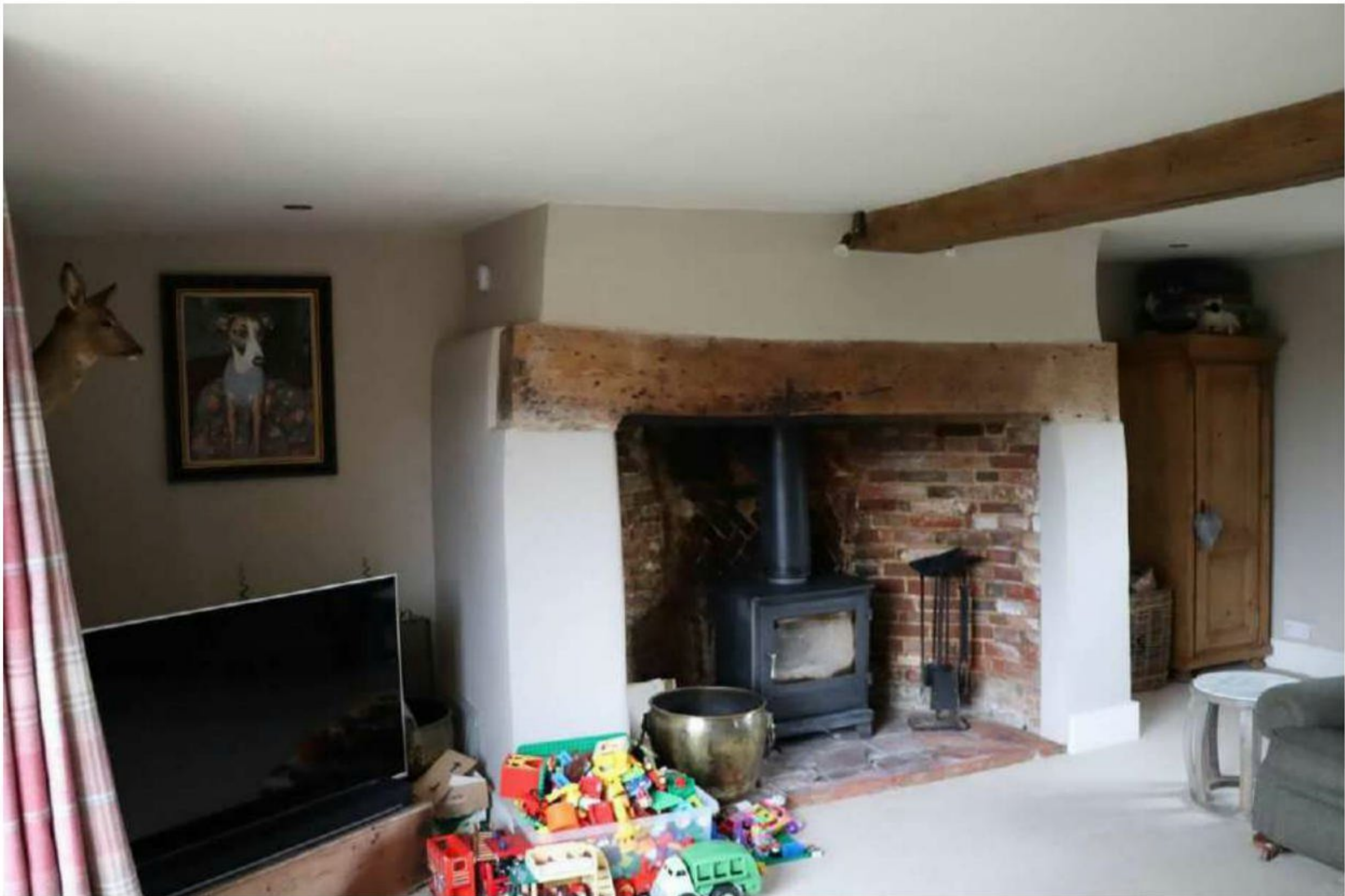
Plate 19: Reopened inglenook on SW wall of G3
