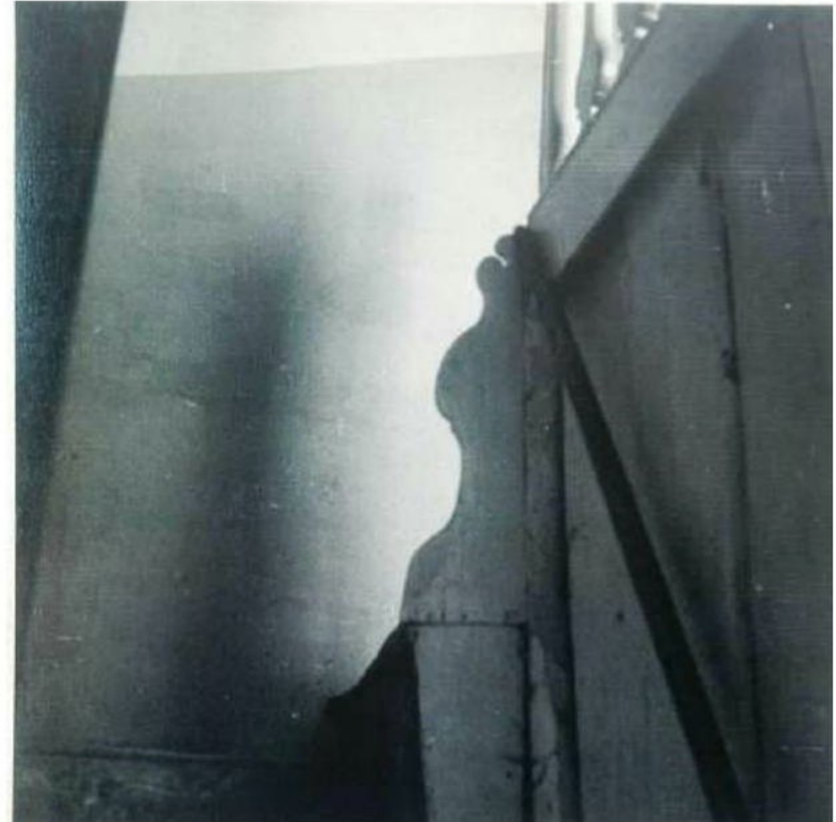
Y1: Detail of carved wooden piece where the staircase turns through 90 degrees up to the first floor (this was not retained)
