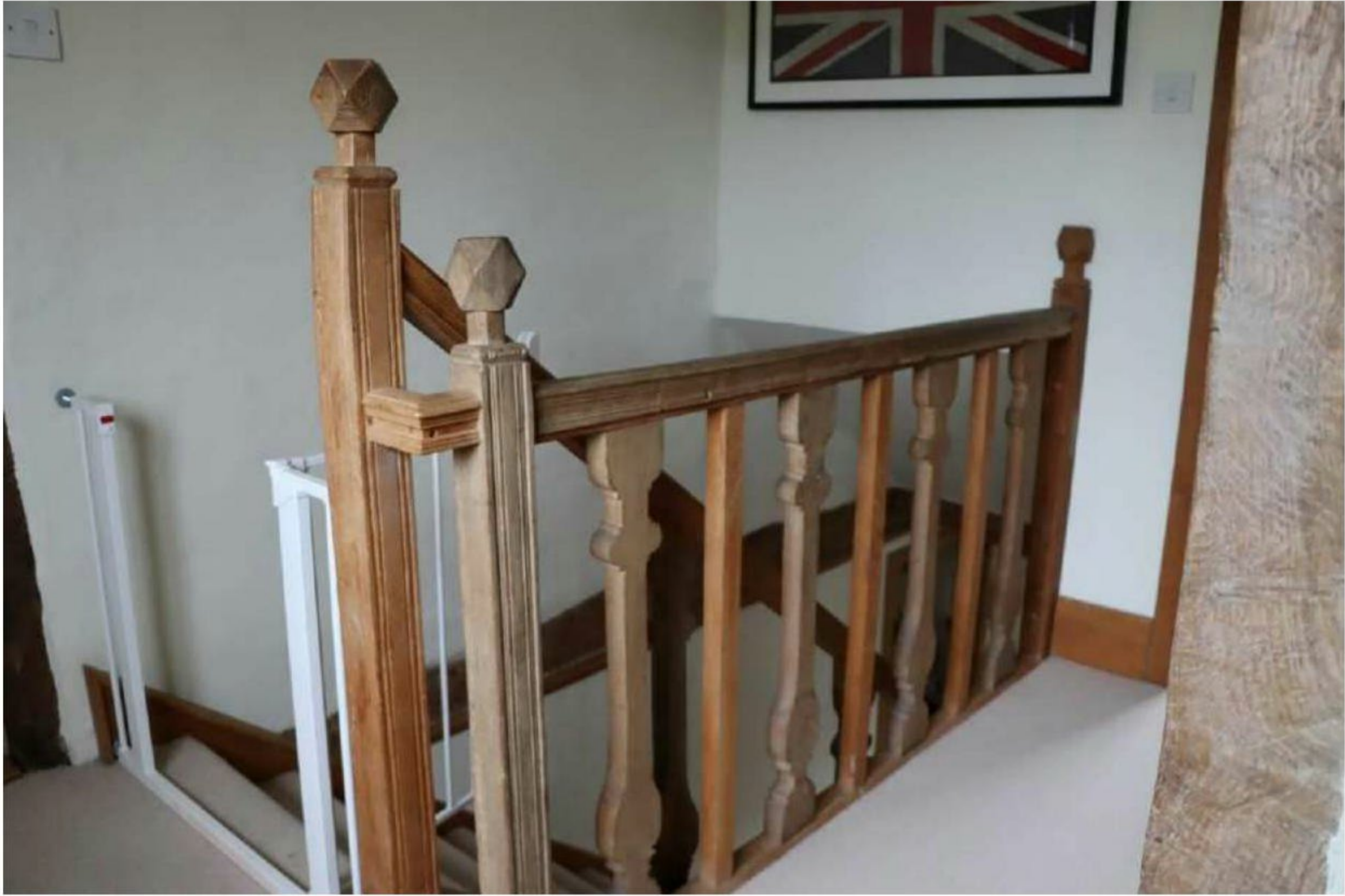
Plate 17: F1 (first-floor landing): note original newel and taller replica, original section of handrail and splat balusters
