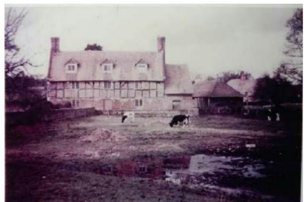
L: Rear elevation before alterations
