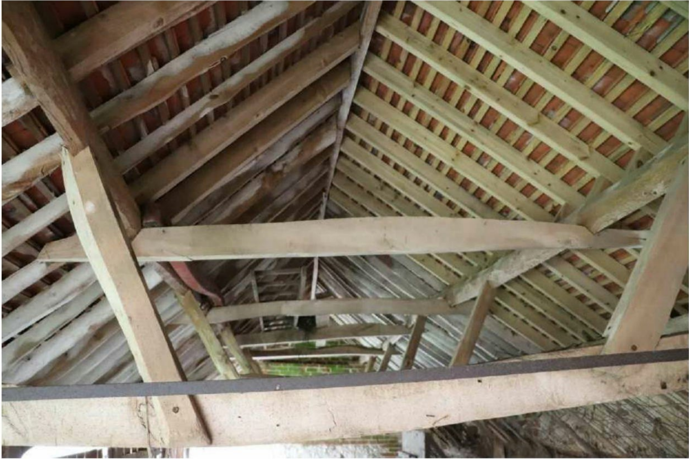
Plate 47: Building B – detail of roof structure
