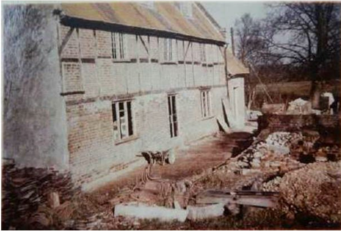
S: Rear elevation with new French doors
