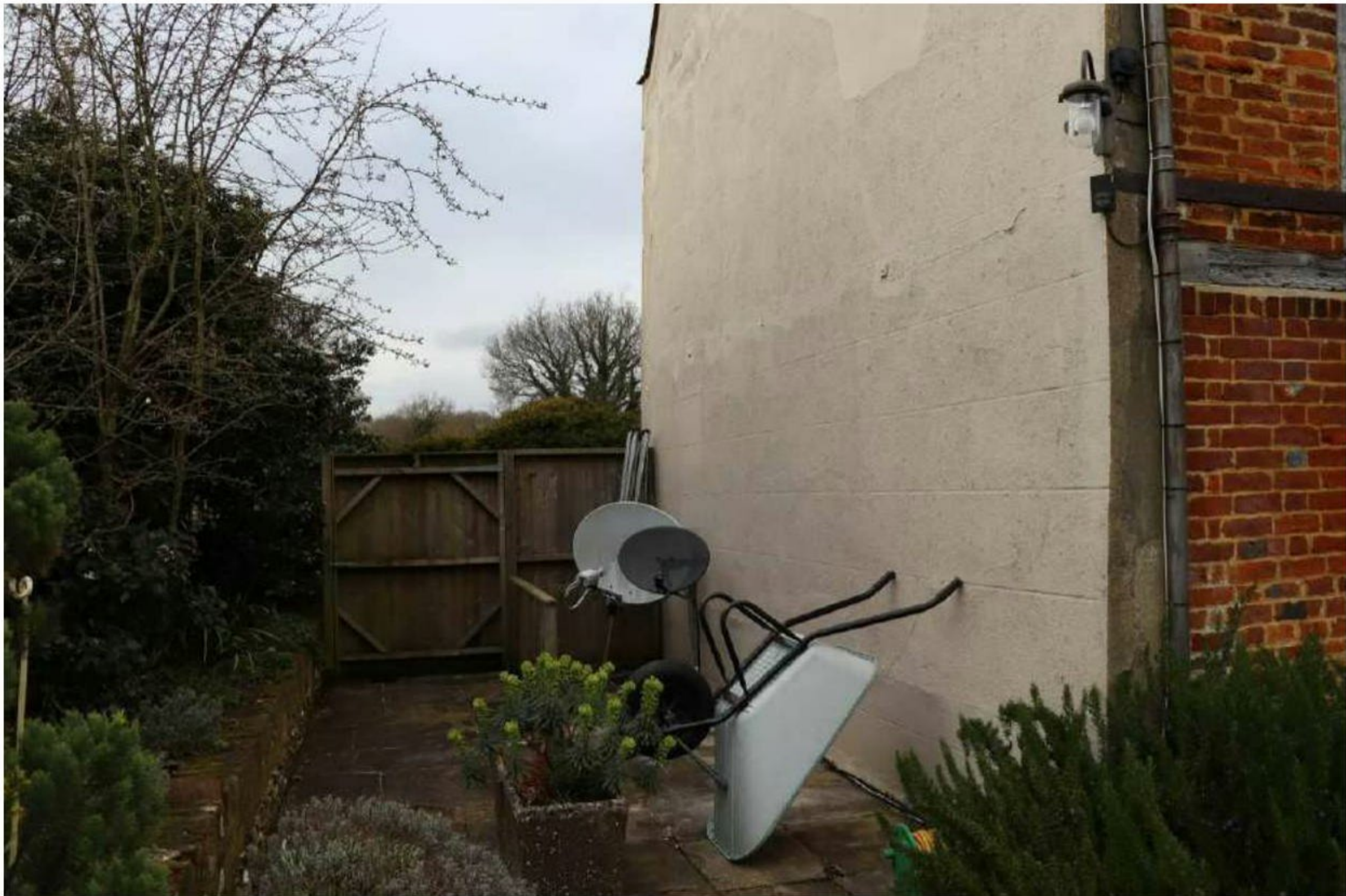
Plate 11: Base of the SW gable end, from where an earth bank was removed in 1957
