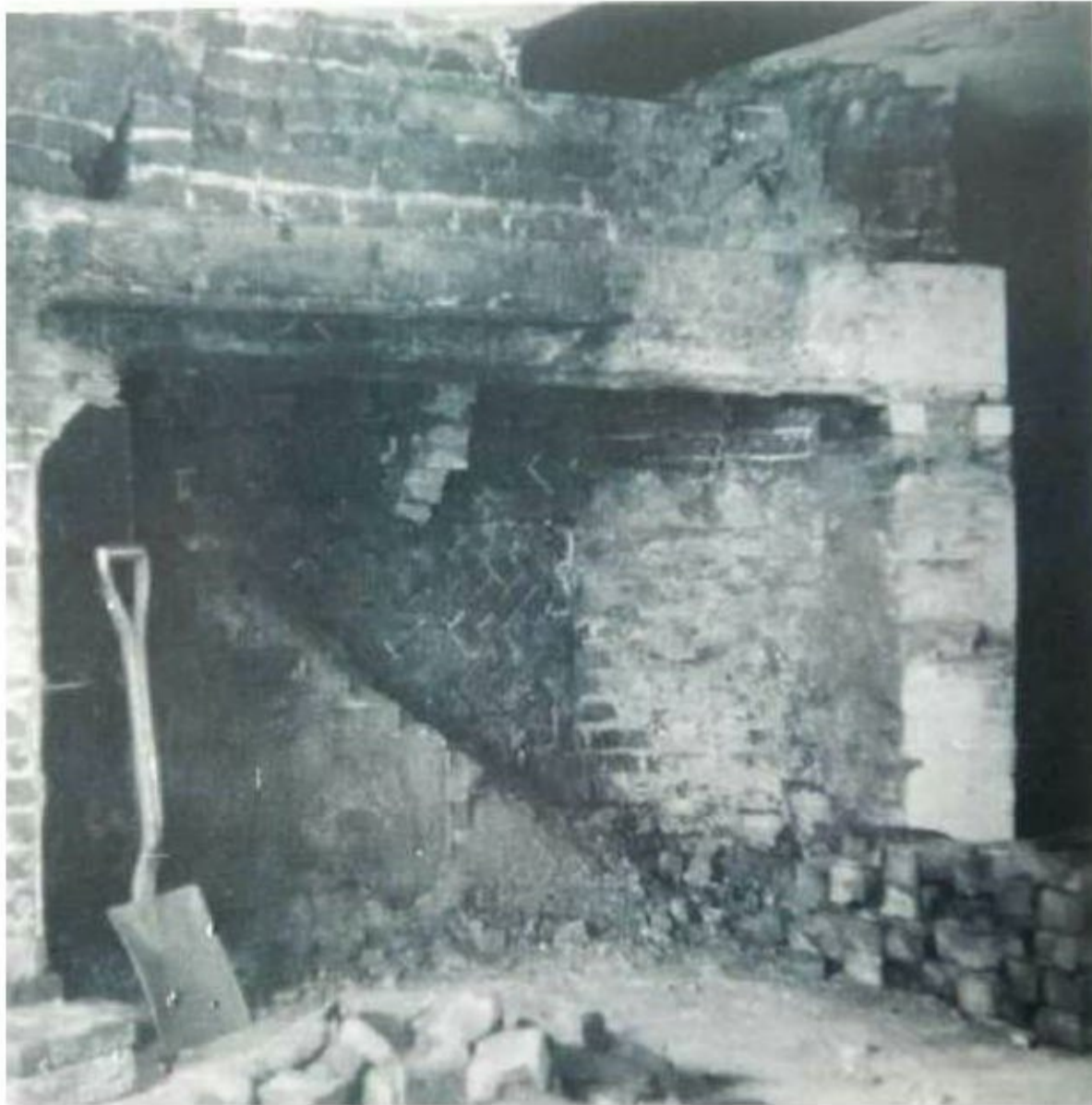
I1: G3: detail of reopened inglenook in G3
