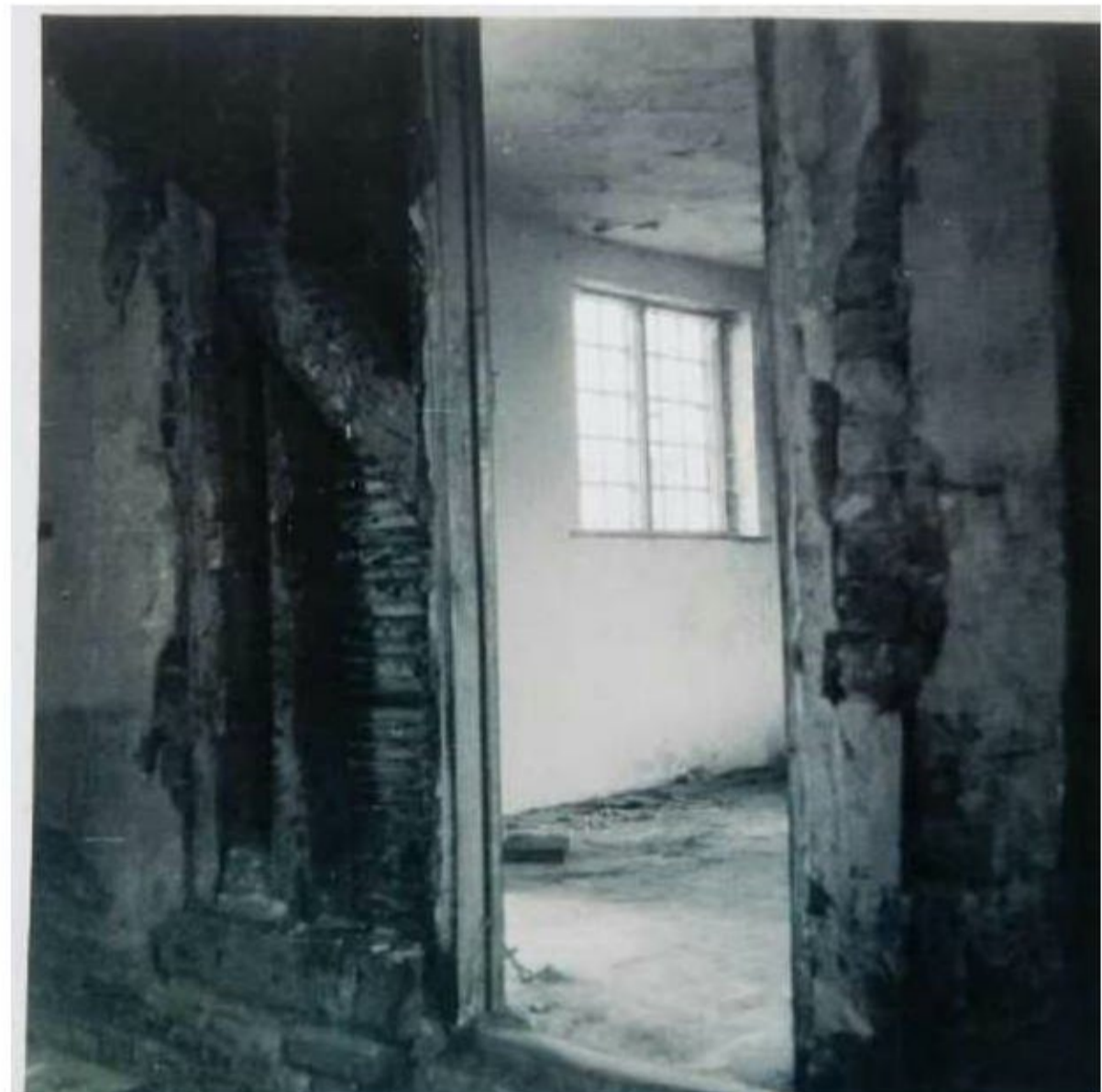
G1: Looking N from central bay into G4 (the timber-framed wall was yet to be demolished)
