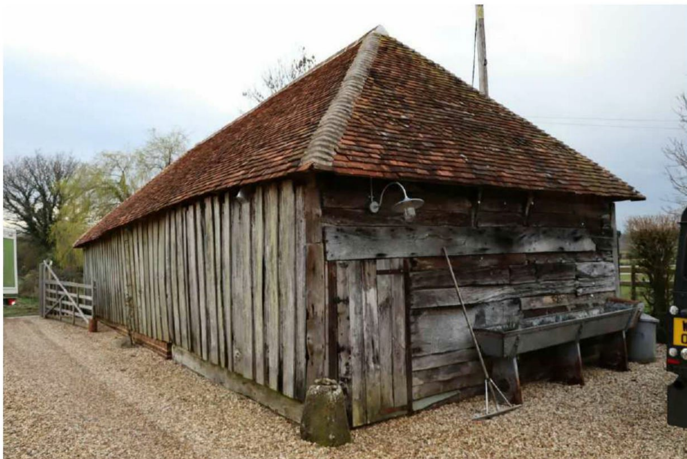
Plate 42: Cartshed (Building A) – long S elevation and E rear end – the building appears originally to have extended further E
