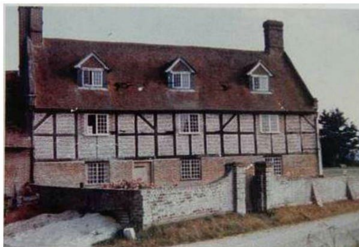
F: Front elevation - September 1959, following works
