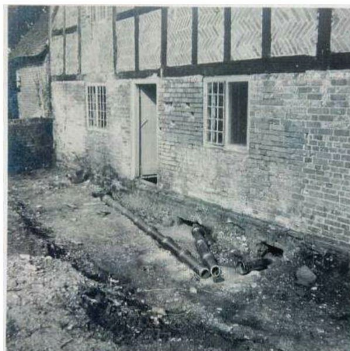
E: Front elevation, drainage works
