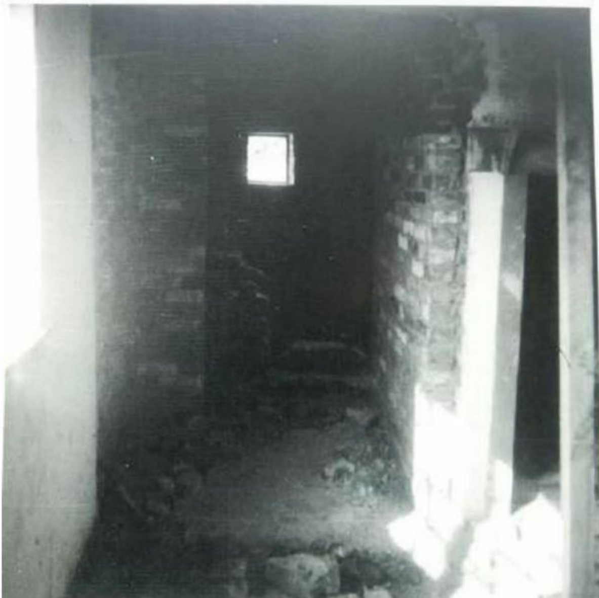
T1: Following demolition of bread oven, looking NE from G4 into G5 in 'brewhouse' addition
