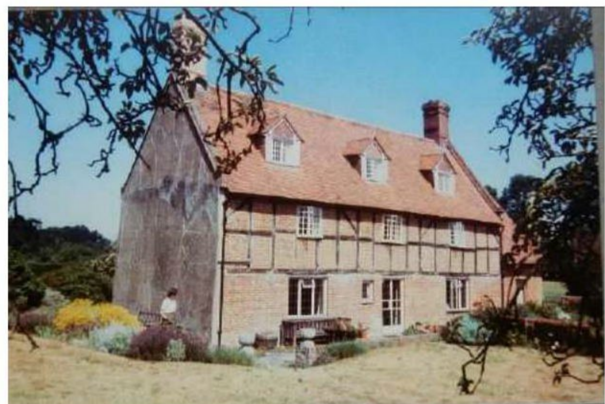
X: SW gable end and rear elevation (1976)
