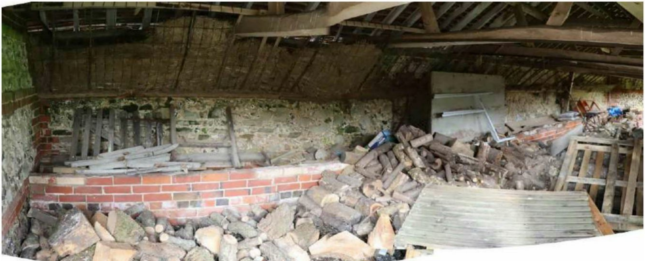
Plate 48: Building B – interior, looking to rear wall with feeding trough and manger
