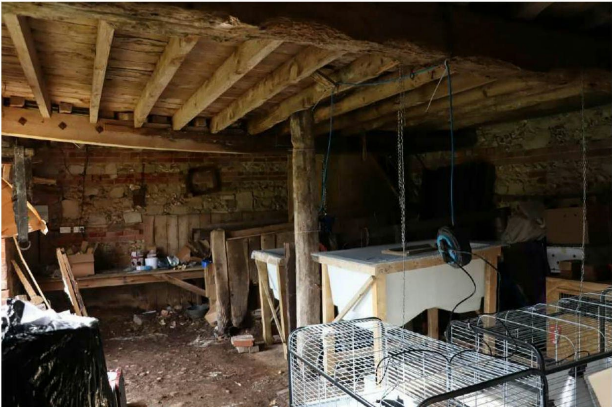
Plate 50: Building C – interior, looking W
