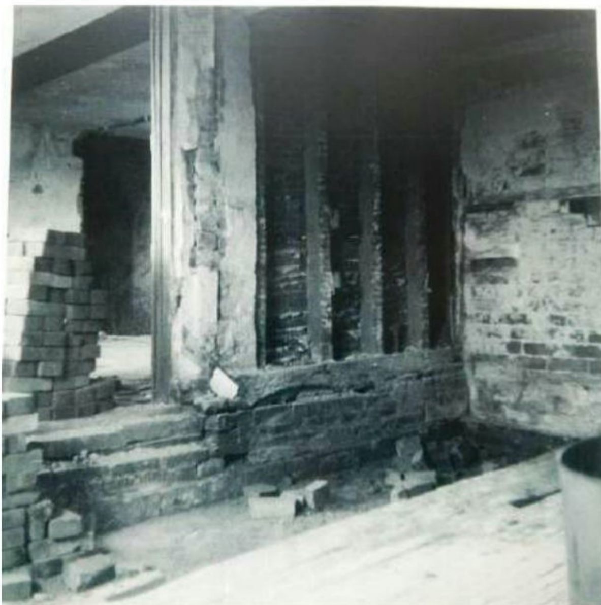
E1: Similar viewpoint as above, further to the right: looking towards remains of timber-framed wall. The brick wall to right was to be removed.
