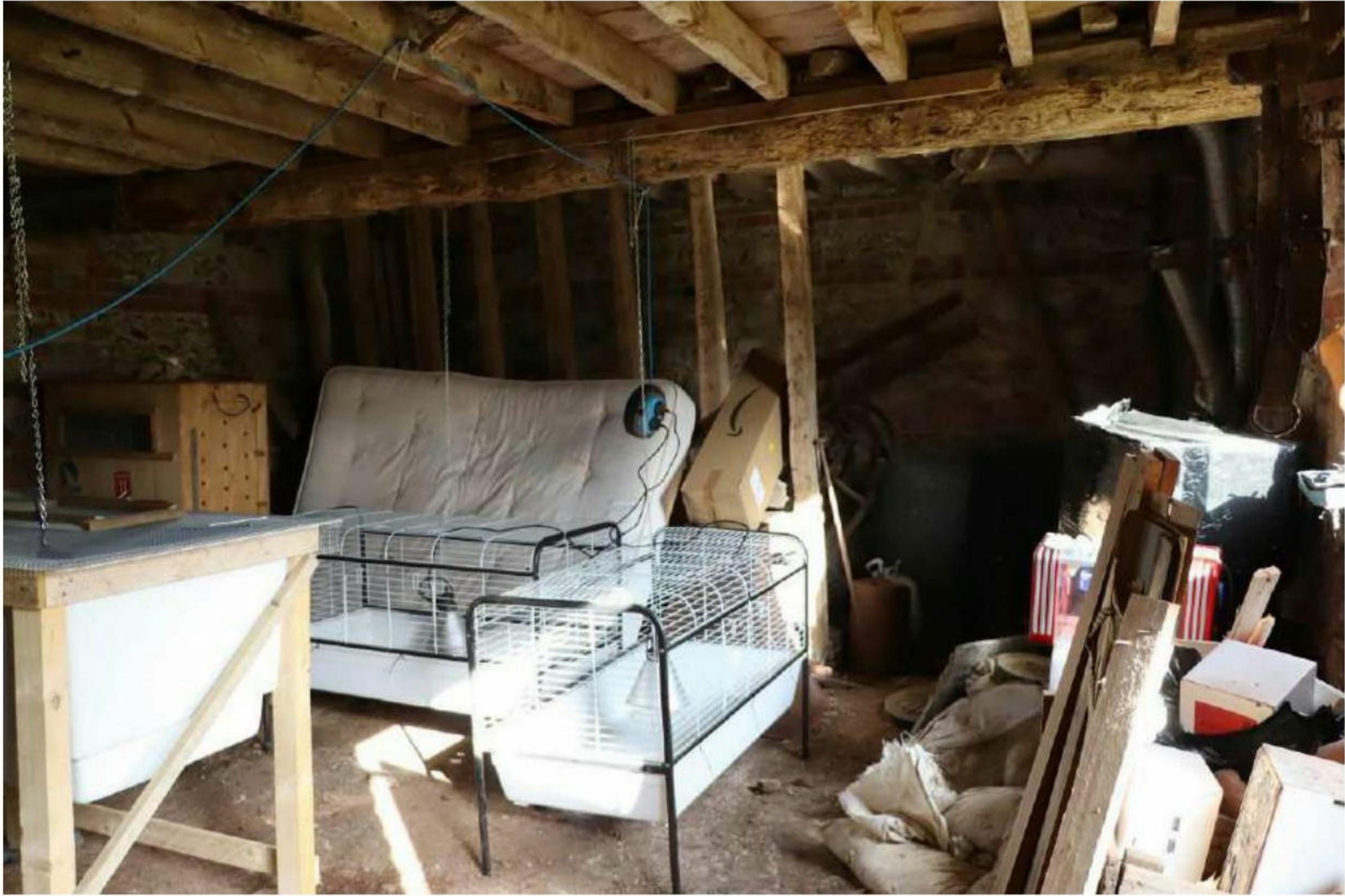
Plate 51: Building C – interior, looking E towards former partition in E end bay, and ladder to hay loft
