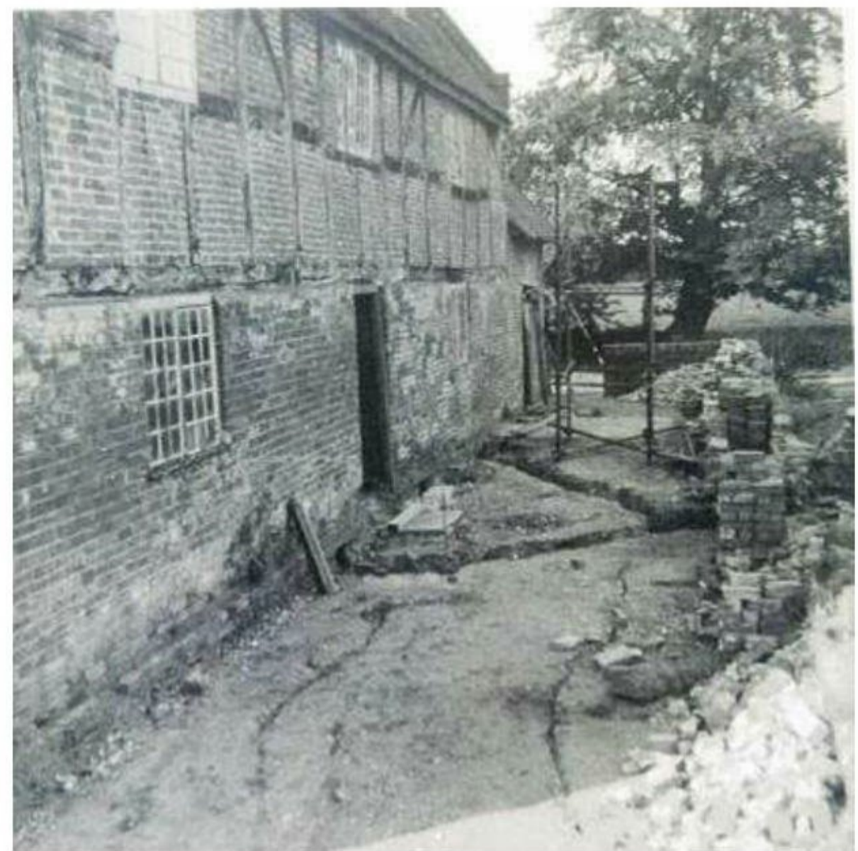
Q: Looking NE along rear elevation
