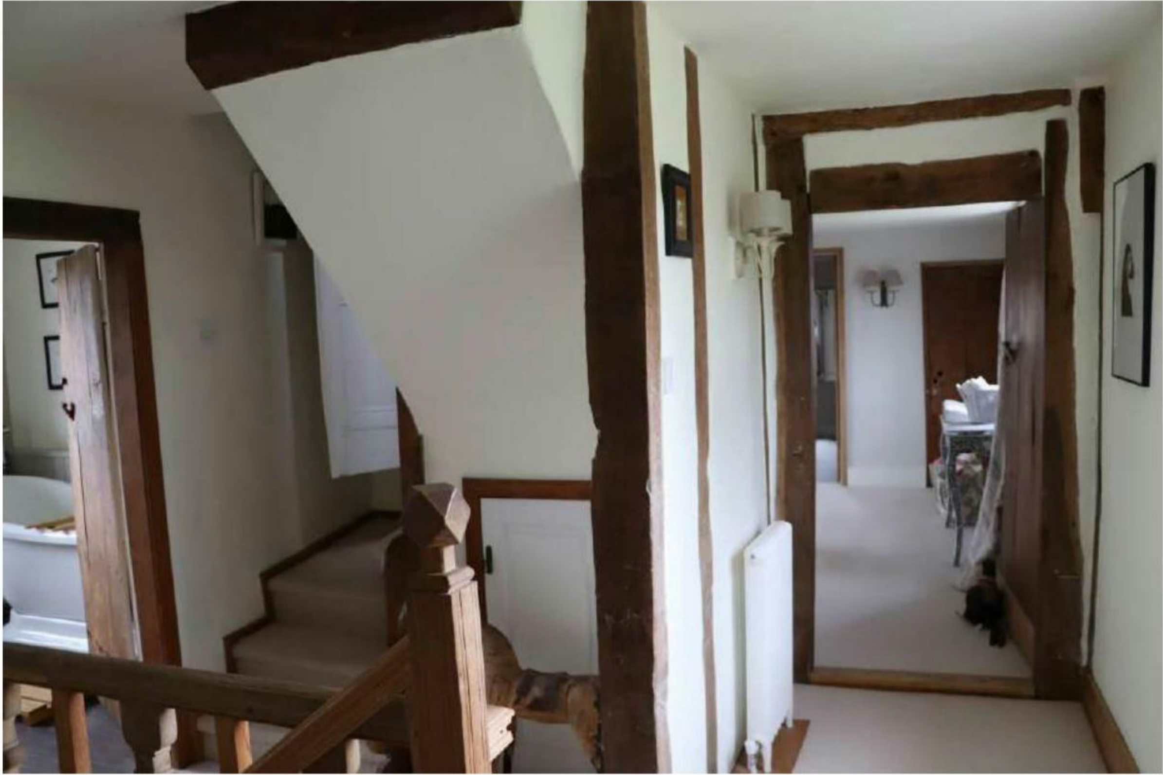
Plate 25: F1 (first-floor landing), looking NE (underside of attic stairs to left)
