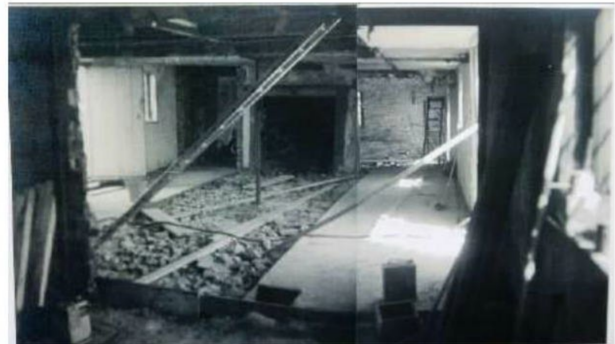
M1: Looking NE from G3 through partially demolished wall where staircase has been removed in central bay across into G4
