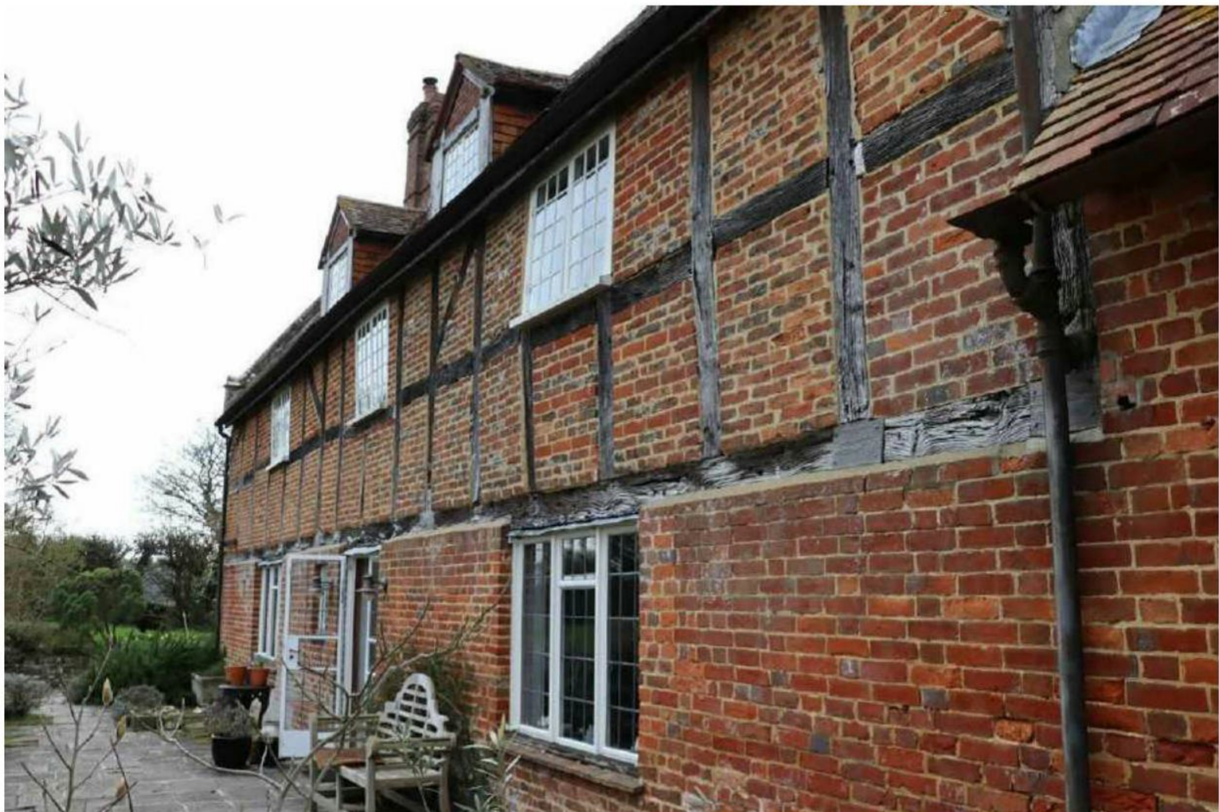
Plate 8: Rear elevation; note projection of ground-floor brickwork from the original building plane, with enlarged window opening in foreground and French doors
