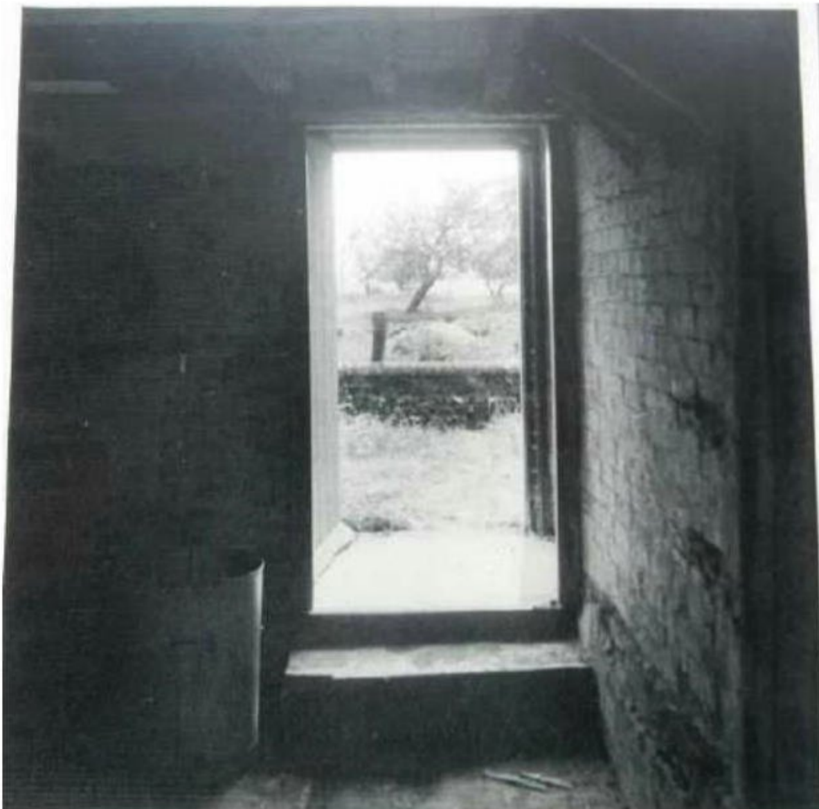
Z: Looking SE past old staircase enclosure (right) through internal doorway onto rear passage and rear entrance (viewpoint now the part of G4 in central bay)
