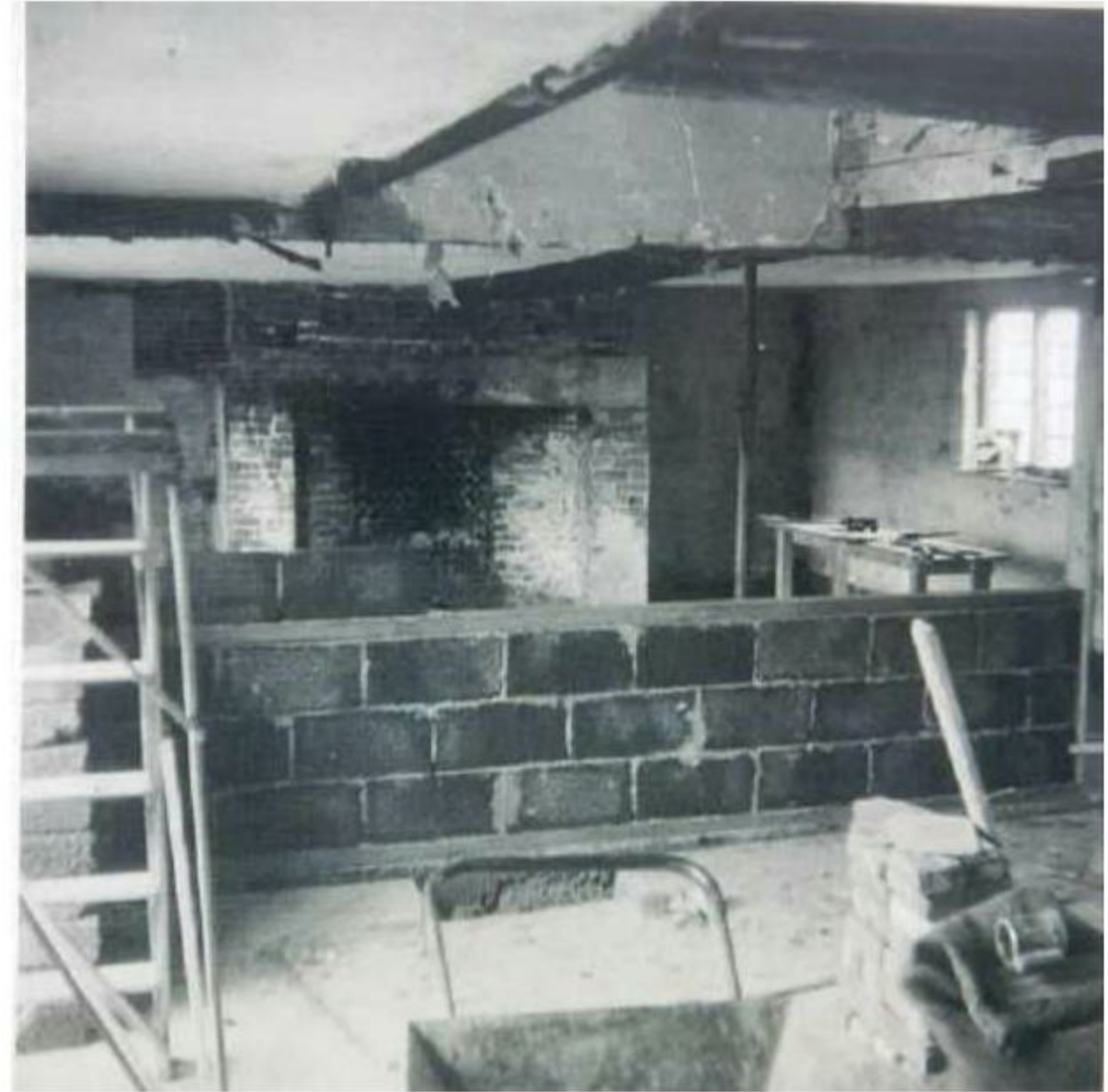
L1: Similar viewpoint to K1 above, looking SW into G3, but from within the central bay: the brick wall is in the process of being replaced with the new concrete block wall
