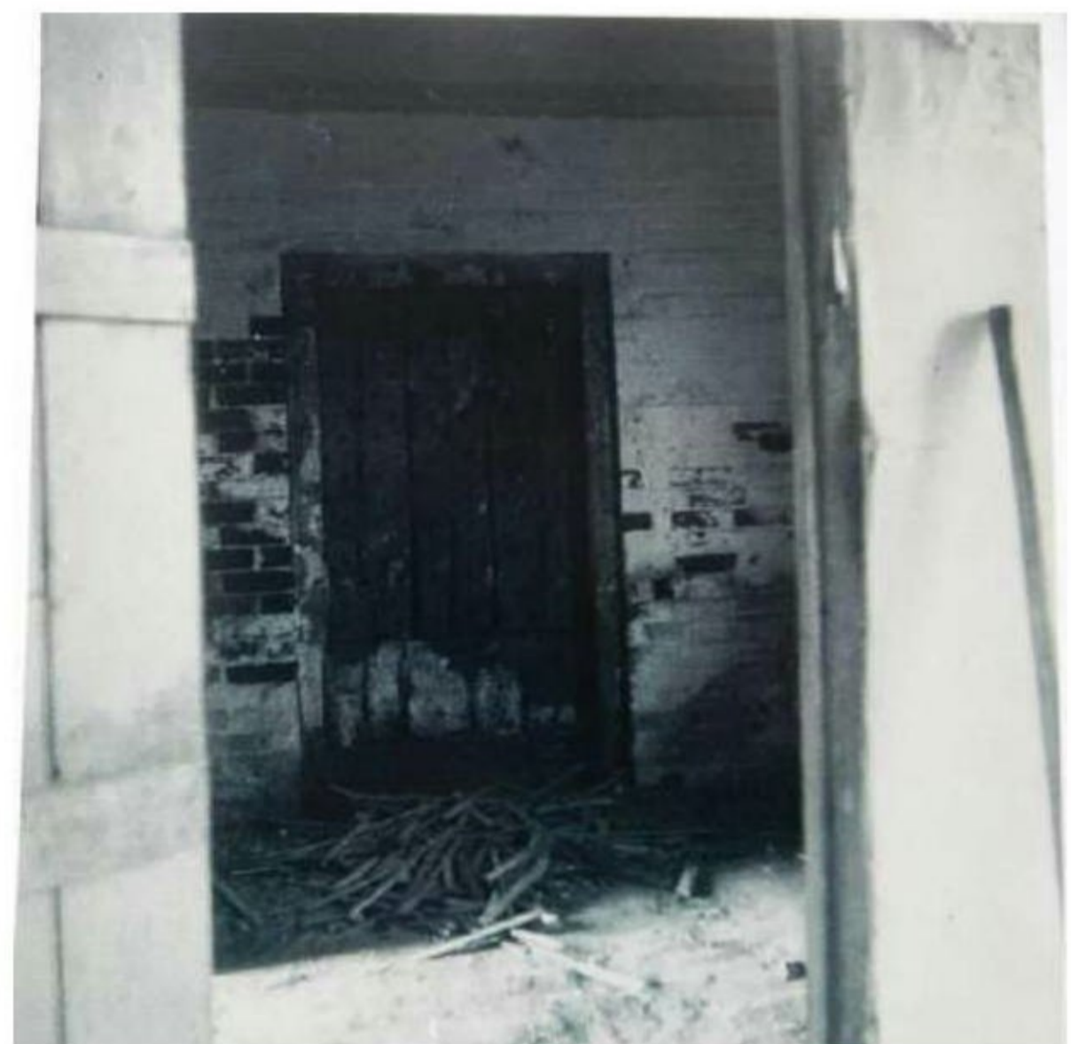
V1: Old double-thickness door in undetermined location. The nature of the brickwork suggests somewhere in the central bay.
