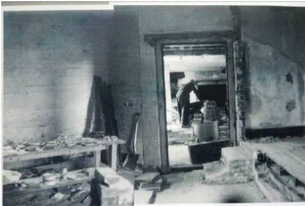
J1: Looking NE from G3 through doorway into central bay and beyond into G4: to the right a wall stood on the alignment of the higher floor level, said to be C19 and dividing the NW part of G3 (dairy) from the SE part (parlour)
