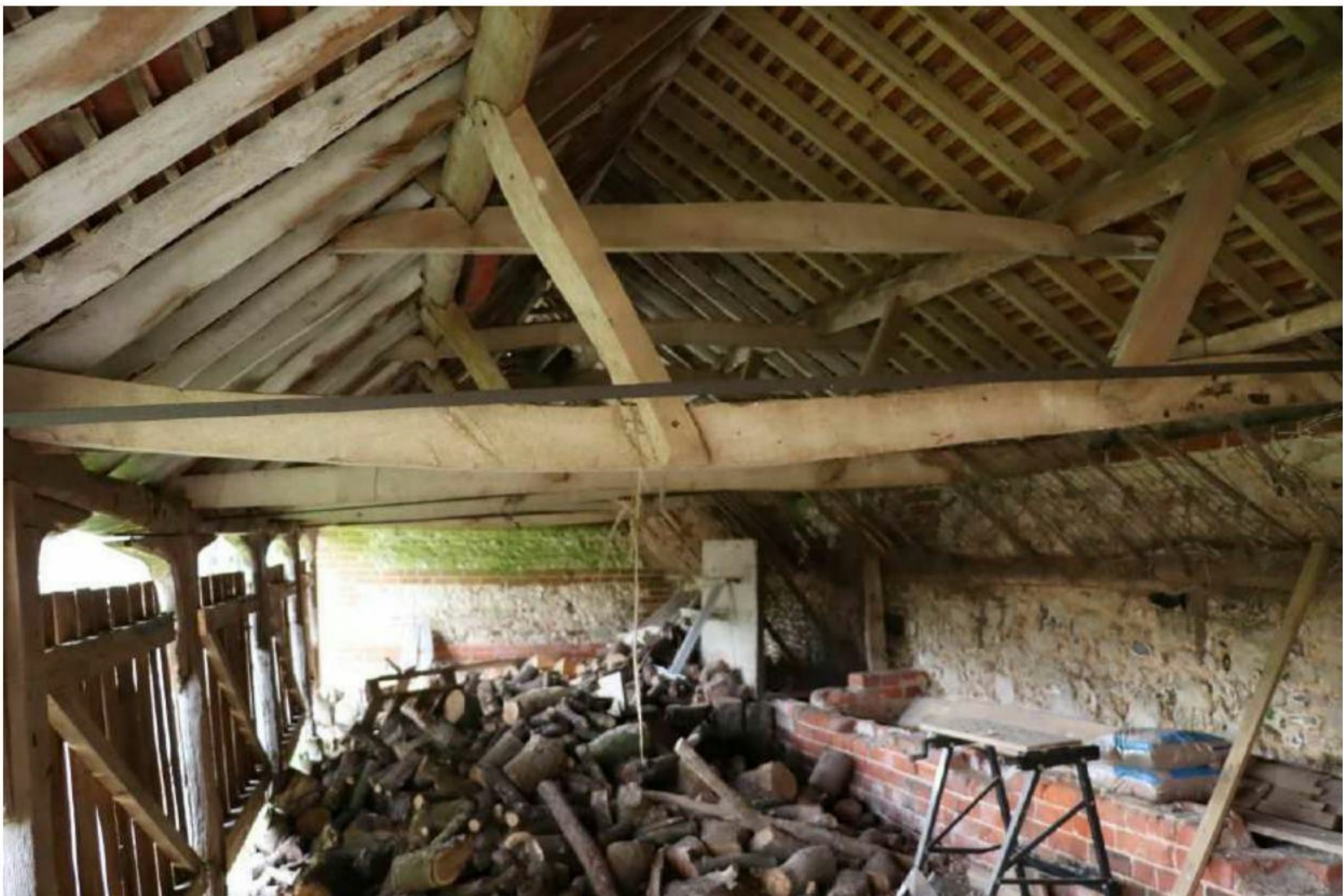
Plate 46: Interior of Building B, looking W
