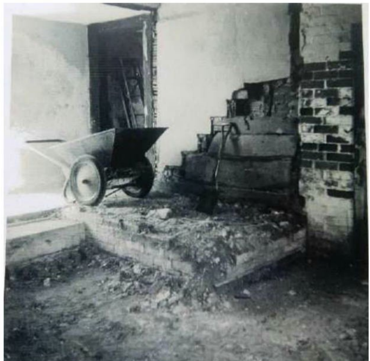
C1: Similar viewpoint to above following further demolition of staircase
