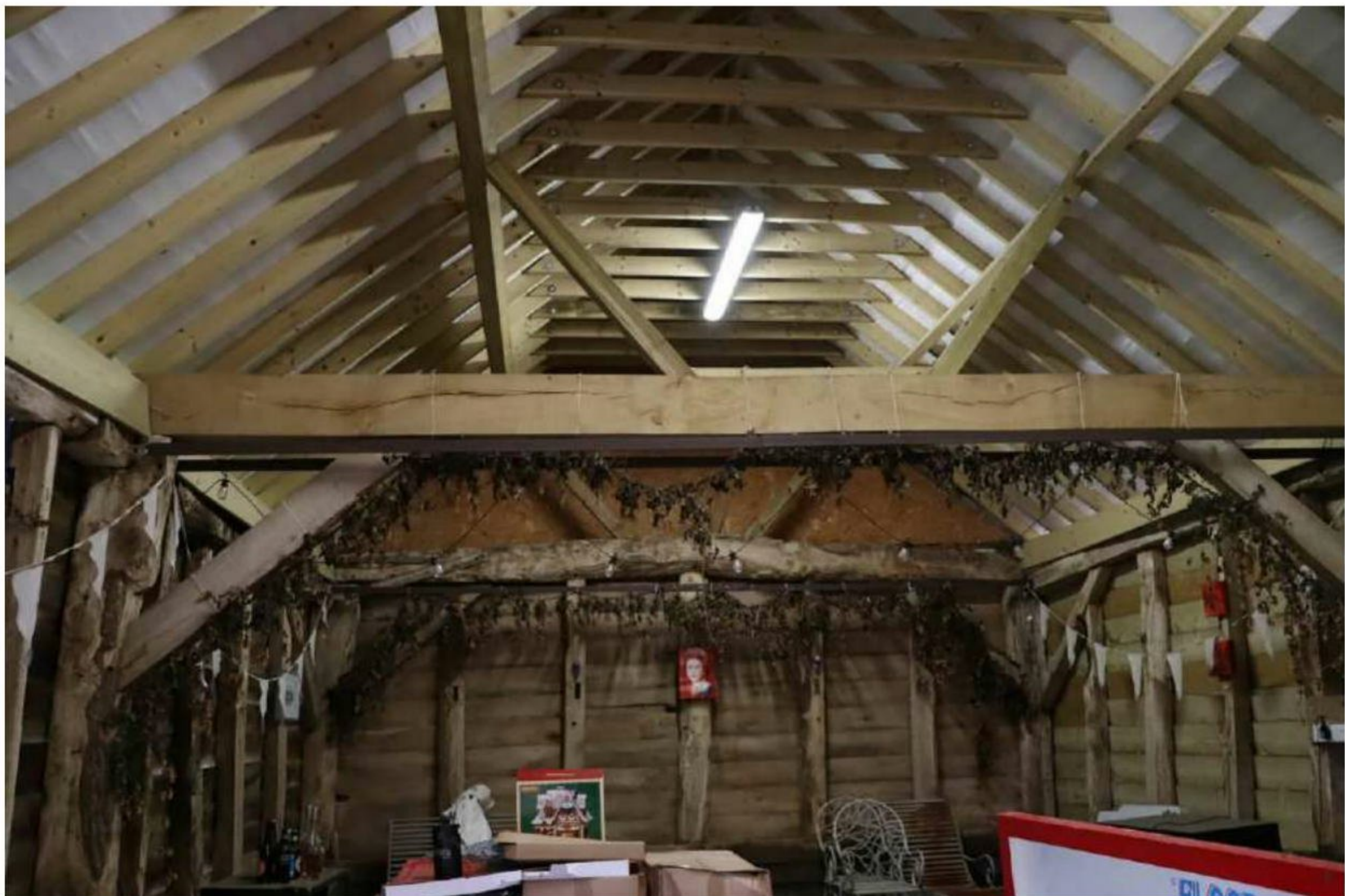
Plate 58: Building D: interior, looking W
