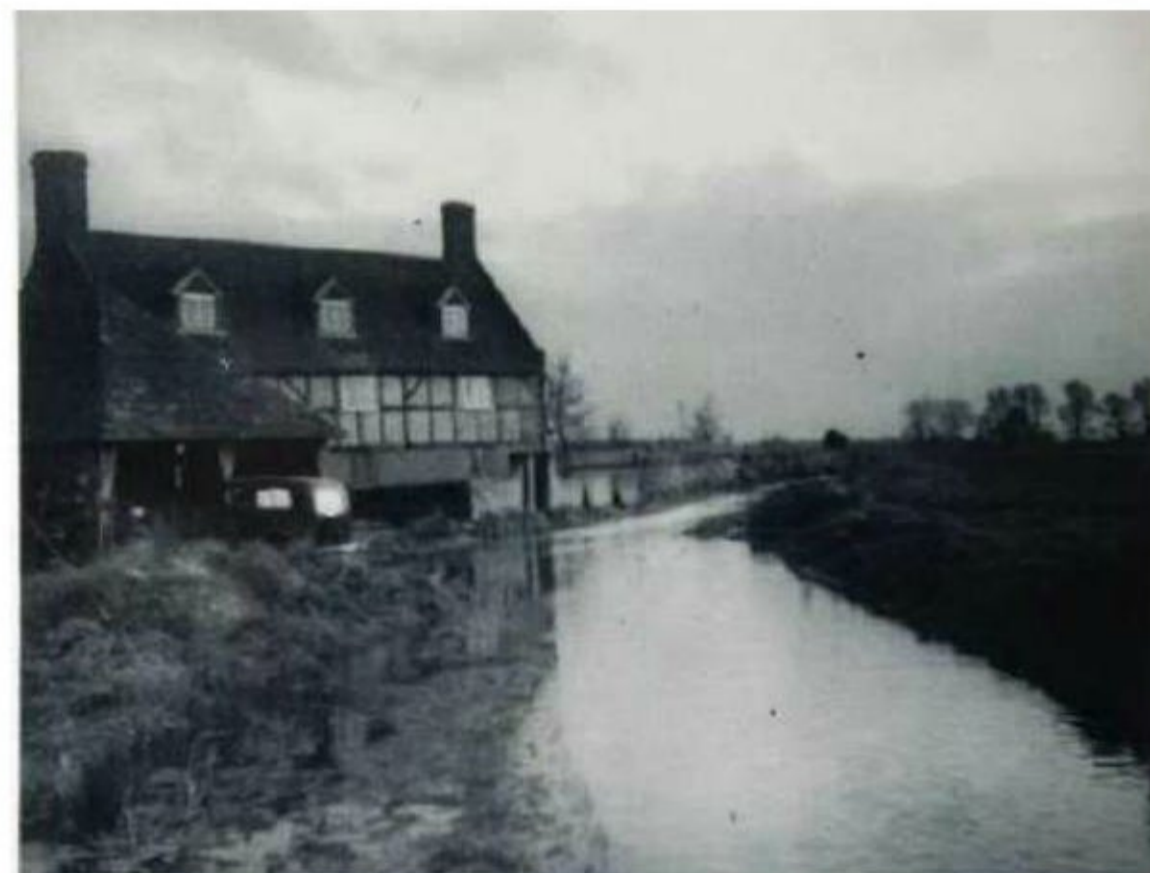
D: Looking S along a flooded Flood Street towards the farmhouse
