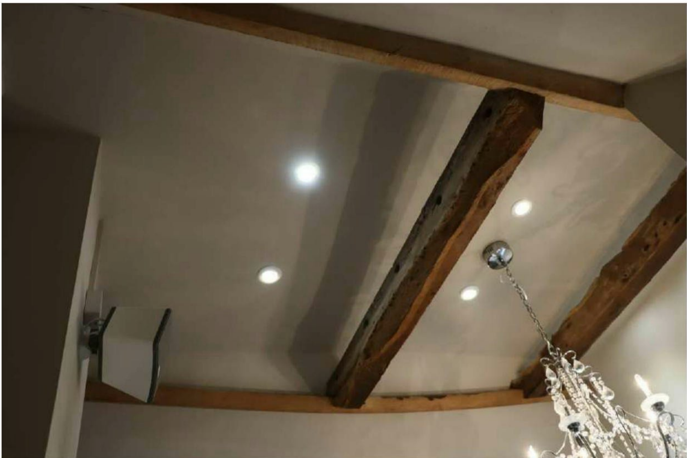
Plate 32: Exposed roof timbers in F4
