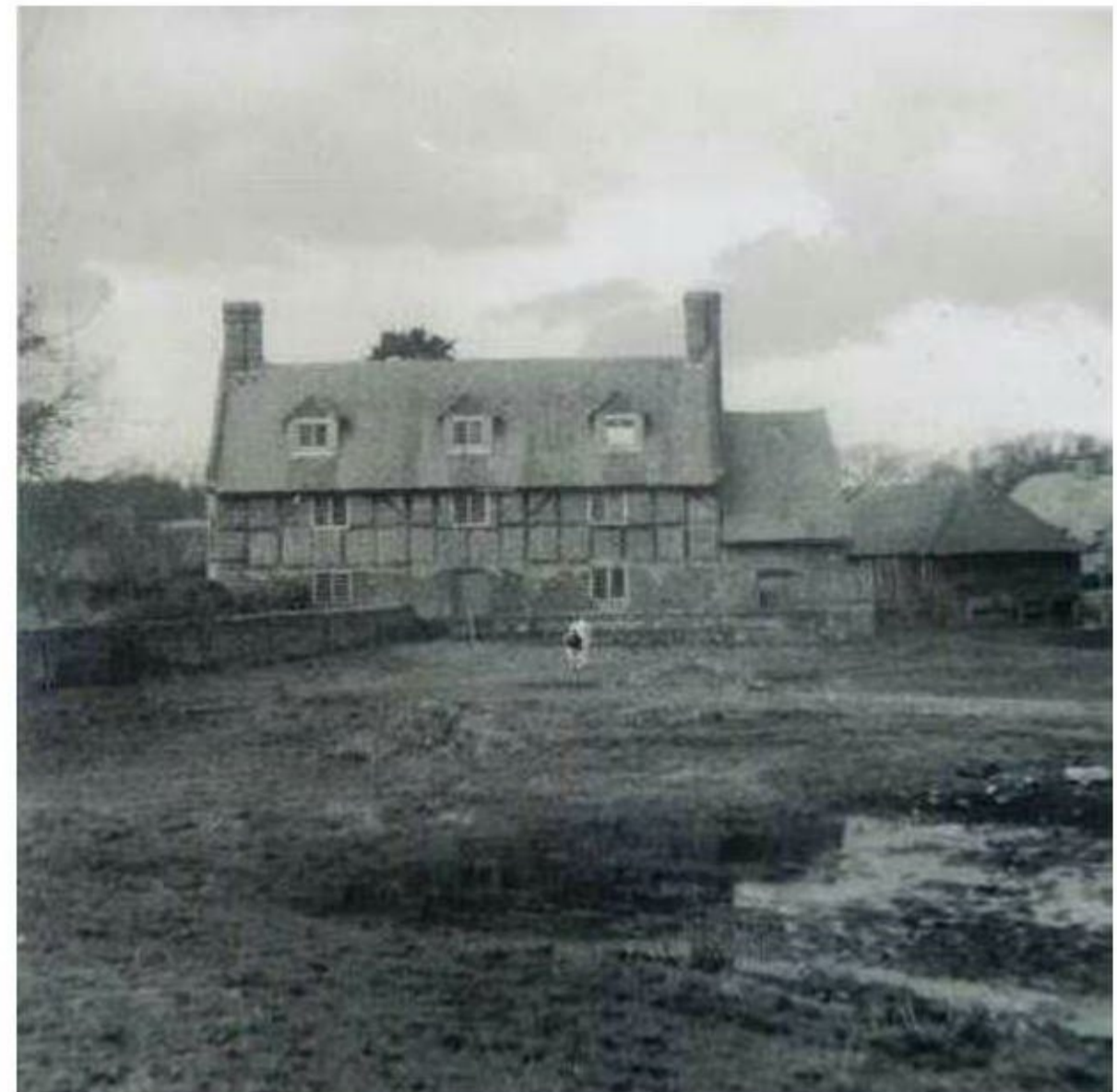
J: Rear elevation before alterations
