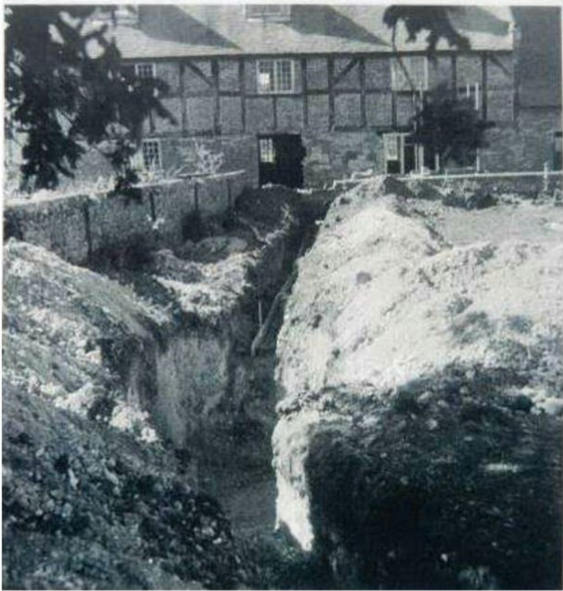
T: Rear elevation showing drainage works
