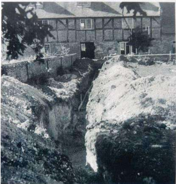
T: Rear elevation showing drainage works
