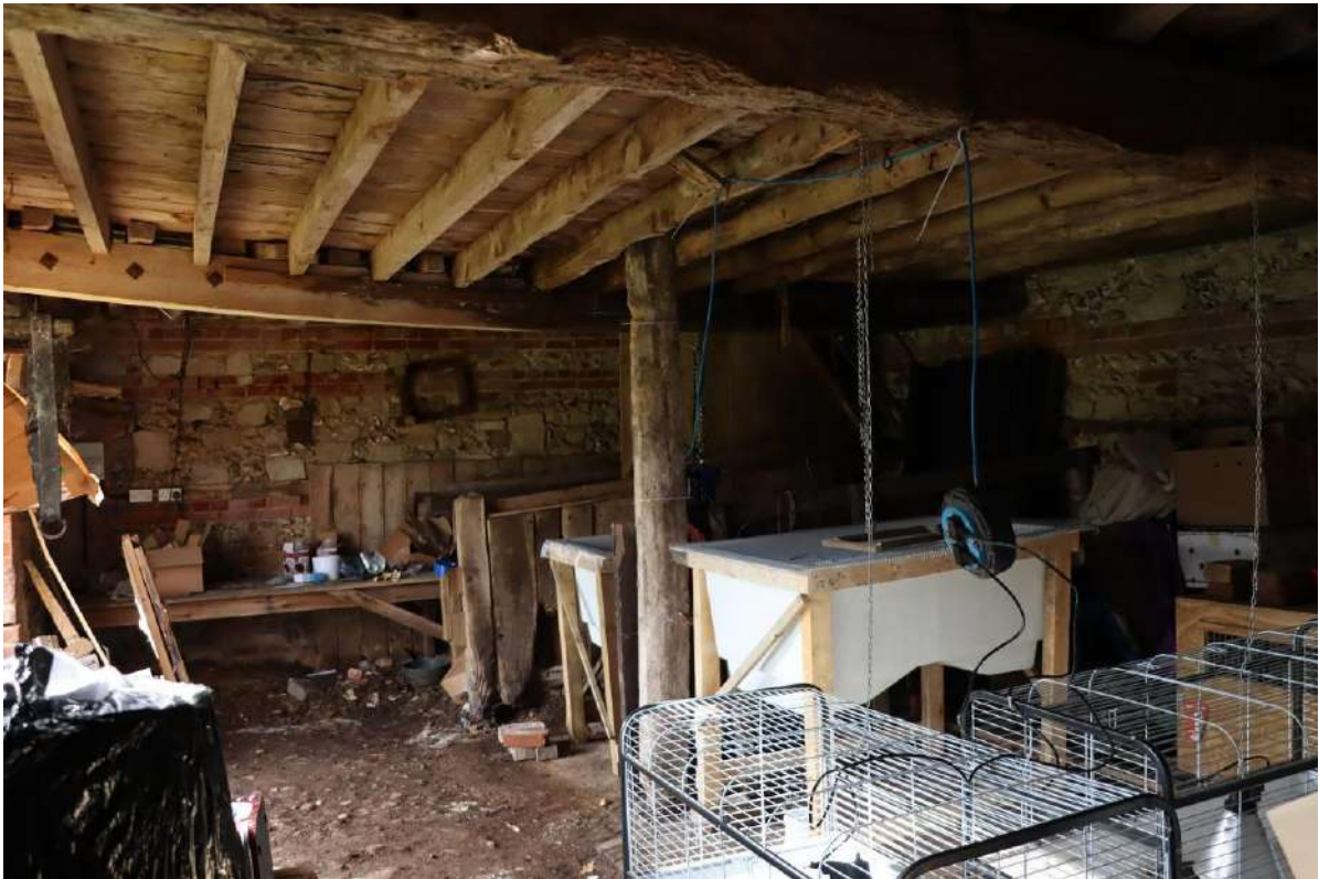
Plate 50: Building C – interior, looking W
