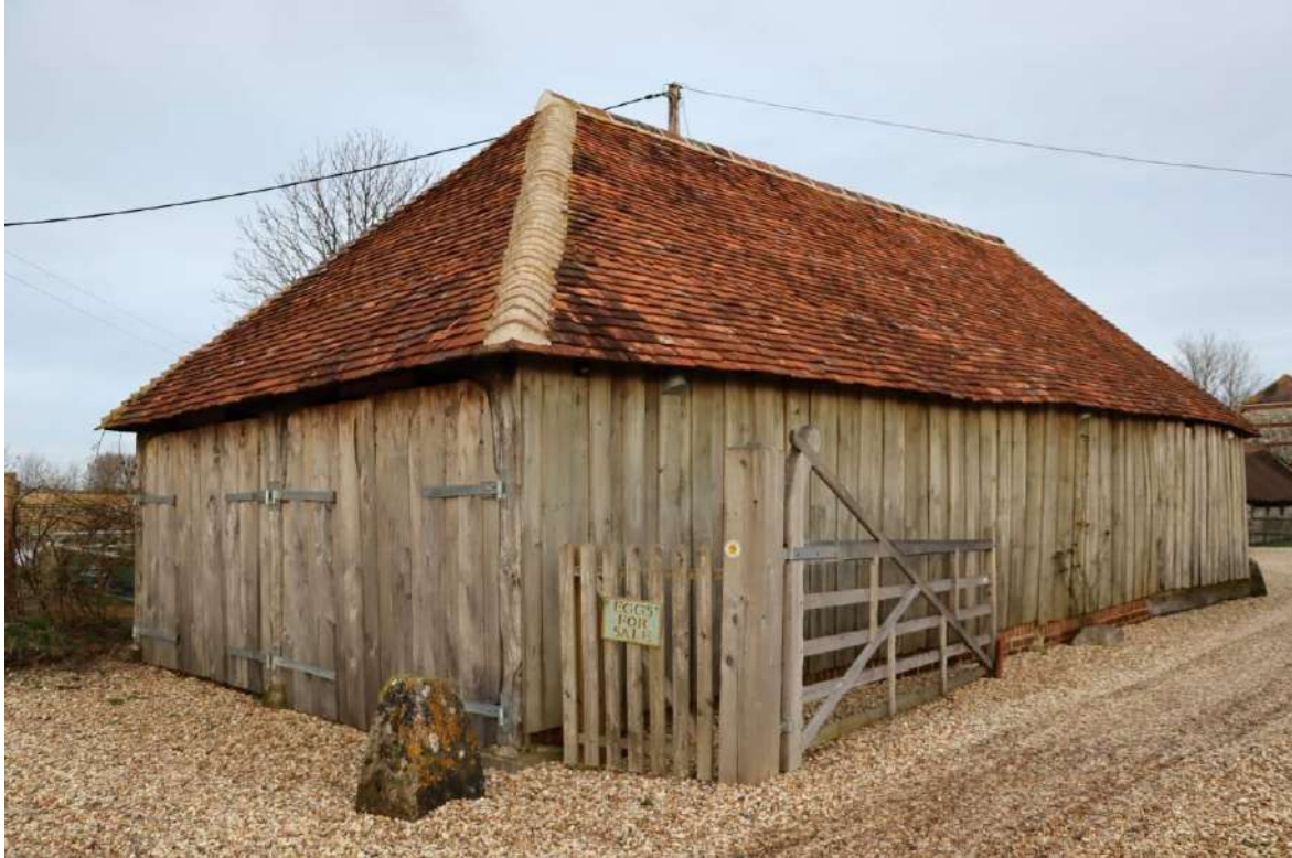
Plate 41: The Grade II listed cartshed restored in 2016 (Building A) – W end with cart entrances and long S elevation
