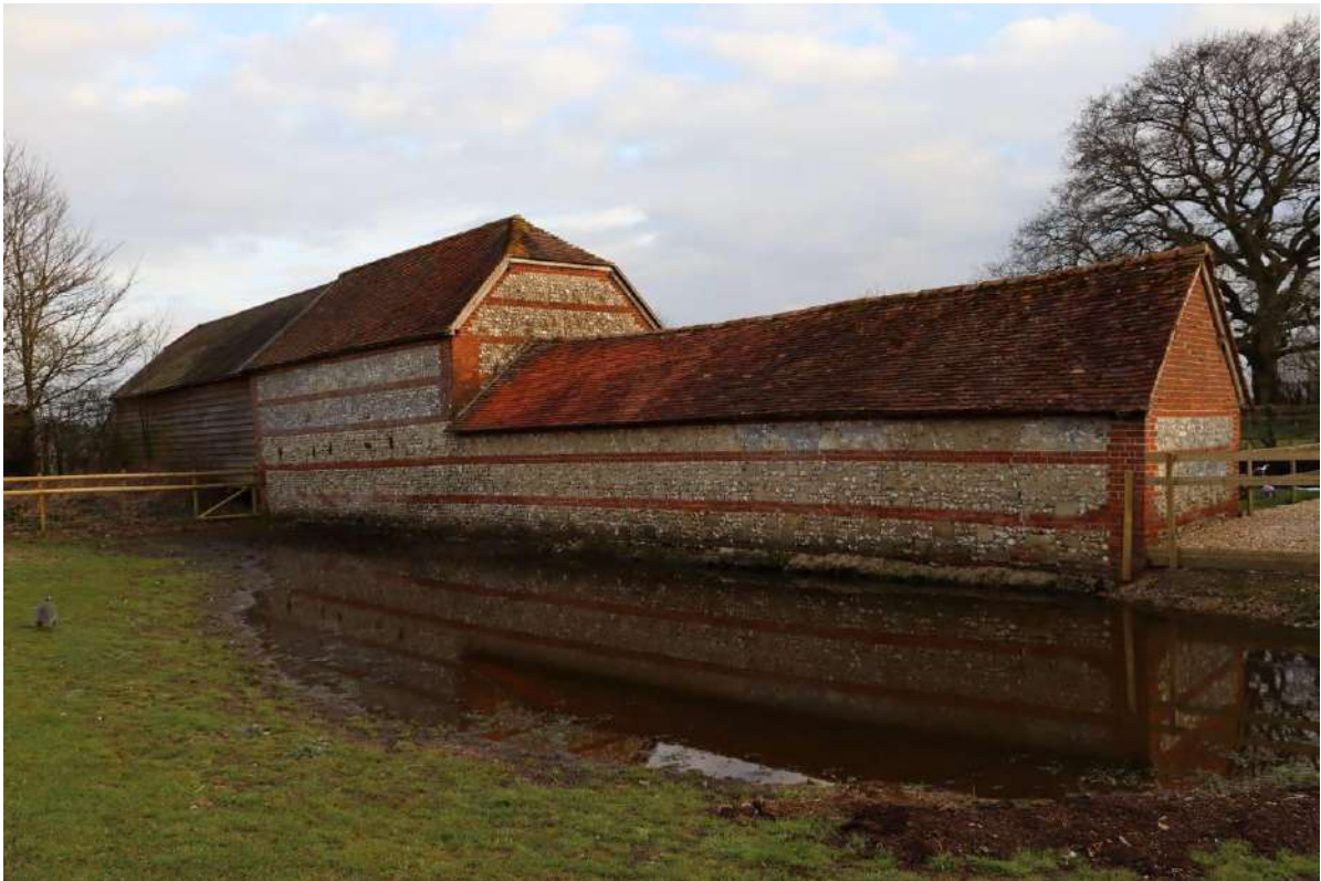
Plate 44: Buildings B, C & D (rear view)
