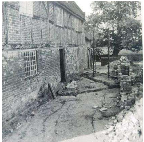
Q: Looking NE along rear elevation
