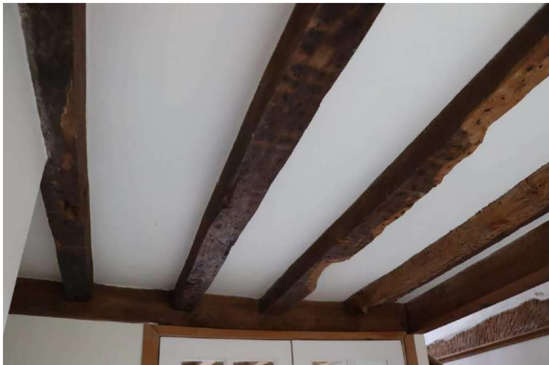
Plate 14: Surviving original joists in G2
