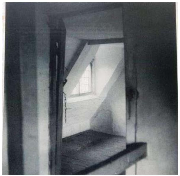
L2: Second-floor dormer
