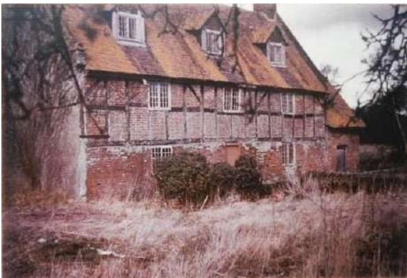
I: Rear elevation before alterations
