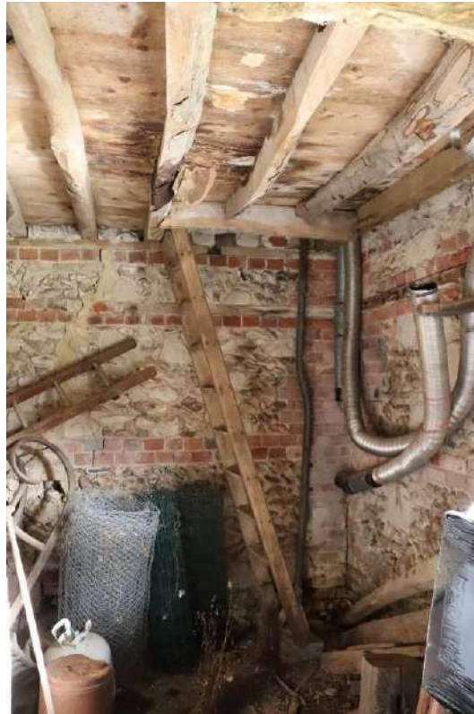
Plate 55: Building C – ladder access to hay loft
