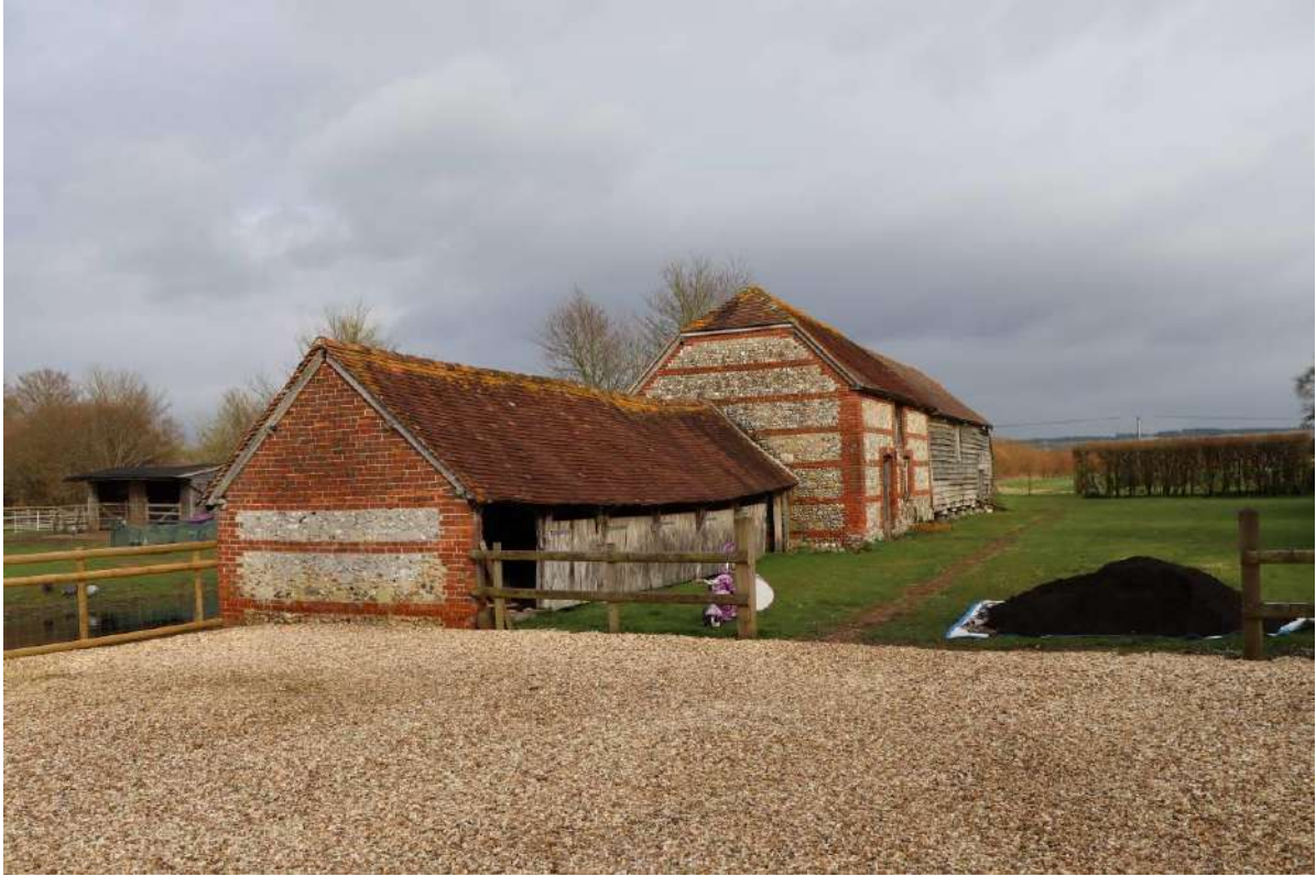
Plate 43: Buildings B (cattle shelter shed), C (stable) & D (granary), looking E
