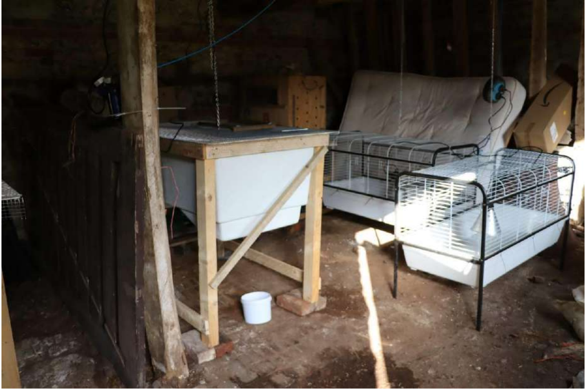
Plate 53: Building C – makeshift later stall divider to left and survival of brick flooring
