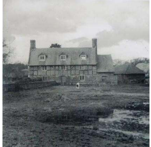
J: Rear elevation before alterations
