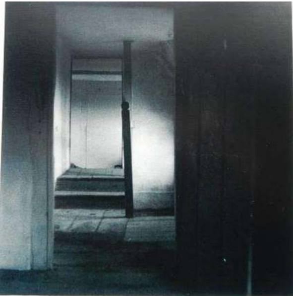
J2: S1, looking NE
