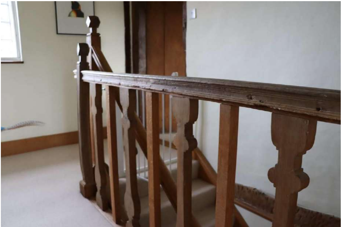
Plate 18: Original section of handrail, newel and splat balusters
