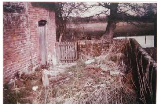
R: Looking NE past rear elevation of brewhouse
