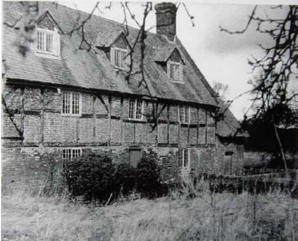
H: Rear elevation before alterations
