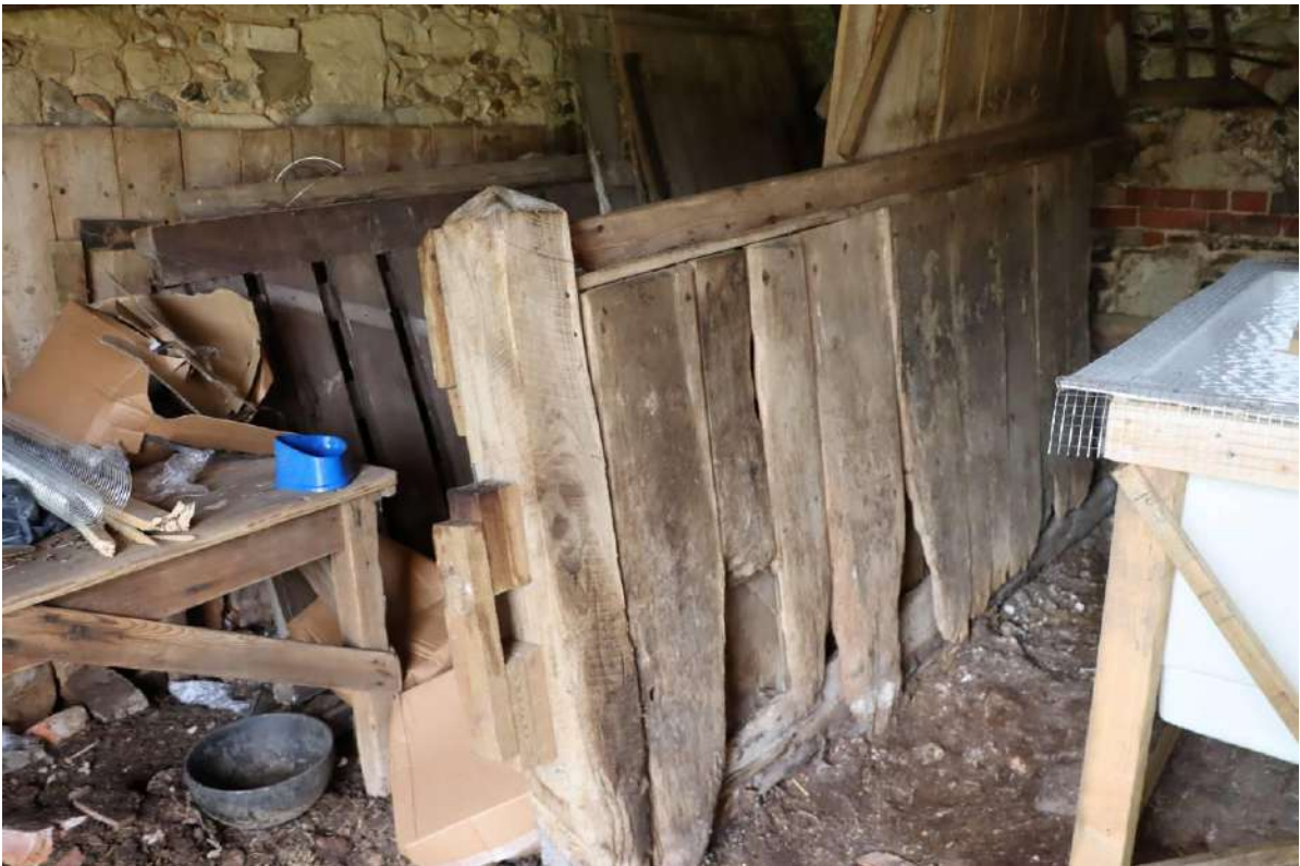
Plate 52: Building C - remnant of wooden stall divider at W end
