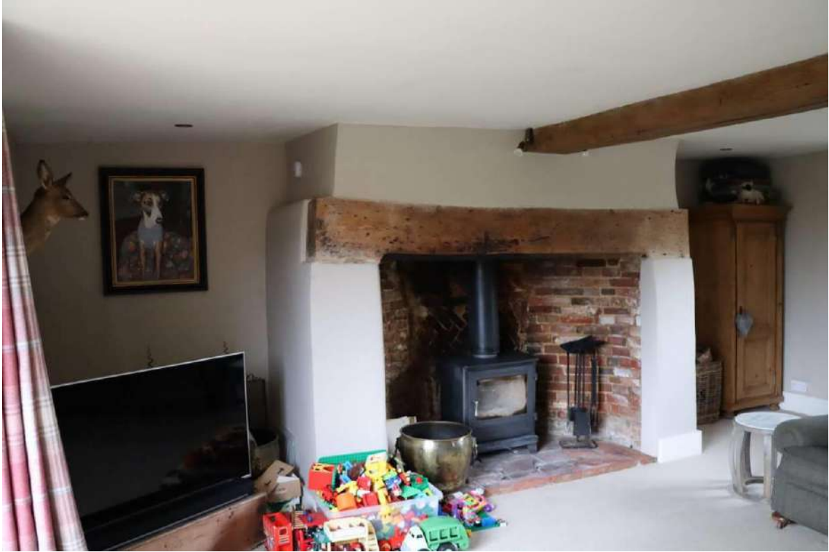
Plate 19: Reopened inglenook on SW wall of G3
