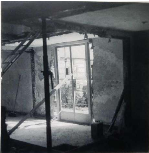
P1: Looking NE towards new rear entrance doors in G4, from G3
