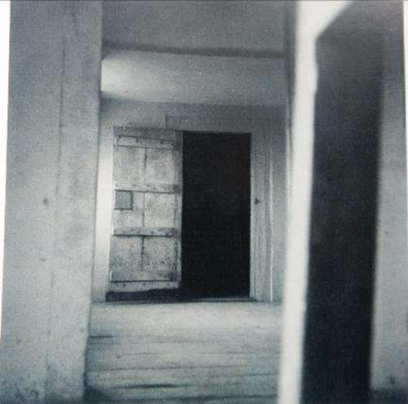
M2: Attic room
