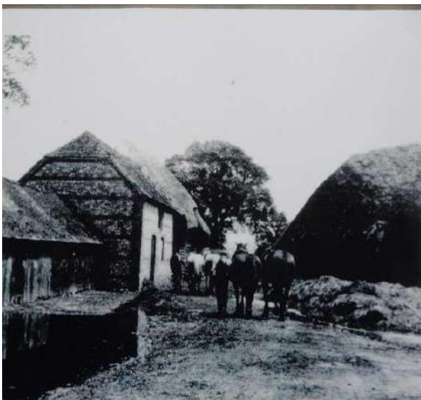
B: Undated, late C19/early C20: Buildings B-D and demolished thatched barn to right
