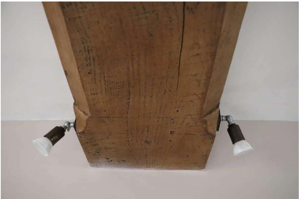
Plate 20: Chamfer stops to beam in G3
