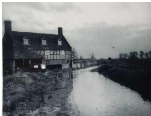
D: Looking S along a flooded Flood Street towards the farmhouse
