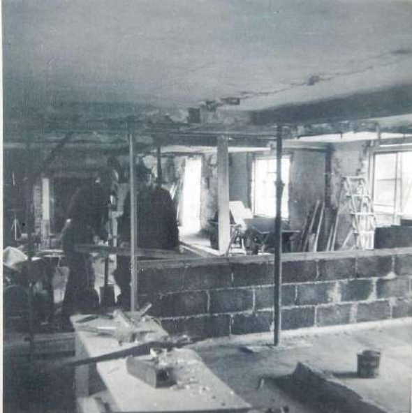
O1: Looking NE from G3 across central bay into G4: new concrete blockwork wall being built to divide G3 from central bay
