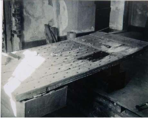
W1: Old double-thickness door, removed and apparently not retained in the farmhouse
