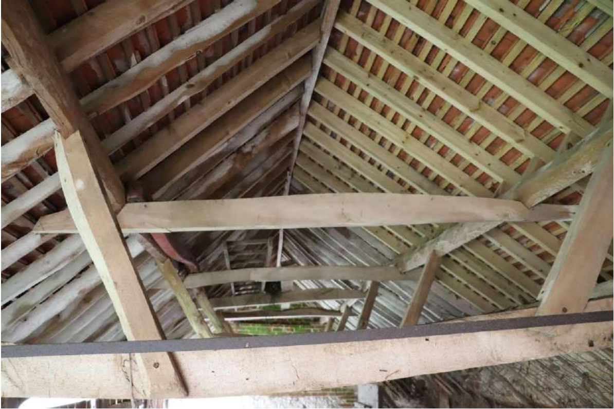
Plate 47: Building B – detail of roof structure
