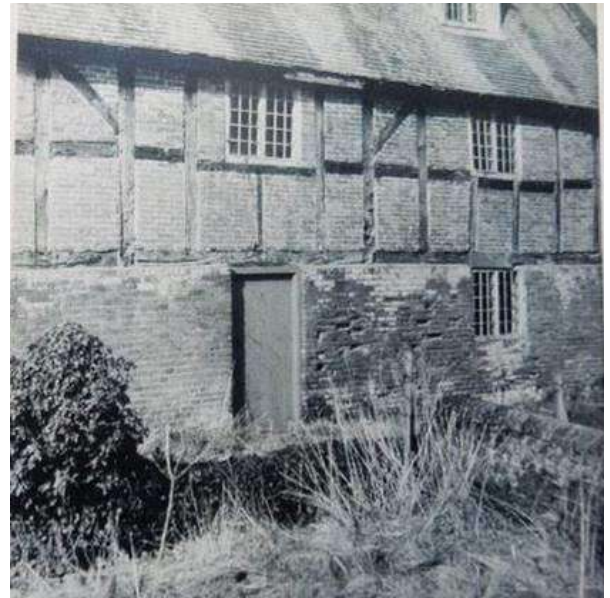
K: Rear elevation before alterations
