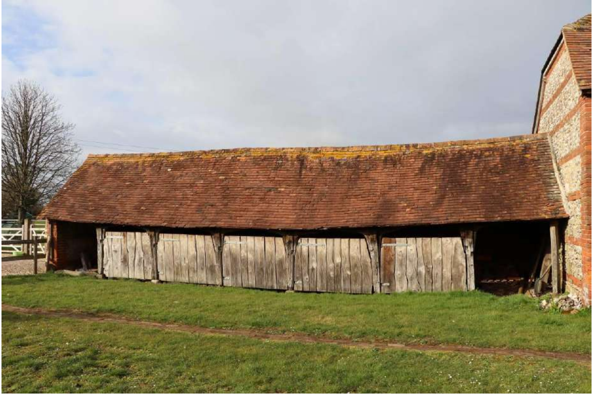
Plate 45: Building B – former cattle shelter shed
