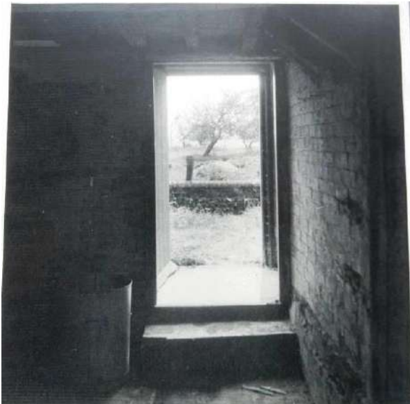
Z: Looking SE past old staircase enclosure (right) through internal doorway onto rear passage and rear entrance (viewpoint now the part of G4 in central bay)
