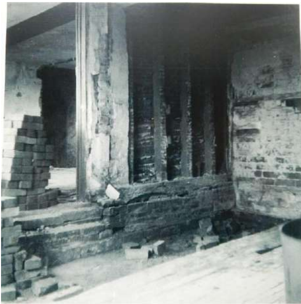
E1: Similar viewpoint as above, further to the right: looking towards remains of timber-framed wall. The brick wall to right was to be removed.
