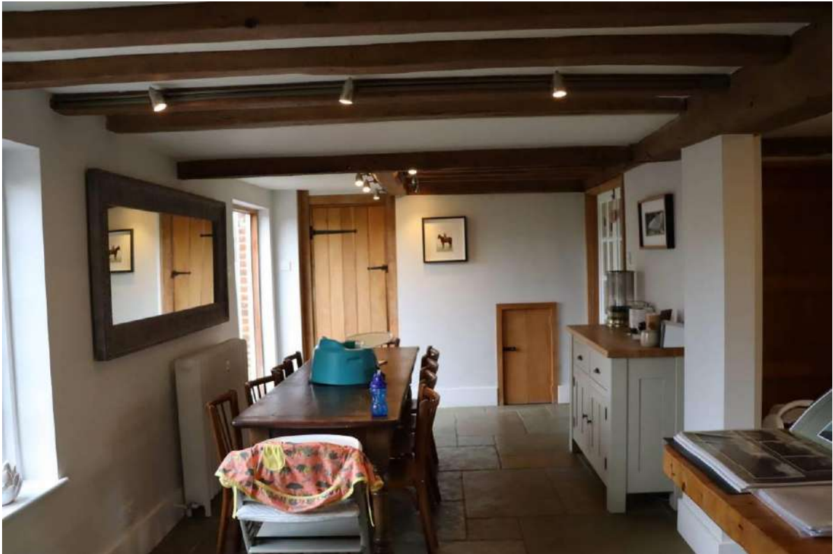
Plate 21: G4, looking SW into area within central bay, formerly divided from G4 by a timber-framed wall
