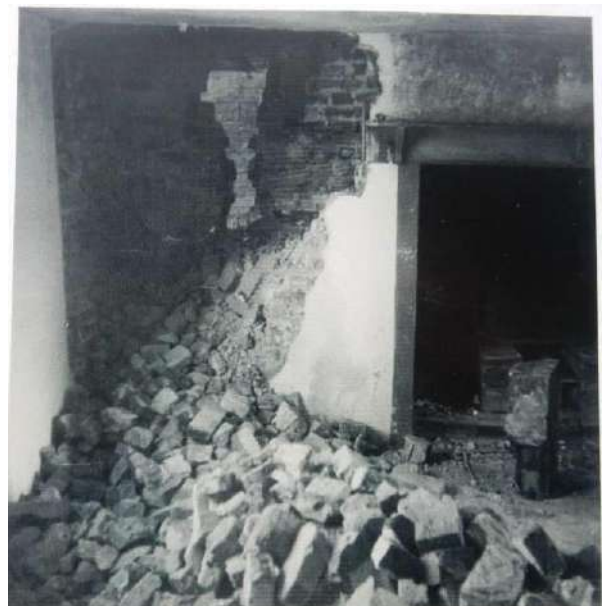
R1: Demolition of wall and bread oven left of G4's fireplace
