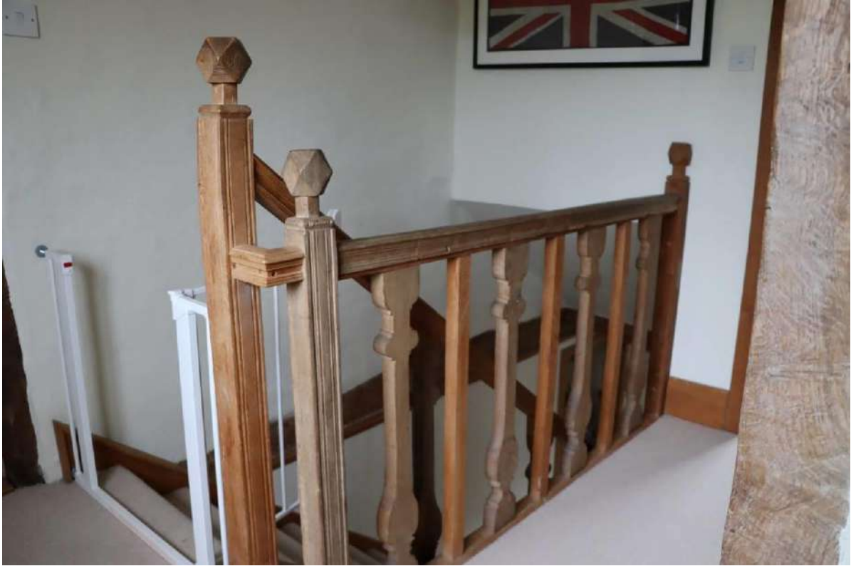
Plate 17: F1 (first-floor landing): note original newel and taller replica, original section of handrail and splat balusters
