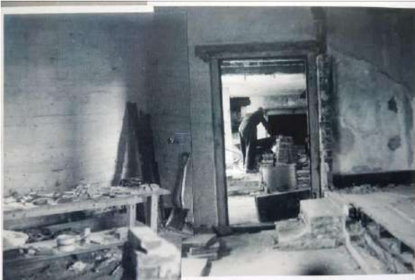
J1: Looking NE from G3 through doorway into central bay and beyond into G4: to the right a wall stood on the alignment of the higher floor level, said to be C19 and dividing the NW part of G3 (dairy) from the SE part (parlour)
