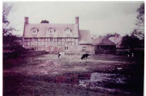
L: Rear elevation before alterations
