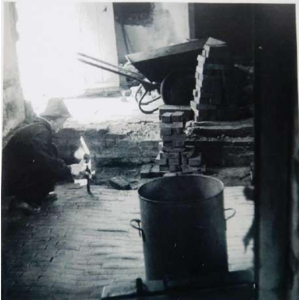
D1: Looking NE from G2; the bricks are on the line of a removed internal wall. The lower brick floor is being dug out
