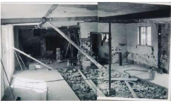
K1: Looking SW from G4 across central bay into G3. A partly demolished brick wall divides central bay from G3. The old staircase (removed) ascended from L to R where the rest of the brick wall has been demolished
