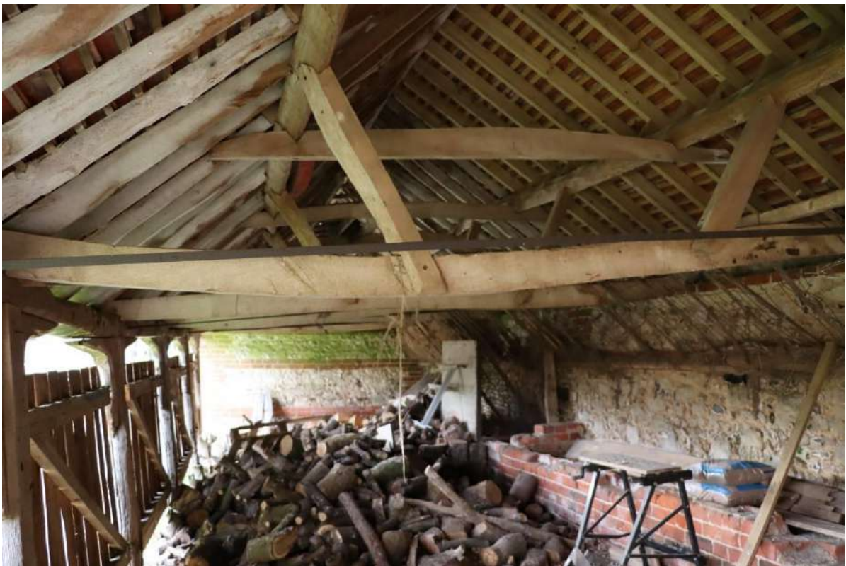
Plate 46: Interior of Building B, looking W
