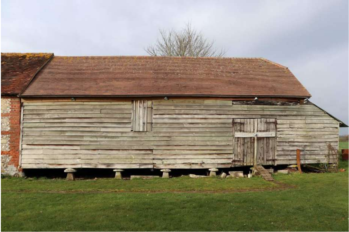
Plate 57: Building D - granary
