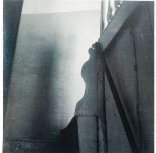
Y1: Detail of carved wooden piece where the staircase turns through 90 degrees up to the first floor (this was not retained)
