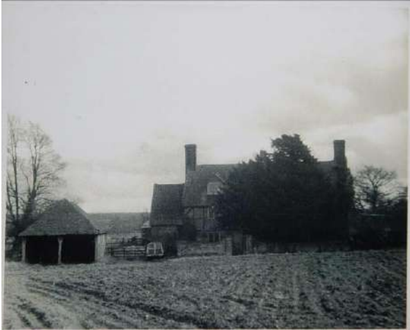
G: Front elevation, largely obscured by tree, and Building A (cart-shed)
