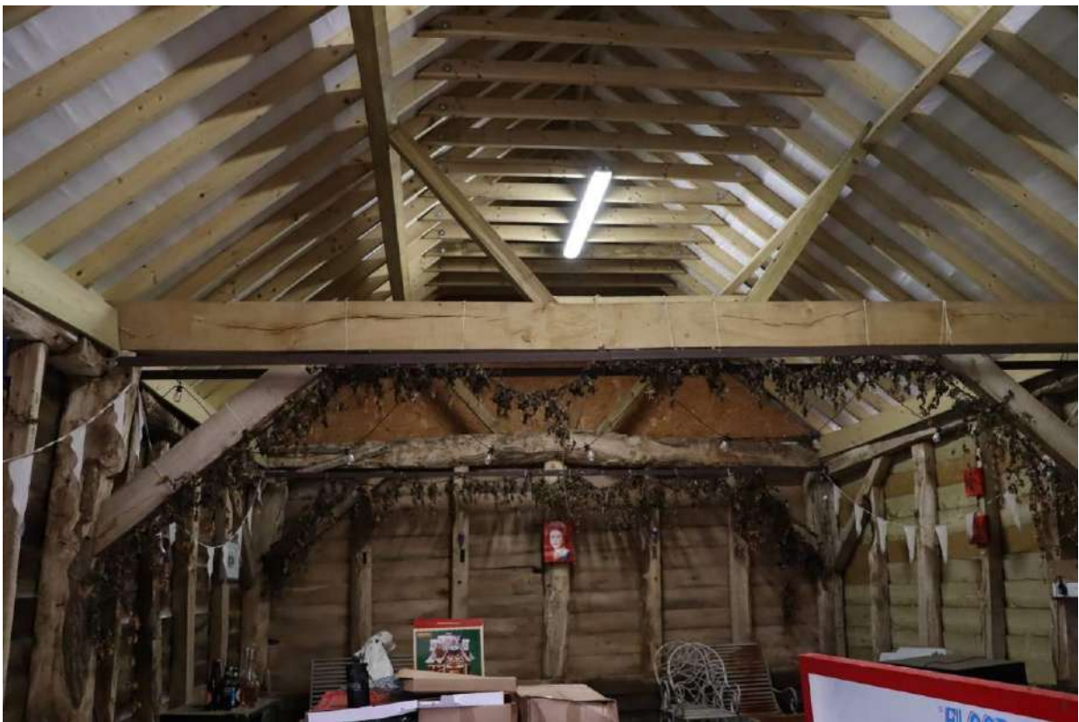
Plate 58: Building D: interior, looking W
