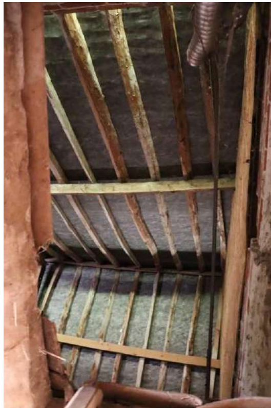
Plate 56: Building C – view into hay loft and roof structure
