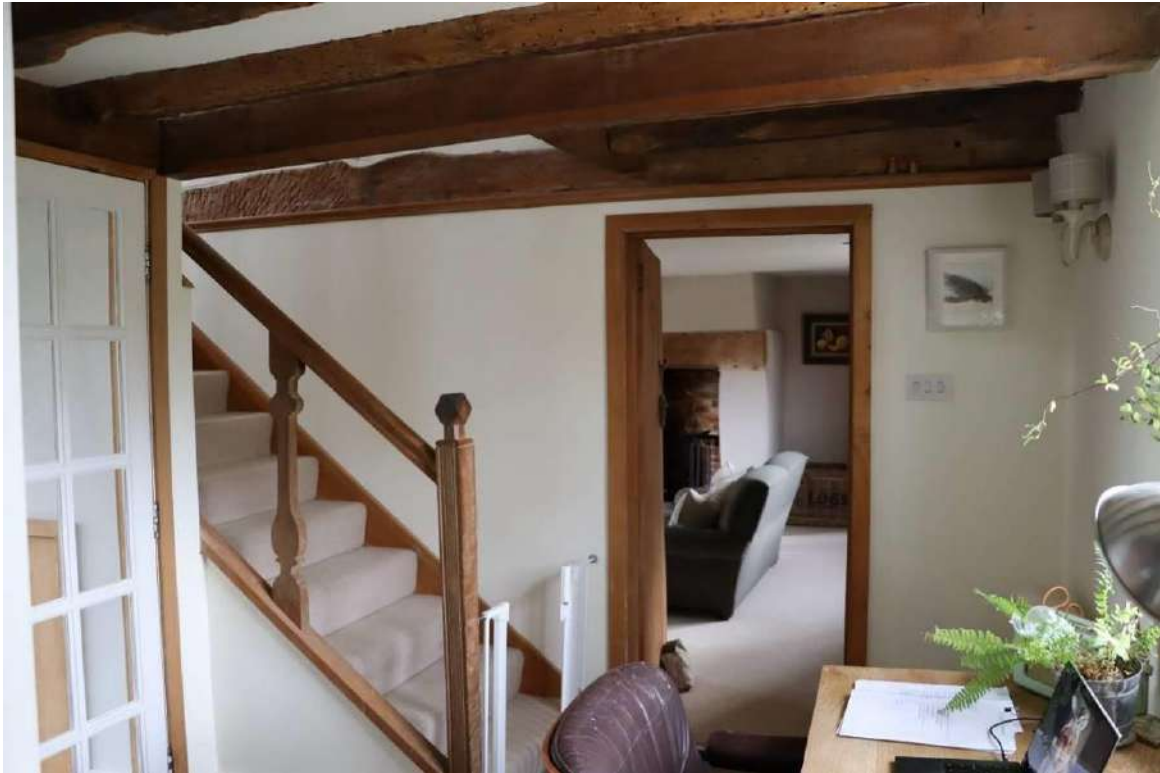
Plate 15: G2, looking towards 1950s' staircase (the newel may be original) and concrete blockwork dividing wall with G3
