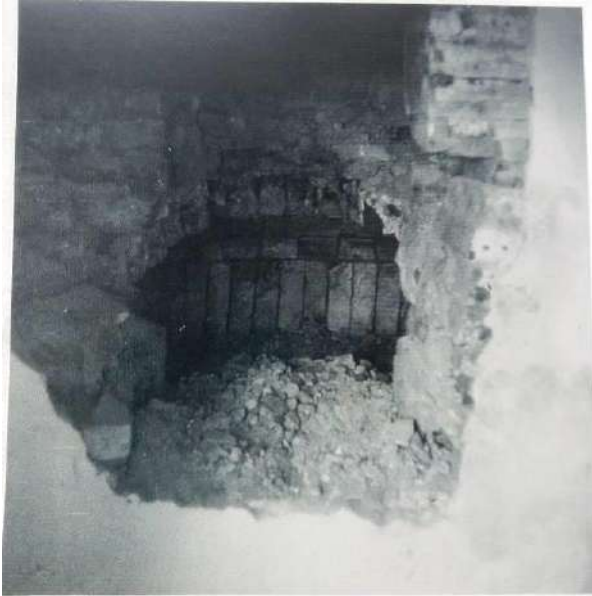
S1: Looking into bread oven before demolition
