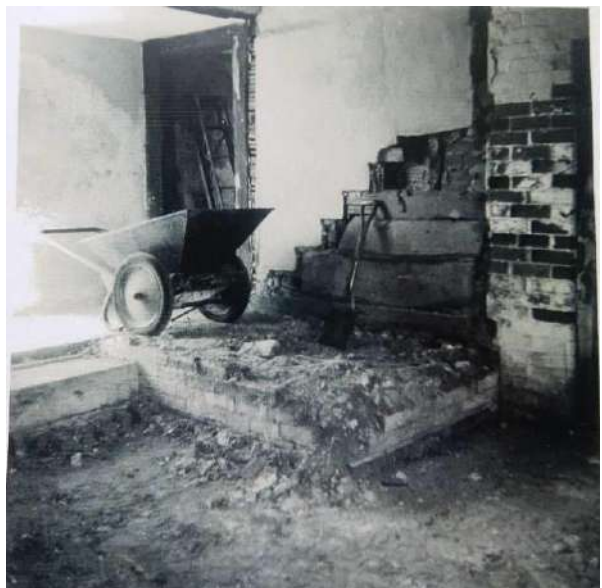
C1: Similar viewpoint to above following further demolition of staircase
