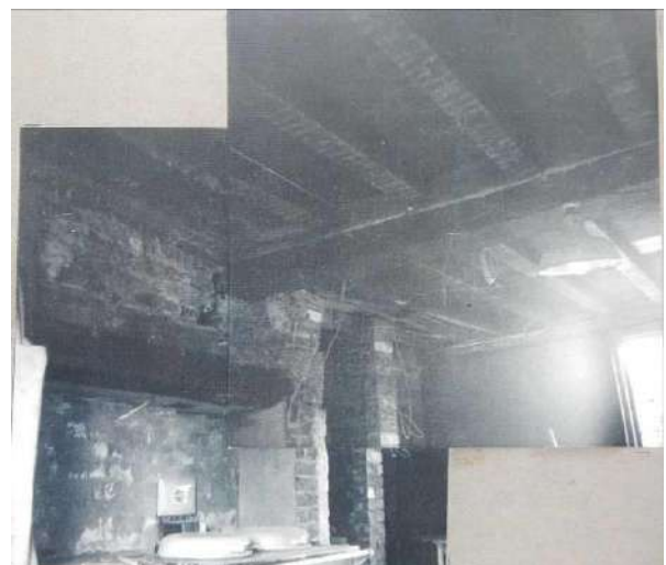
N1: G4, fireplace with newly installed Aga to left
