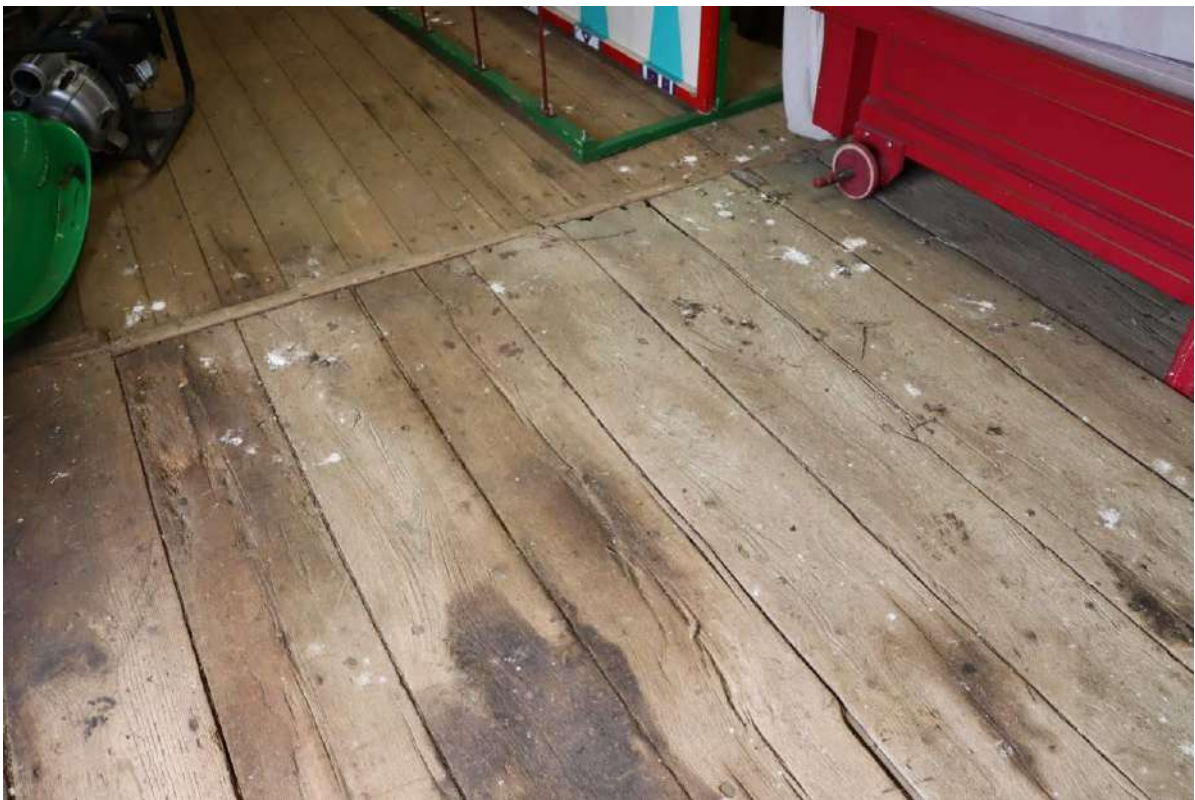
Plate 60: Building D: floorboards (wider earlier ones in foreground)
