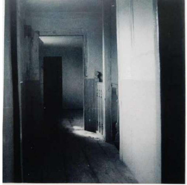
C2: F1, looking SW
