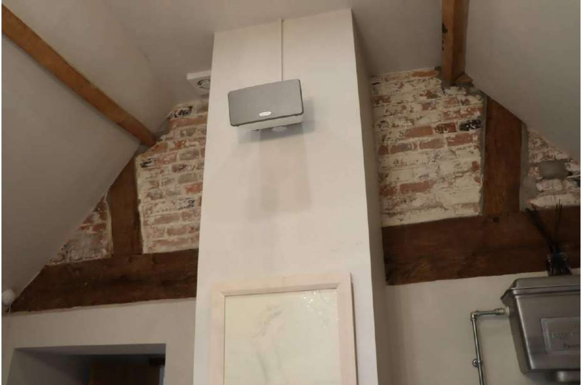
Plate 33: F4: chimneybreast and exposed truss struts in NE gable end of main range
