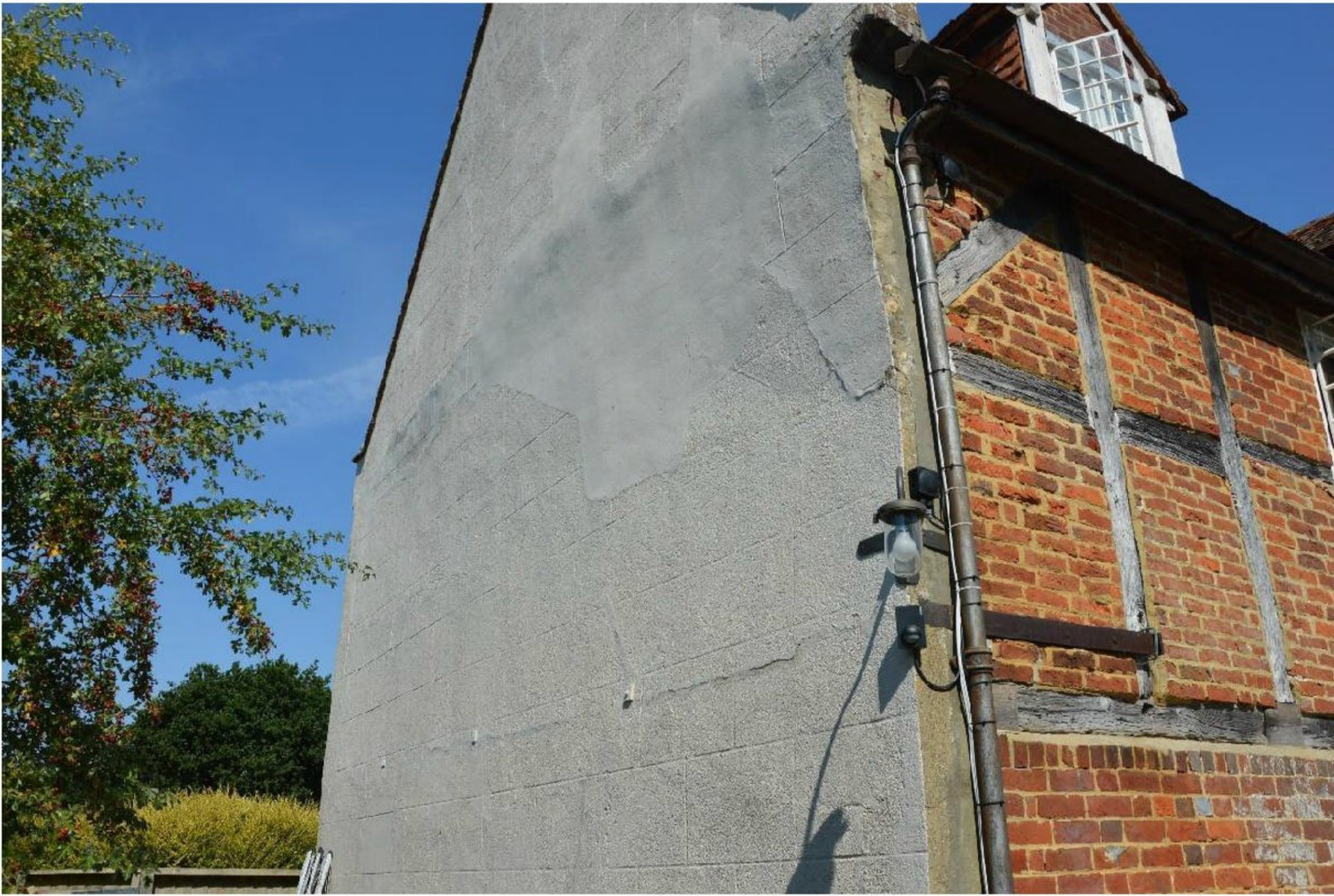
Plate 1. South gable where linking structure will join the main house.
