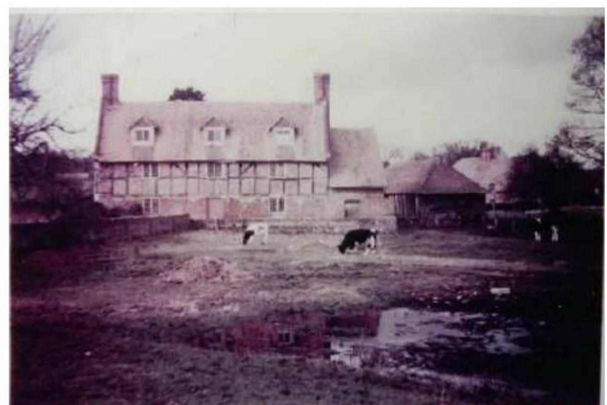
L: Rear elevation before alterations
