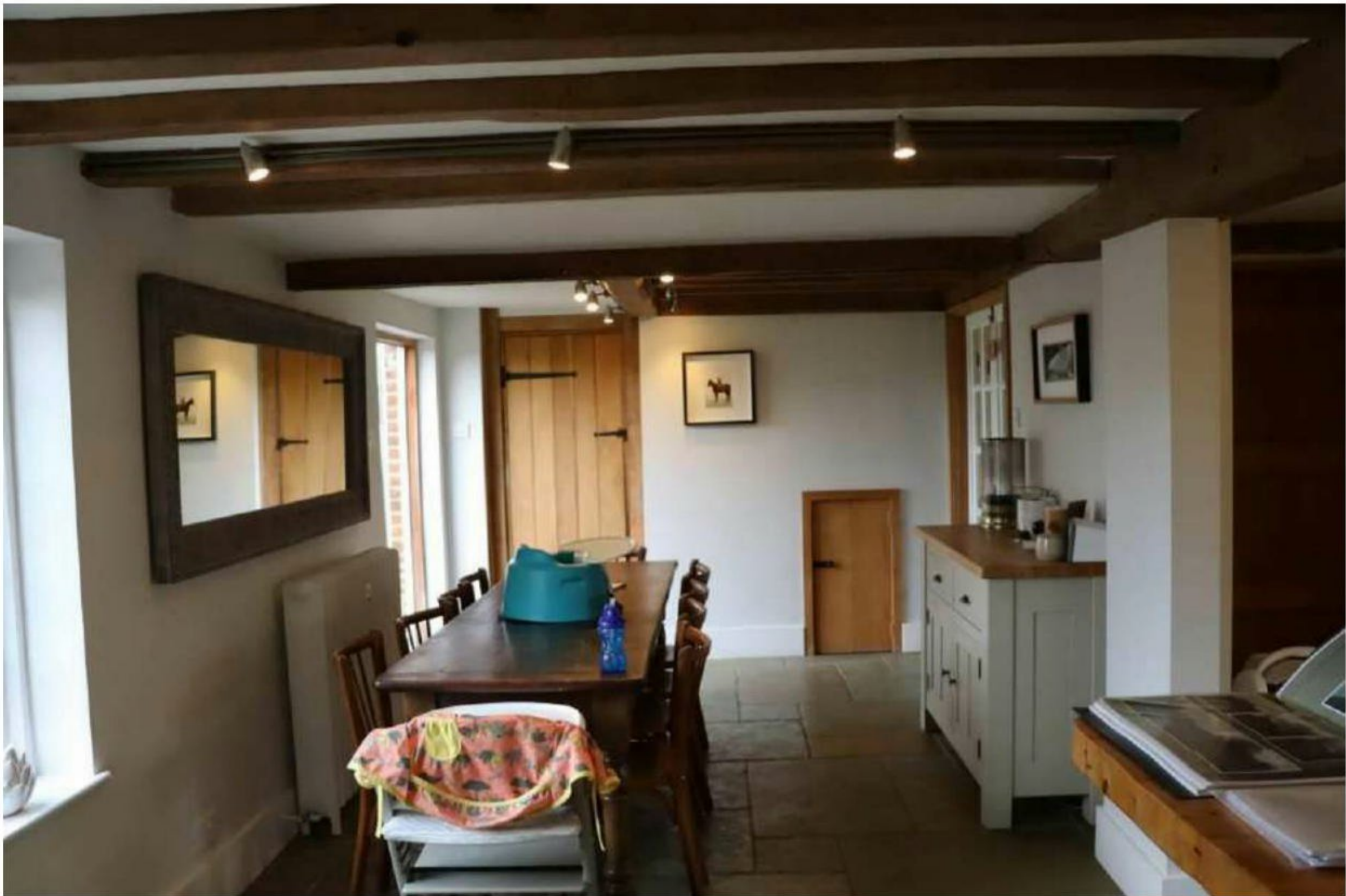
Plate 21: G4, looking SW into area within central bay, formerly divided from G4 by a timber-framed wall
