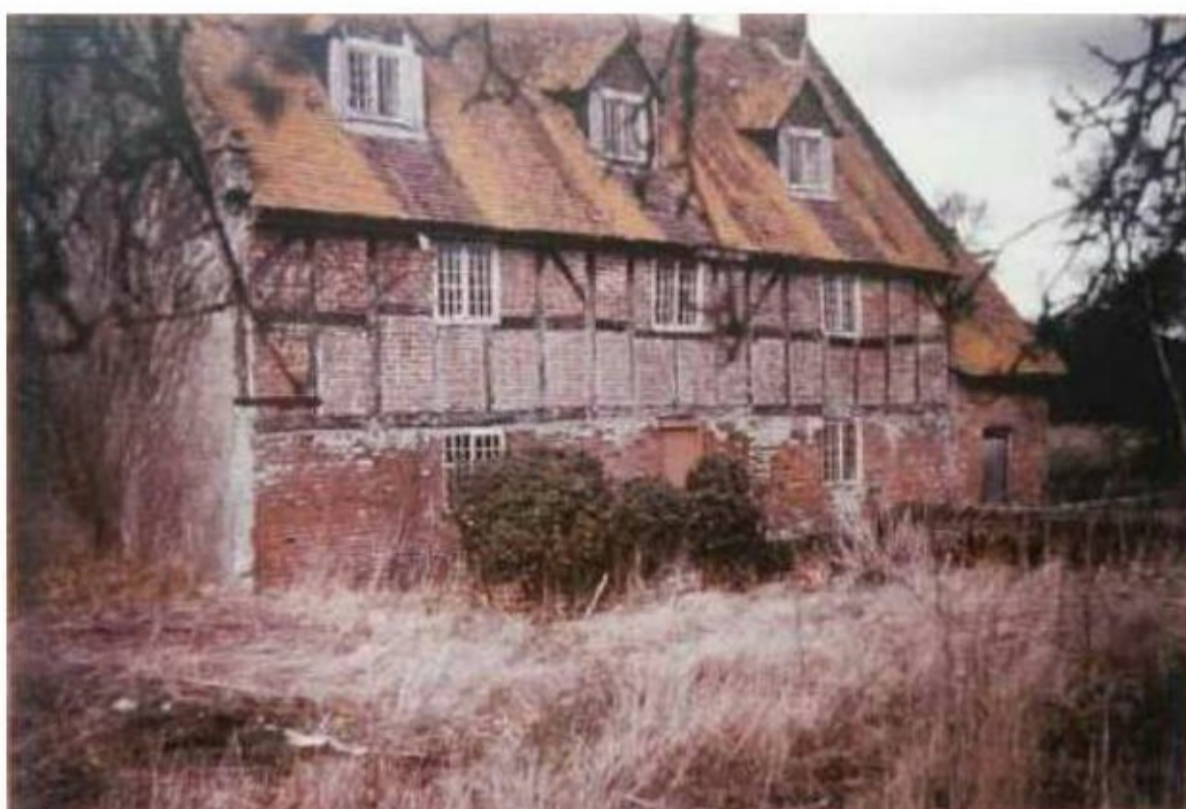
I: Rear elevation before alterations
