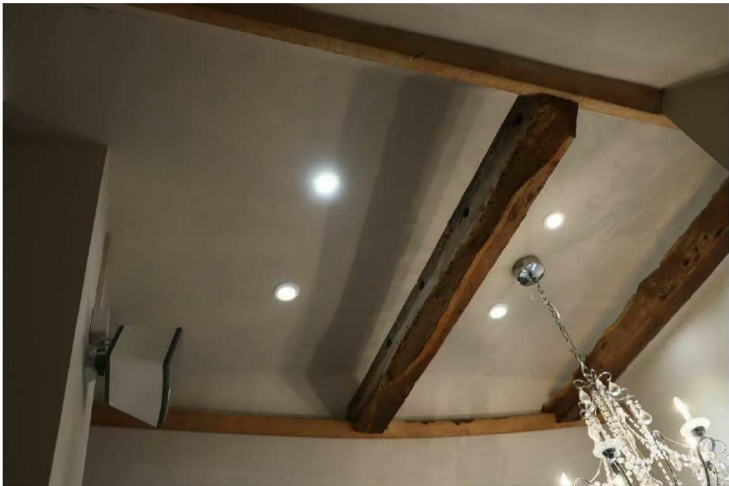
Plate 32: Exposed roof timbers in F4
