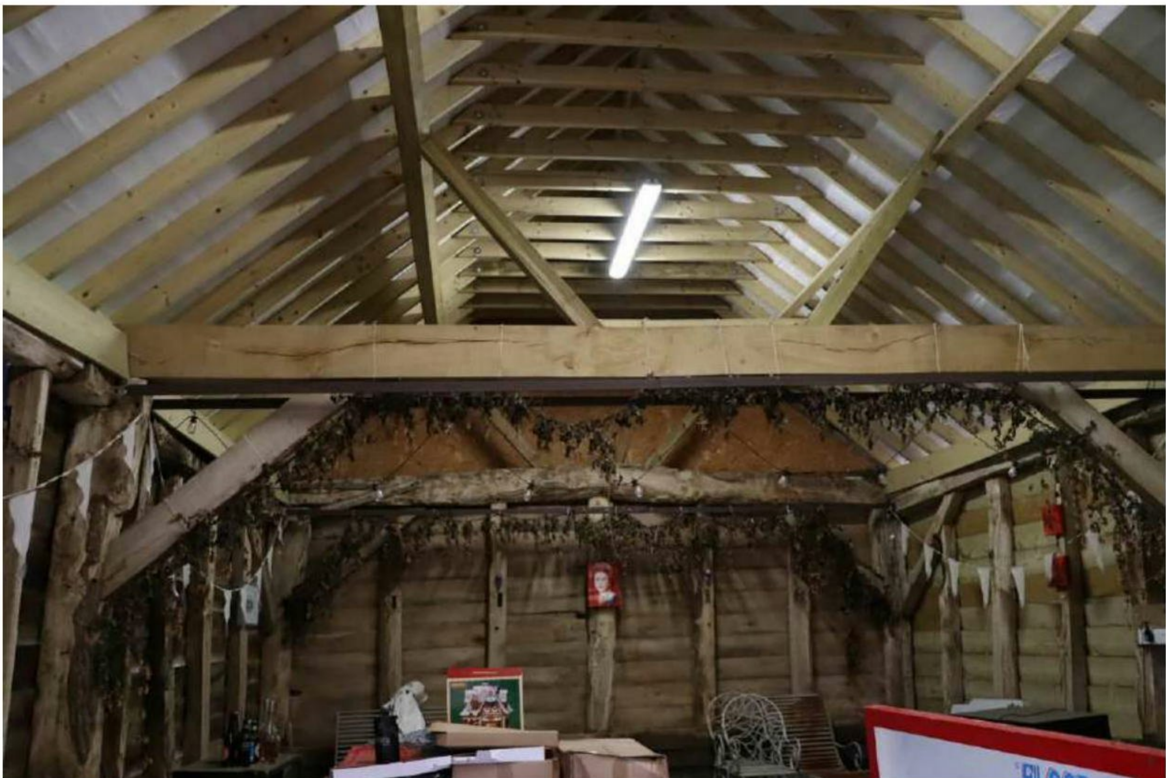
Plate 58: Building D: interior, looking W
