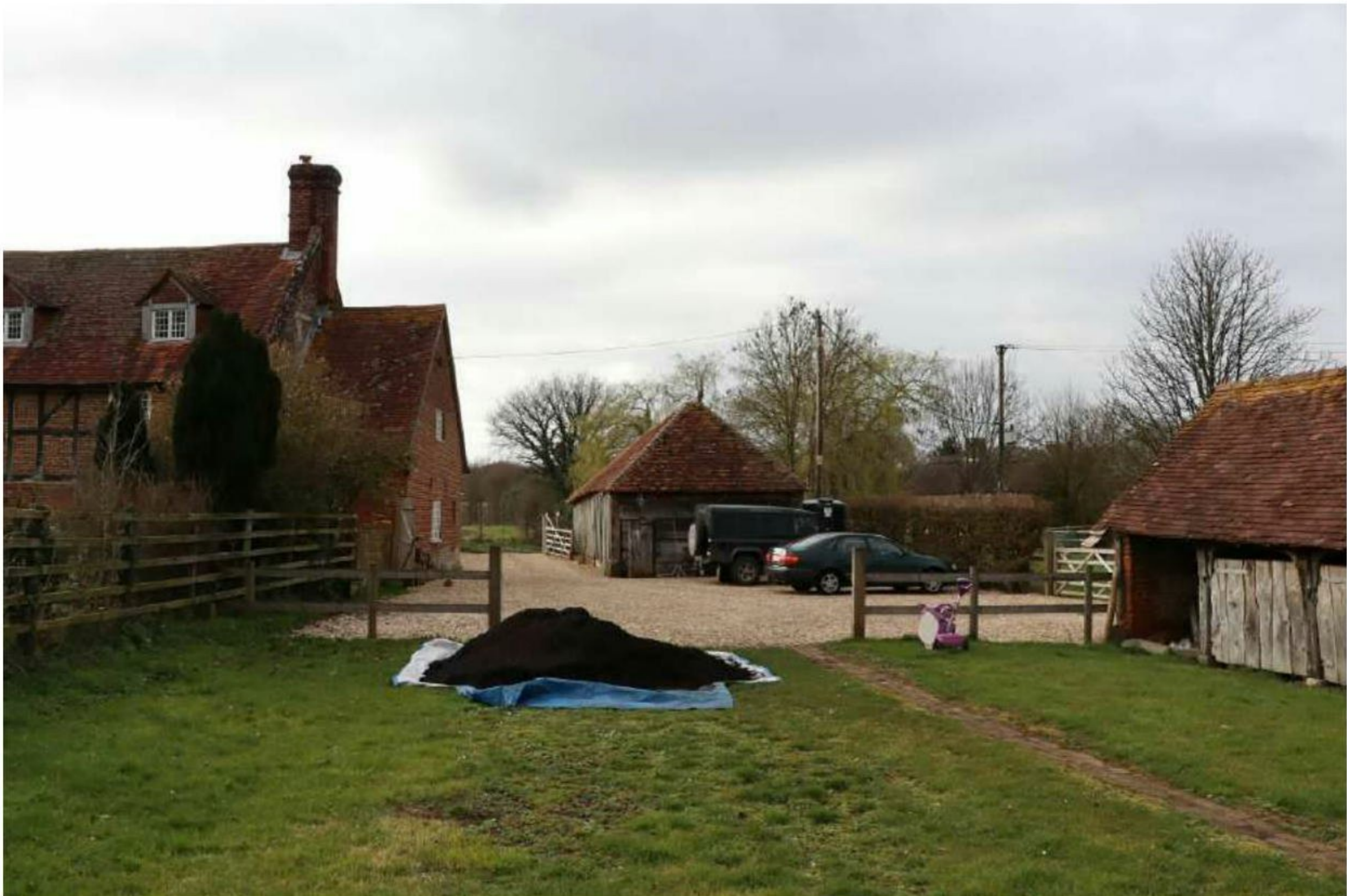
Plate 62: Looking W past Buildings B-D (right) along the historic farm access
