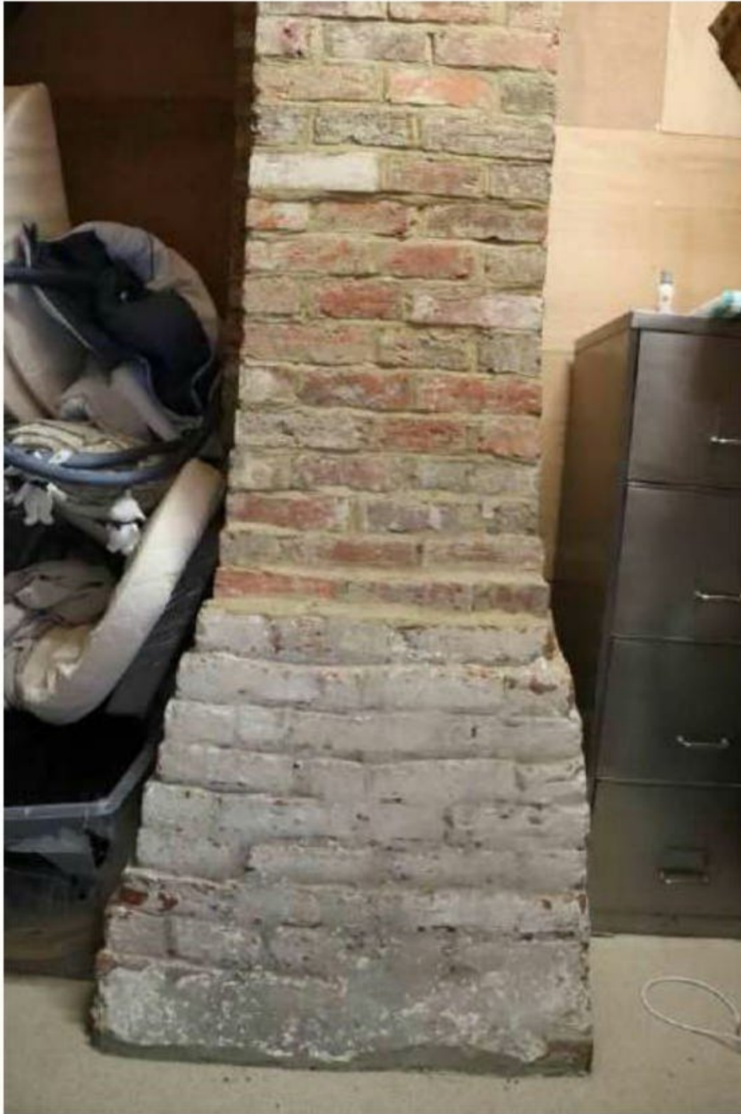
Plate 39: Chimneystack on SW wall of S4; note the rebuilt section above the white brick
