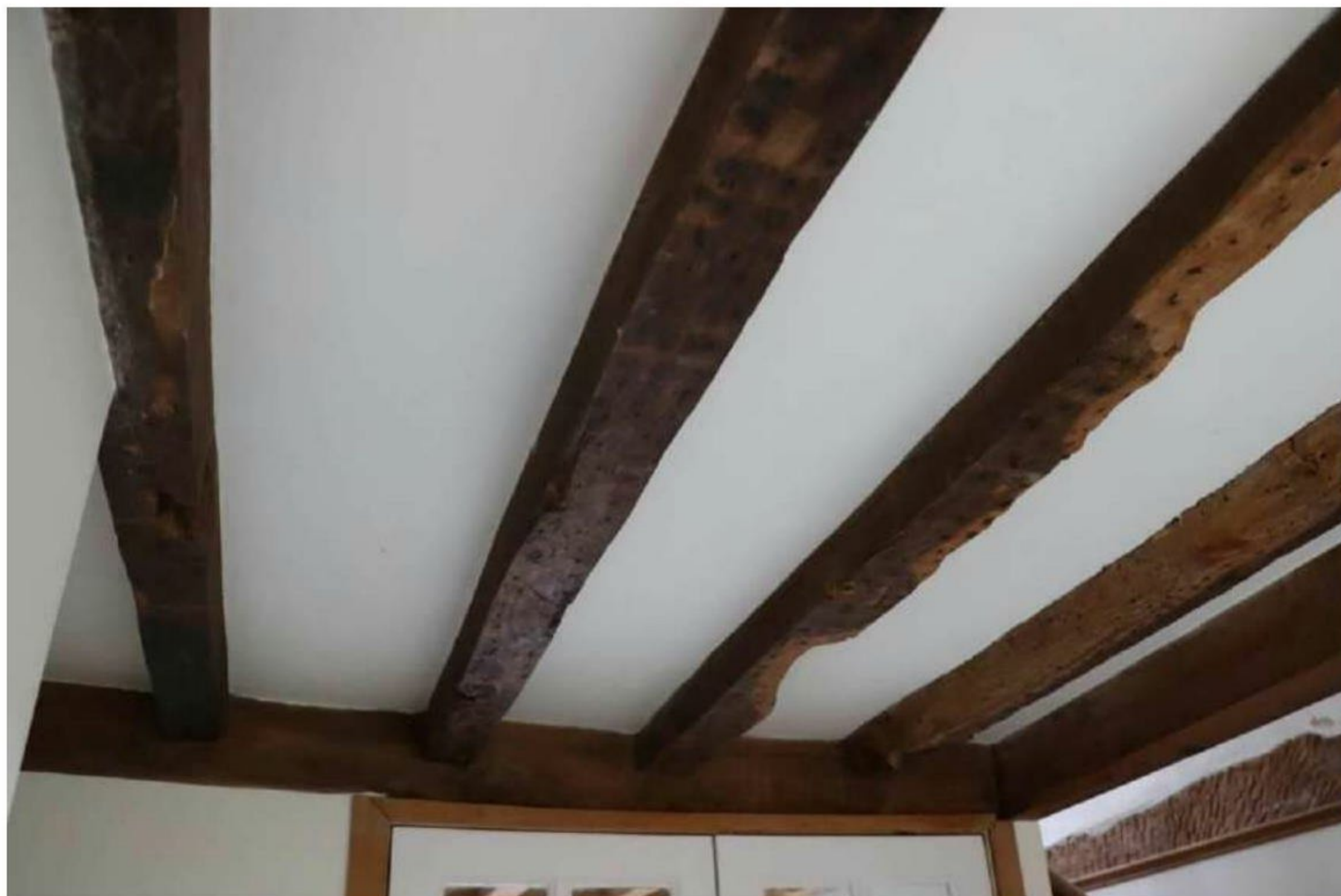
Plate 14: Surviving original joists in G2
