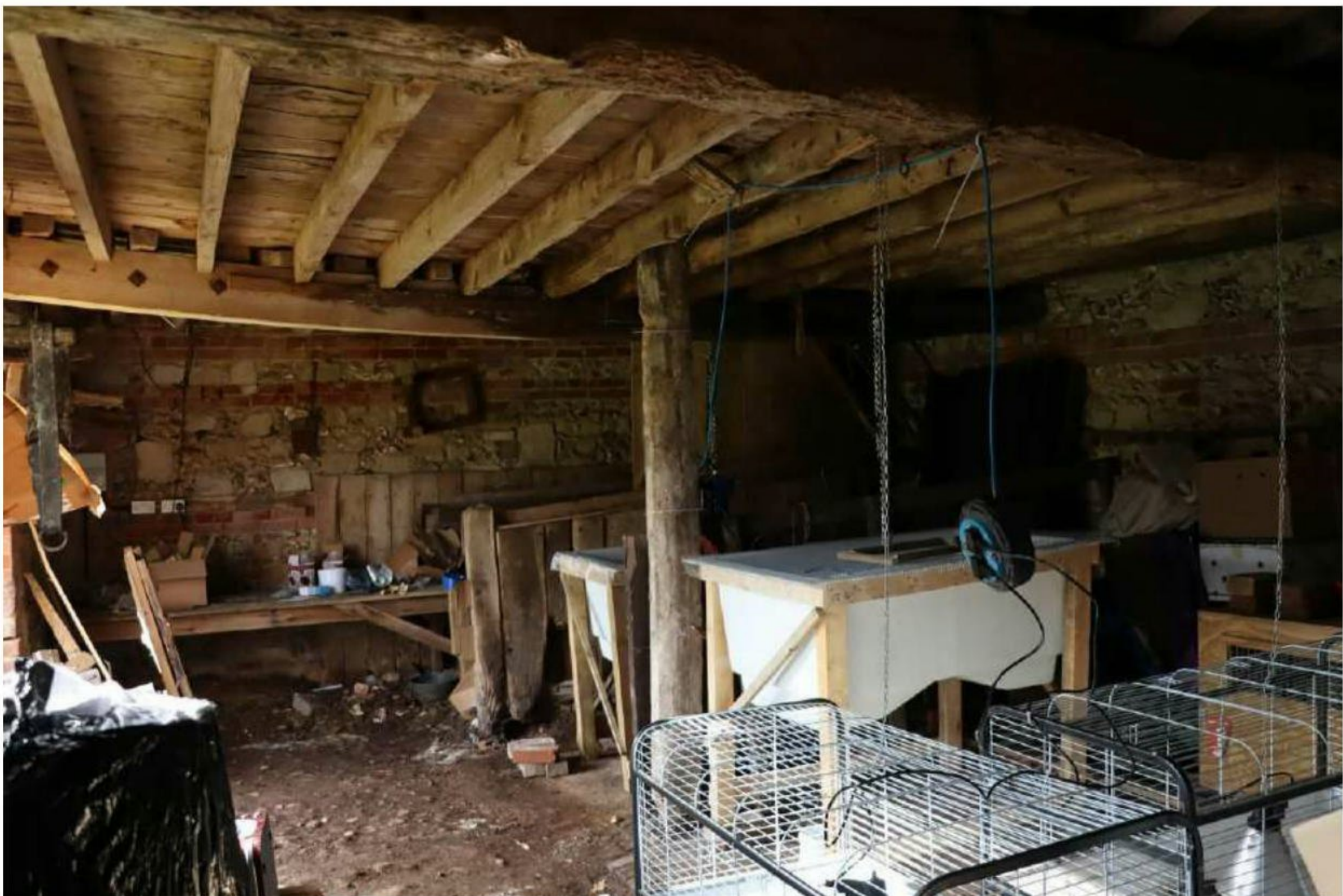
Plate 50: Building C – interior, looking W
