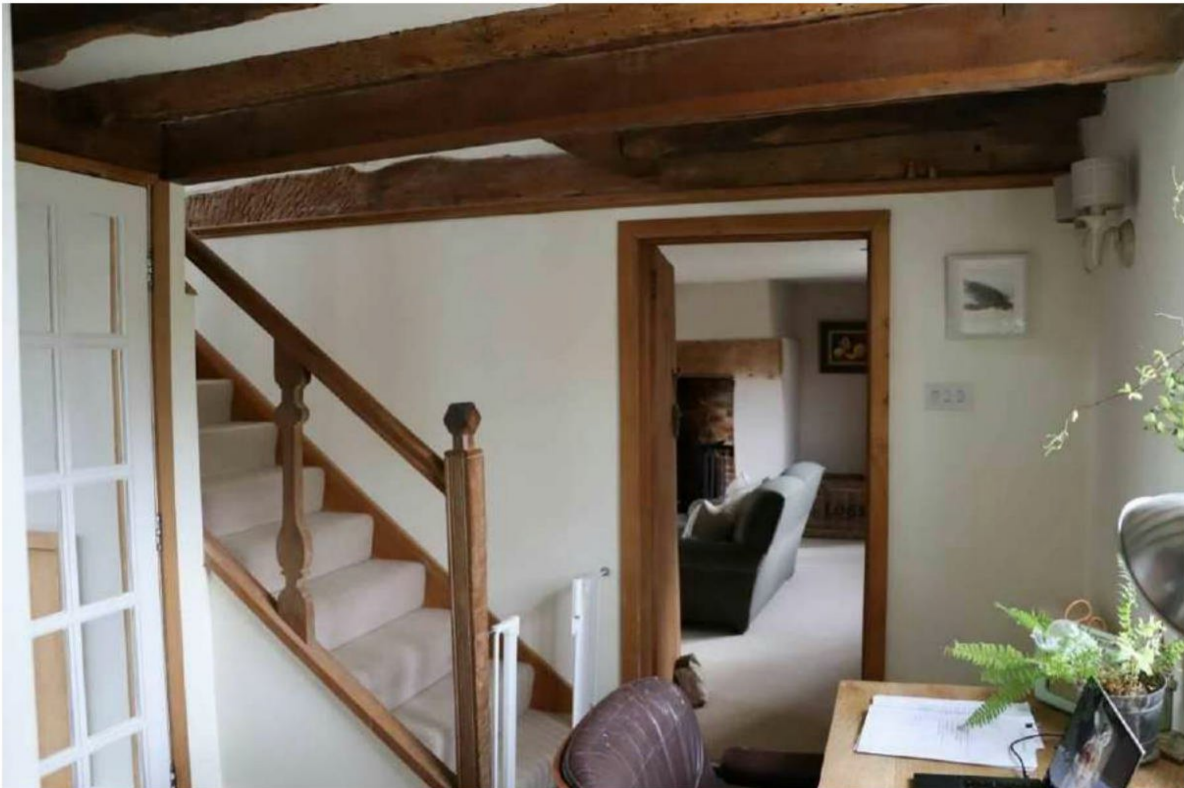
Plate 15: G2, looking towards 1950s' staircase (the newel may be original) and concrete blockwork dividing wall with G3
