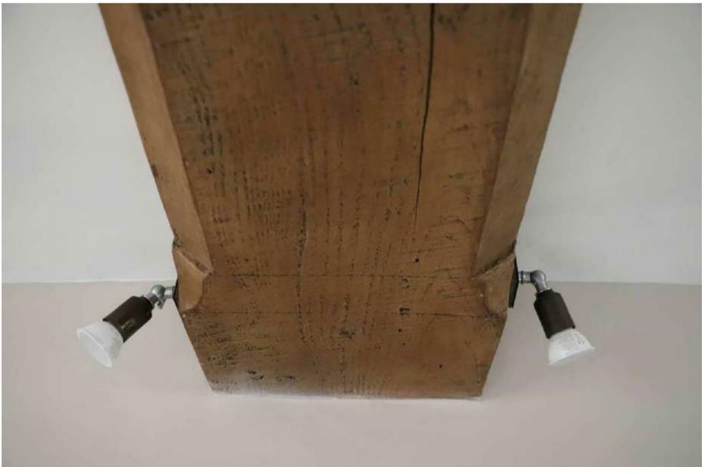
Plate 20: Chamfer stops to beam in G3
