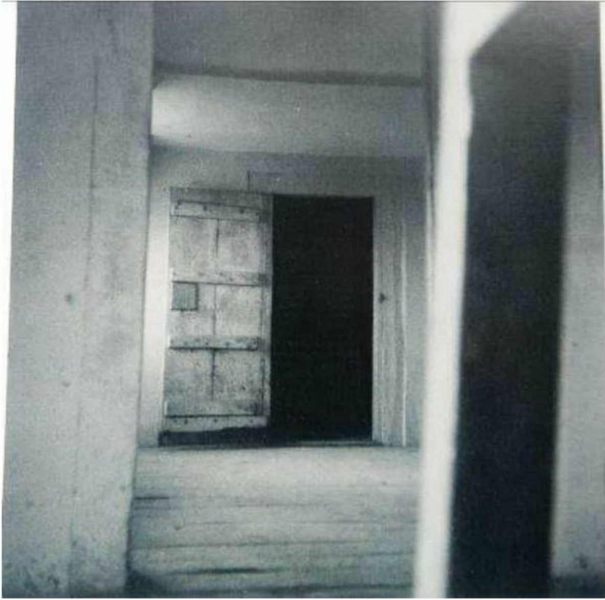
M2: Attic room
