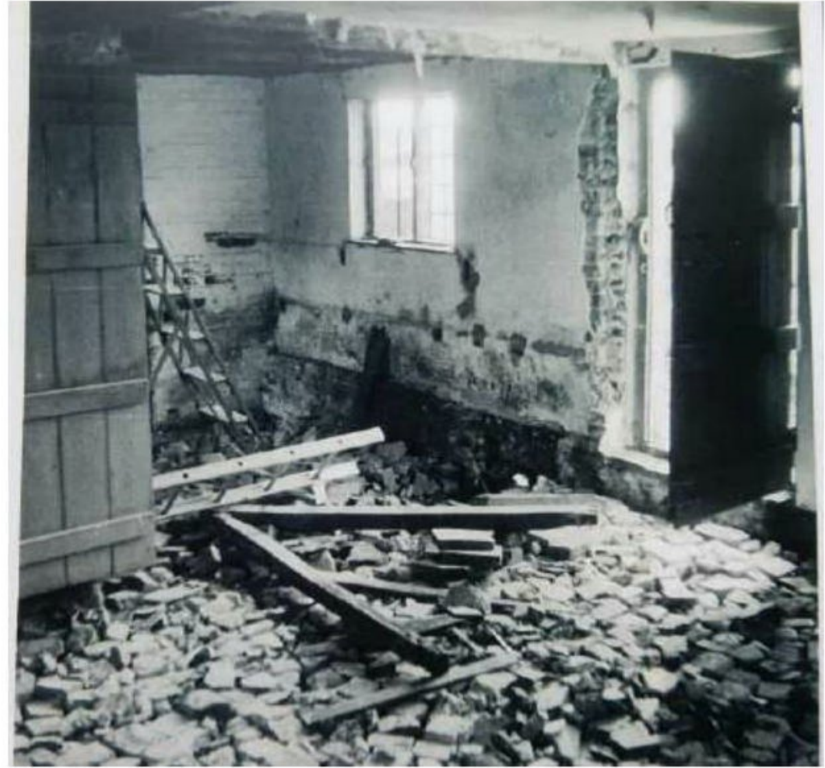
F1: Looking SW from G4 to back door through where demolished wall between G4 & the central bay stood, & into the central bay: the brick floor has been dug out (the person in Photo D1 above is sitting just L of the door in this image)
