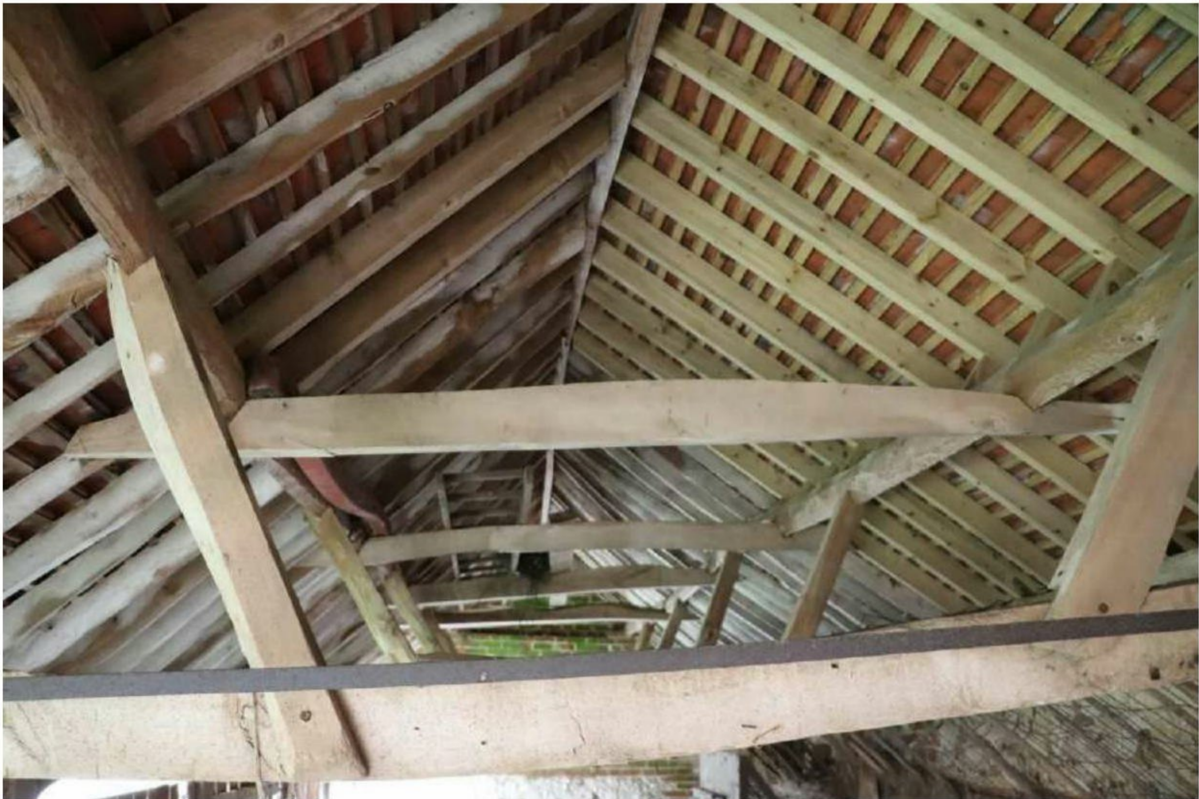
Plate 47: Building B – detail of roof structure
