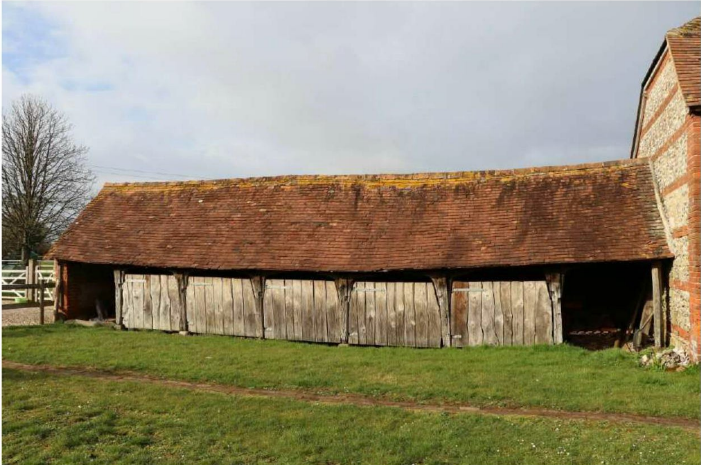
Plate 45: Building B – former cattle shelter shed
