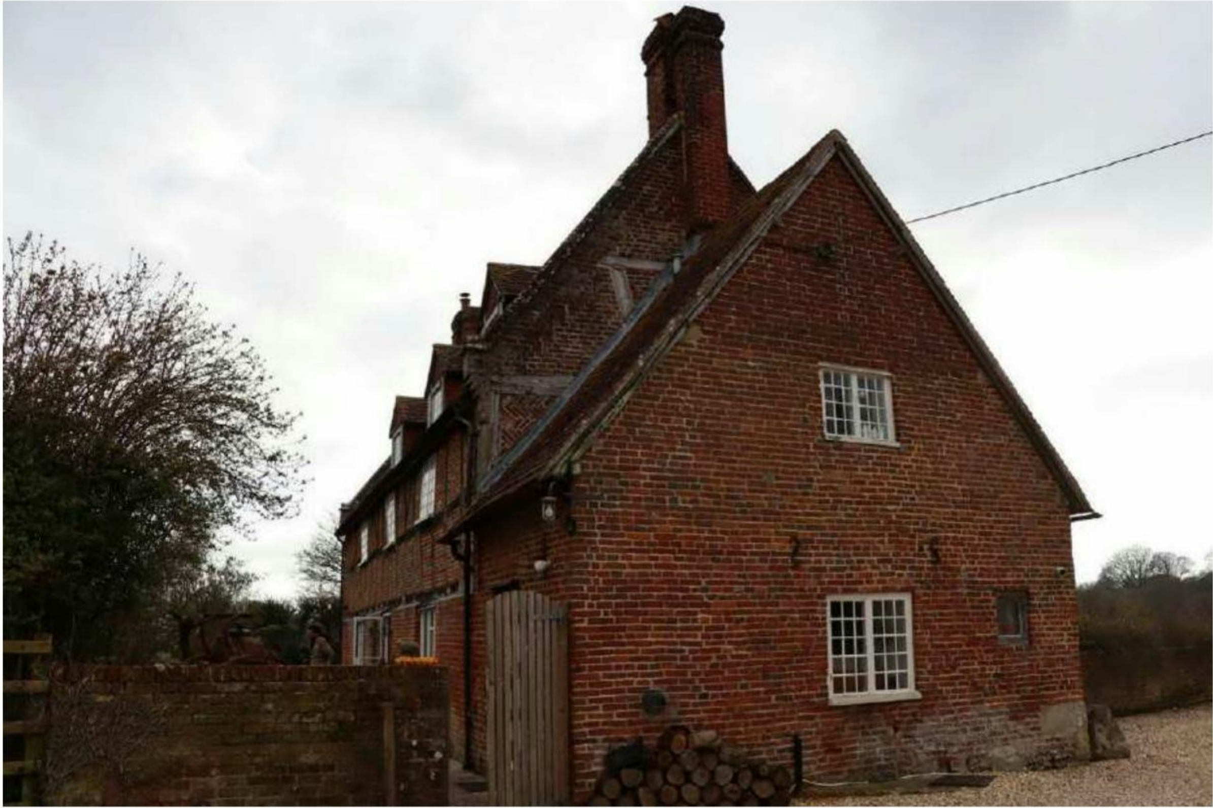
Plate 5: NE gable end of farmhouse and 'brewhouse' addition
