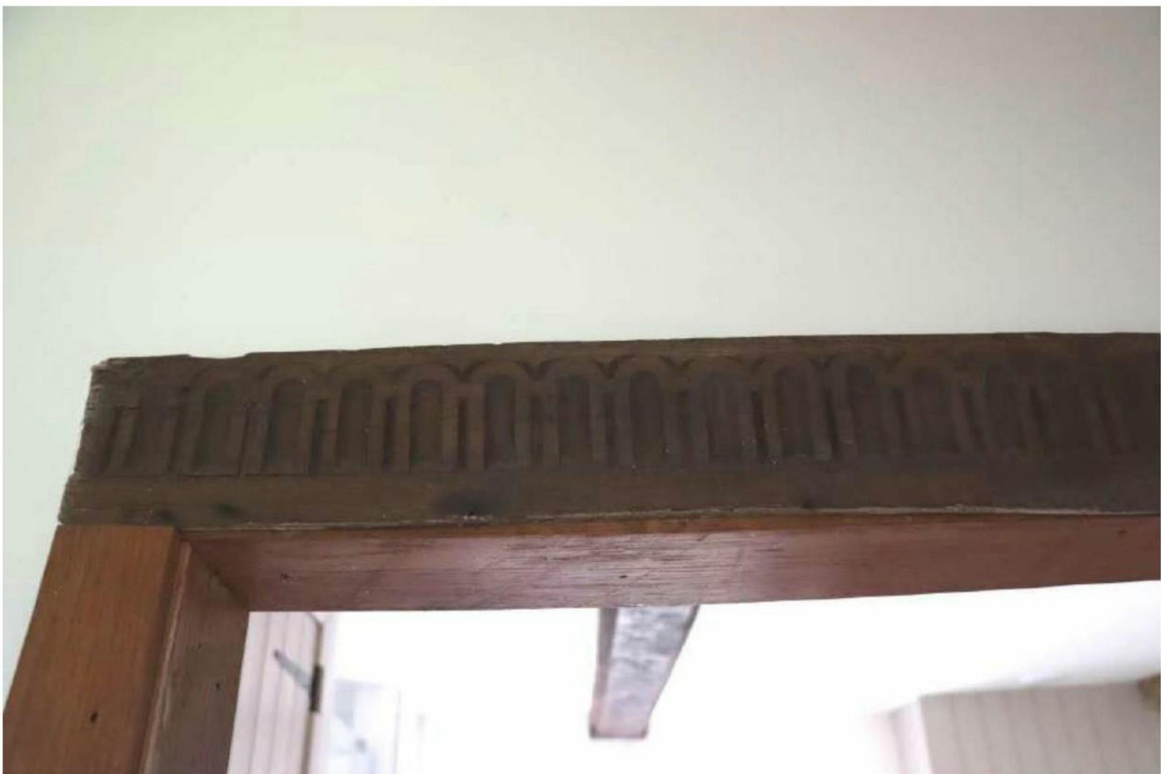
Plate 28: Carved arcading decoration over door into bathroom, F2
