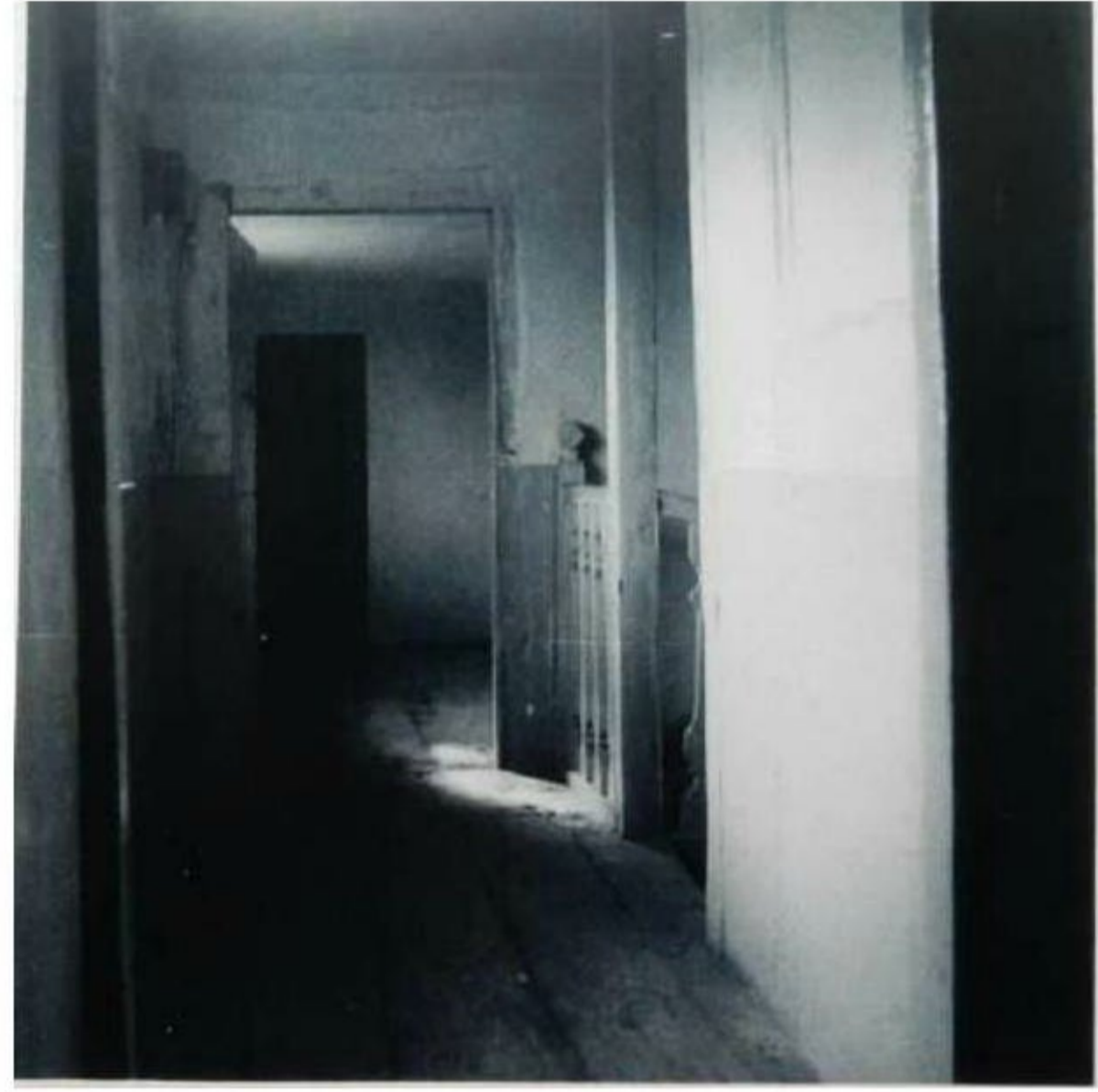
C2: F1, looking SW
