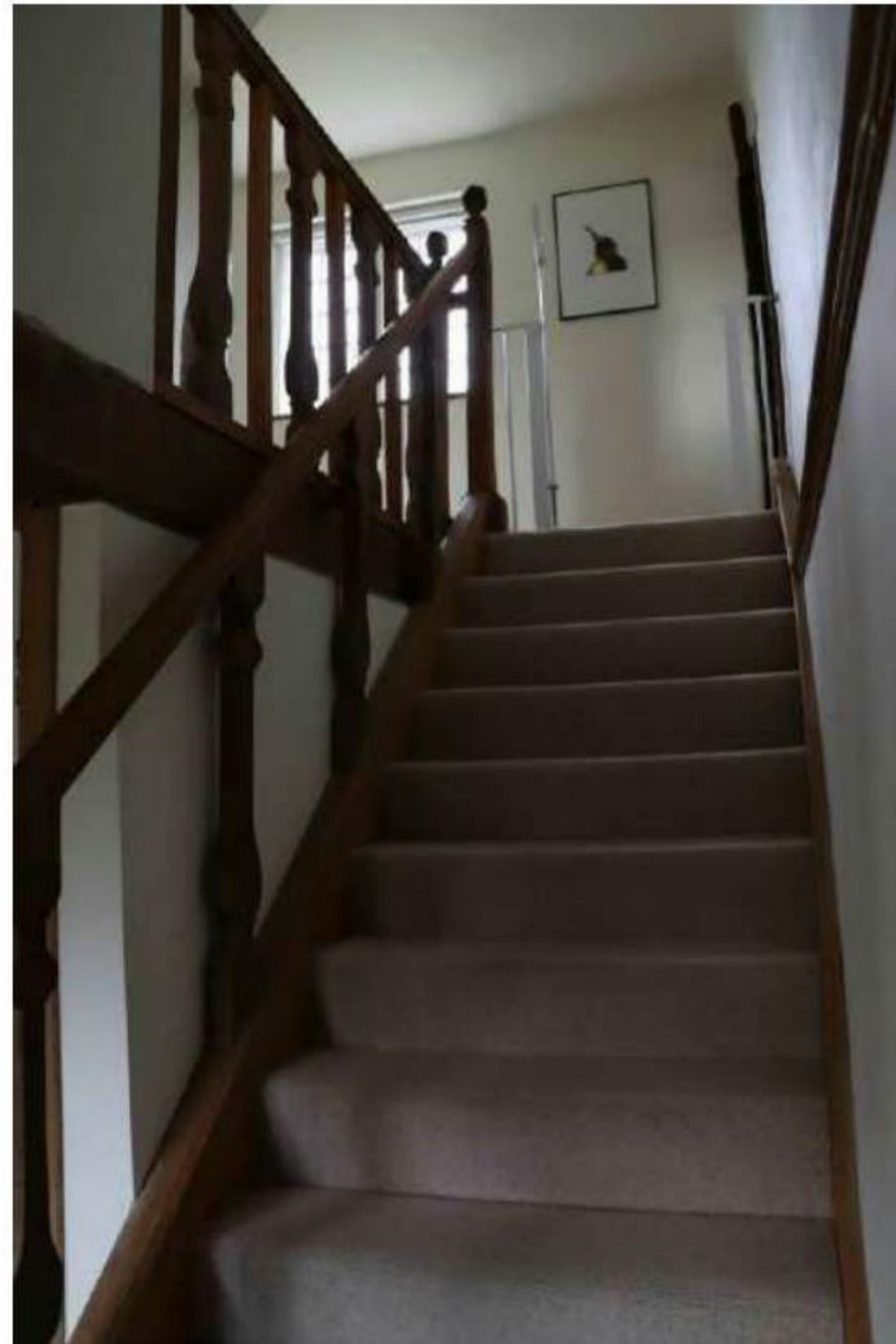
Plate 16: The 1950s' staircase to the first floor; note reused 17 th -century splat balusters
