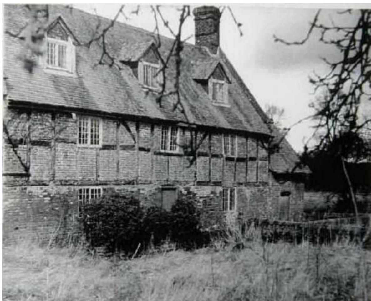
H: Rear elevation before alterations
