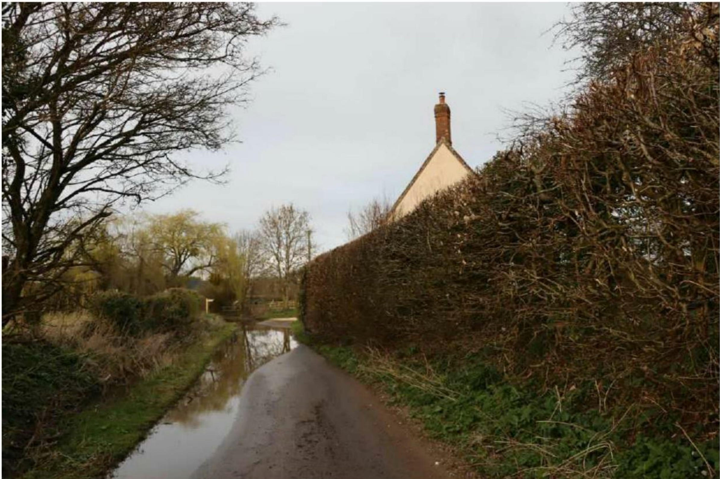
Plate 68: Looking N along Flood Street towards rendered SW gable end of farmhouse
