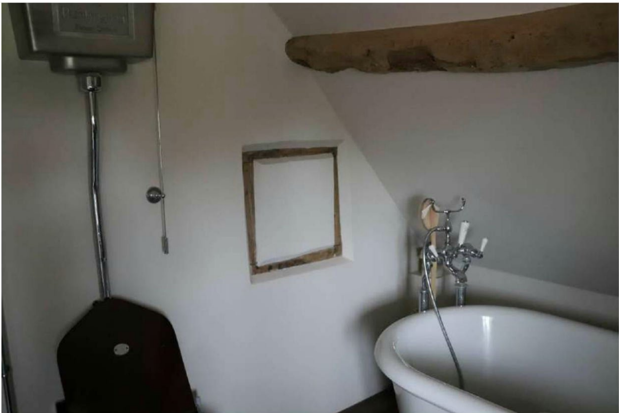
Plate 34: Blocked former window opening in NE gable end of main range, seen in F4
