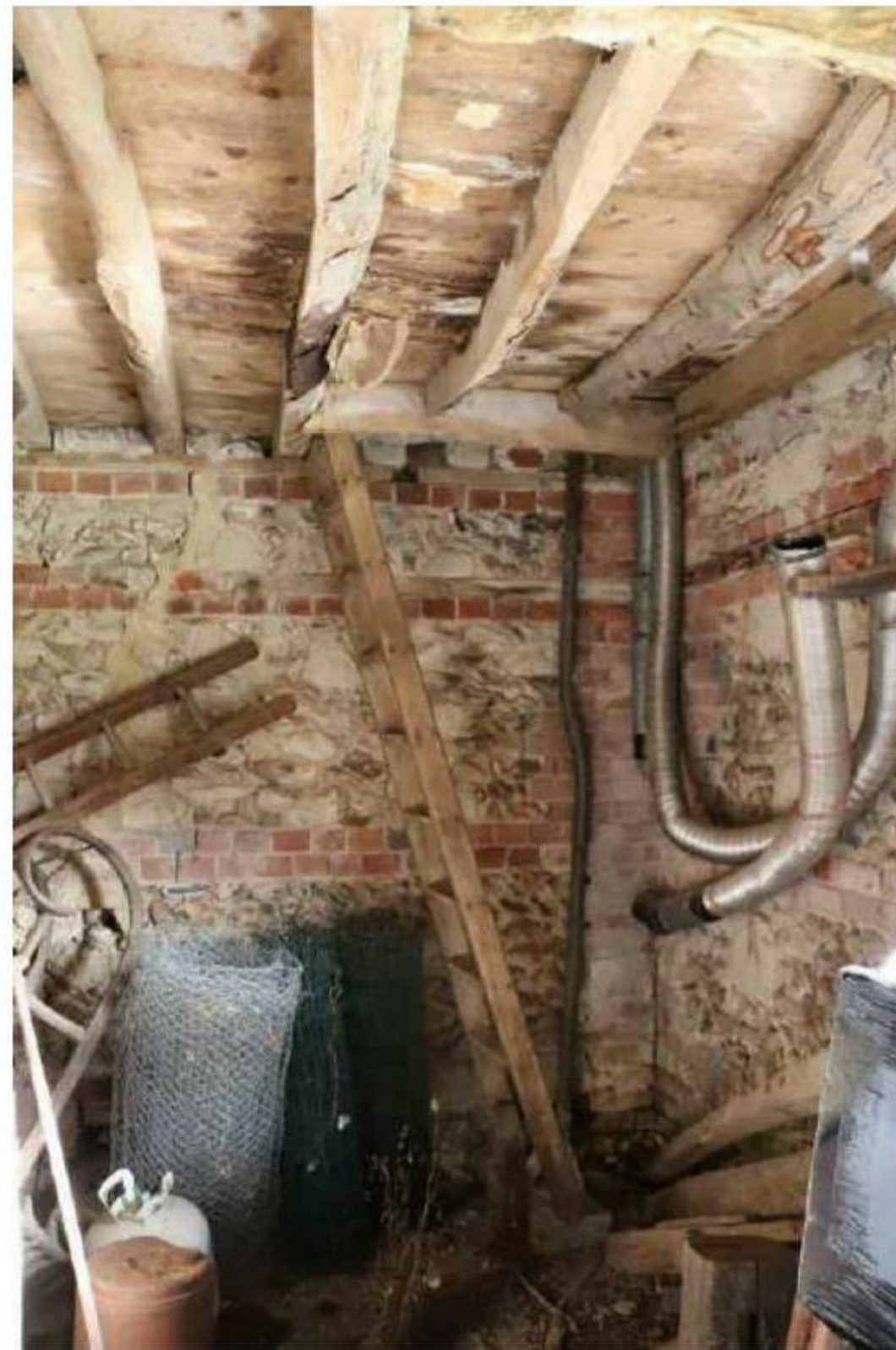
Plate 55: Building C – ladder access to hay loft
