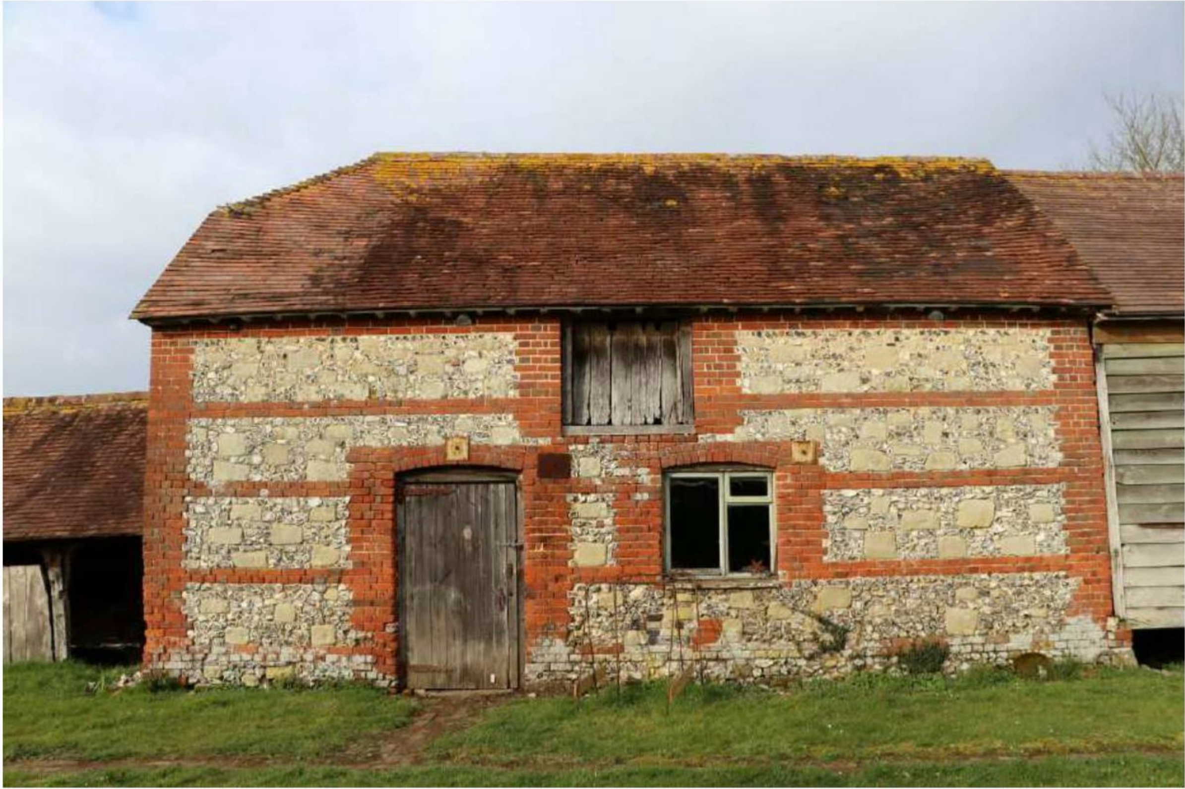
Plate 49: Building C – former stable
