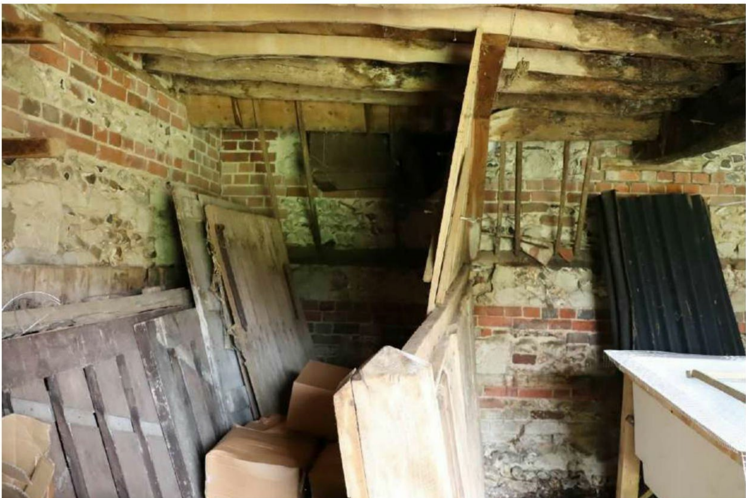
Plate 54: Building C - remnants of wooden manger against rear wall of stalls
