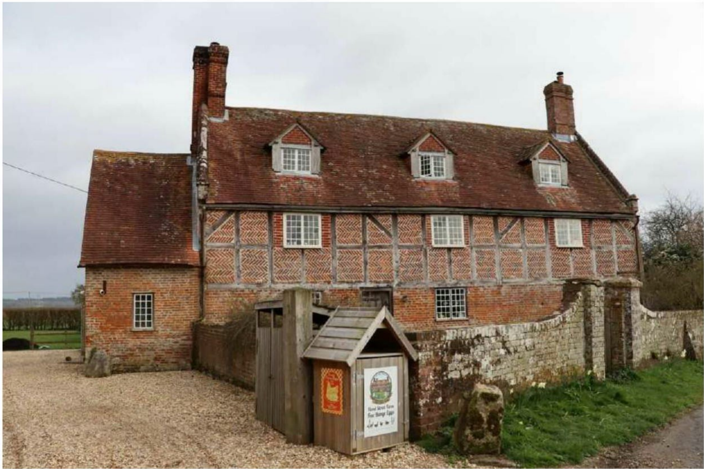
Plate 1: Front (NW) elevation of farmhouse
