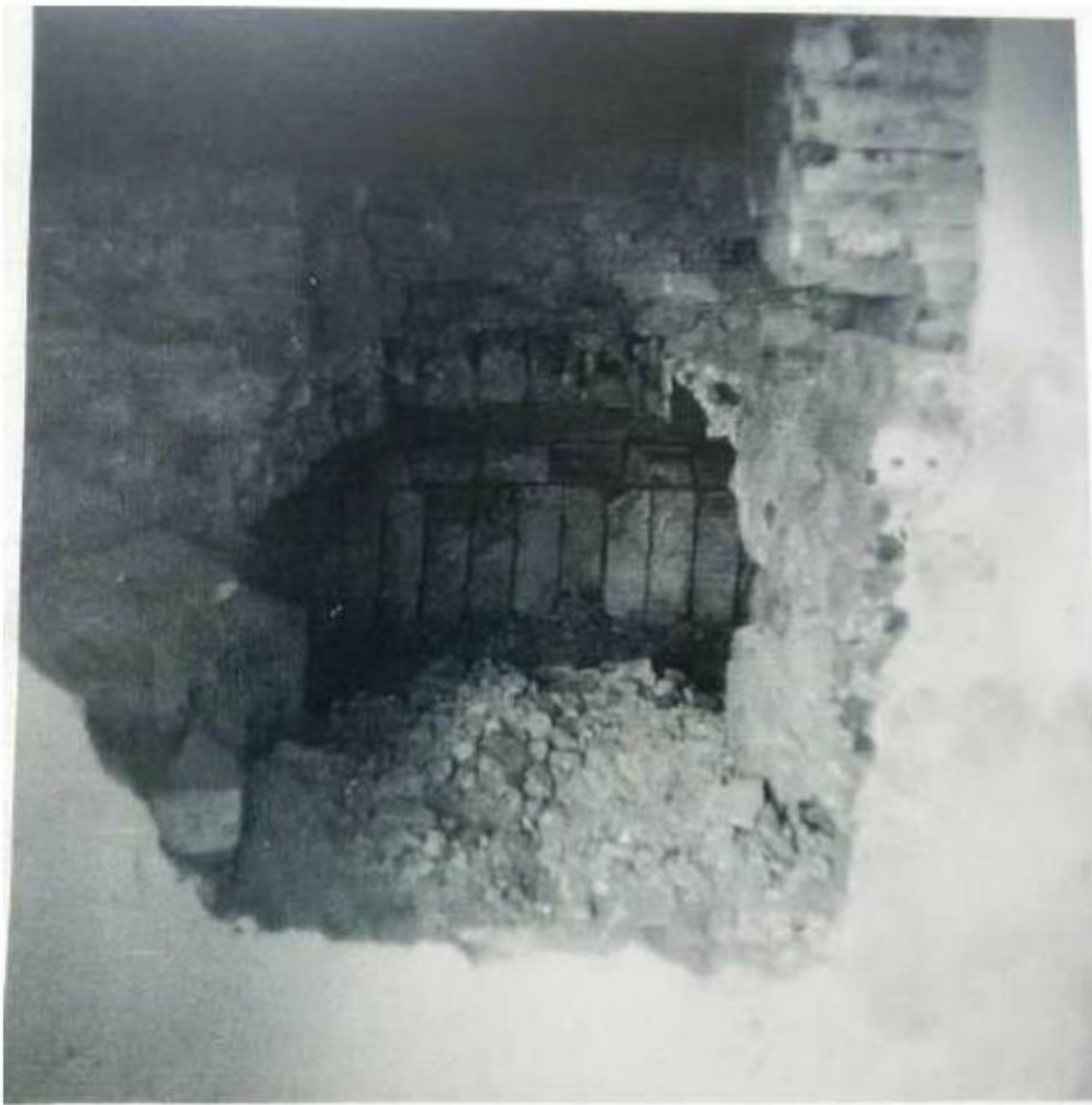
S1: Looking into bread oven before demolition
