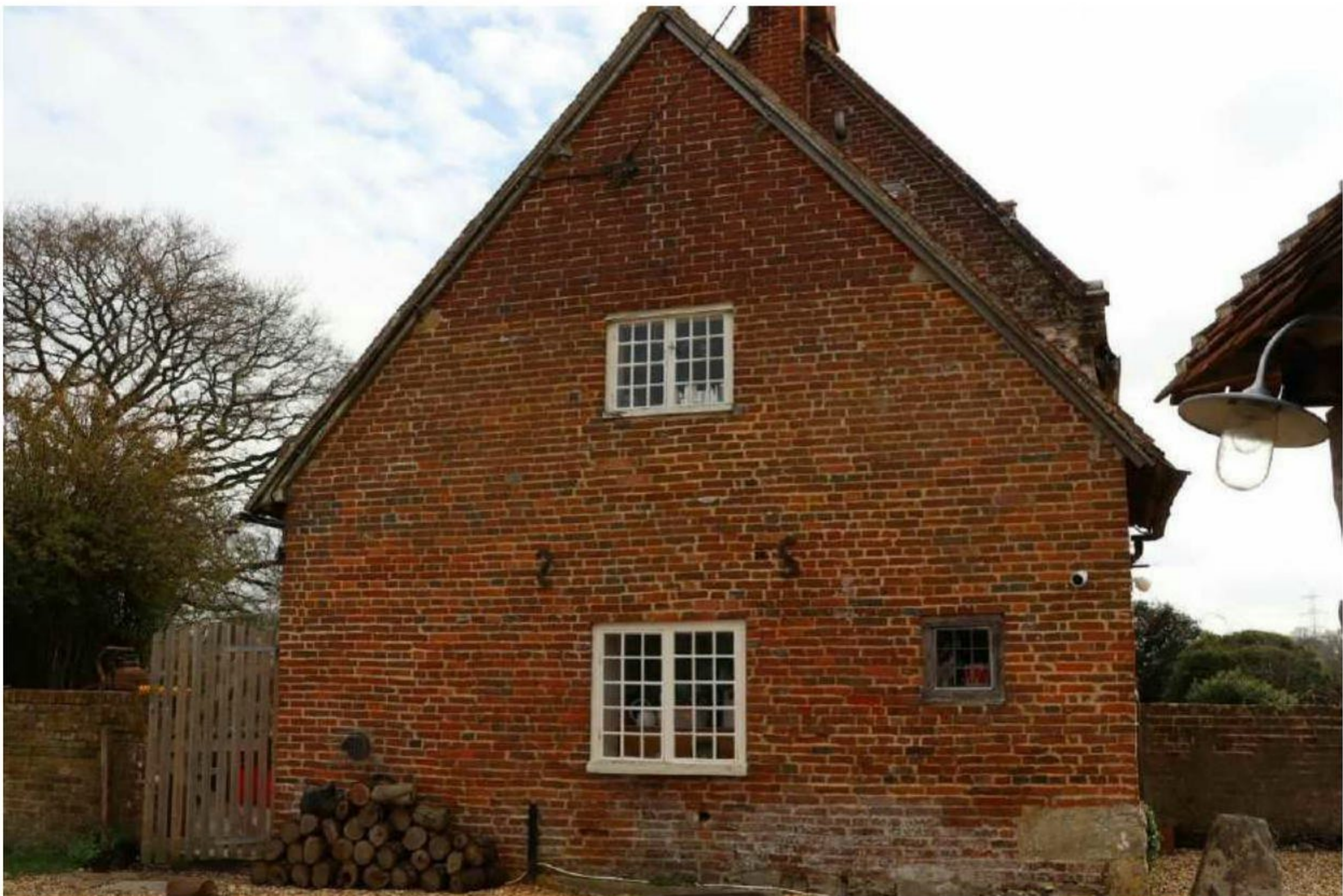
Plate 6: NE gable end of 'brewhouse' addition
