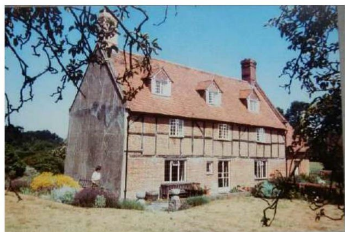
X: SW gable end and rear elevation (1976)
