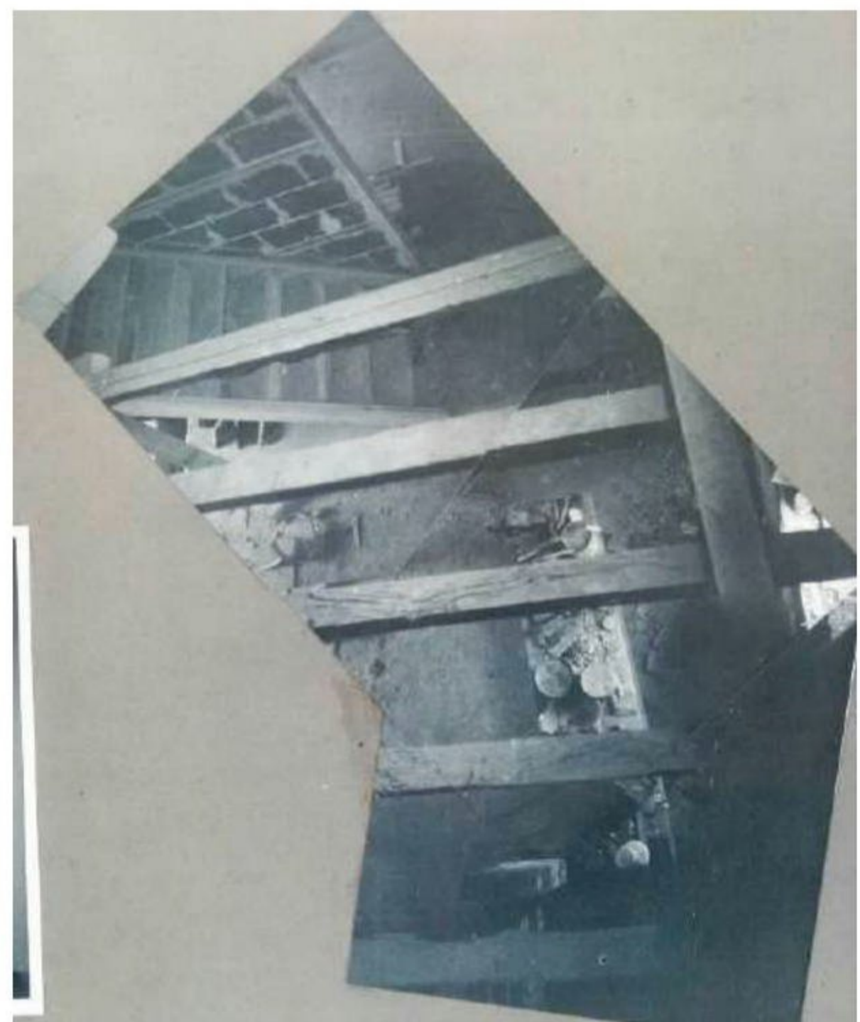
H2: Looking down from F2 into central bay: new staircase, or a temporary one, can be seen against new blockwork wall
