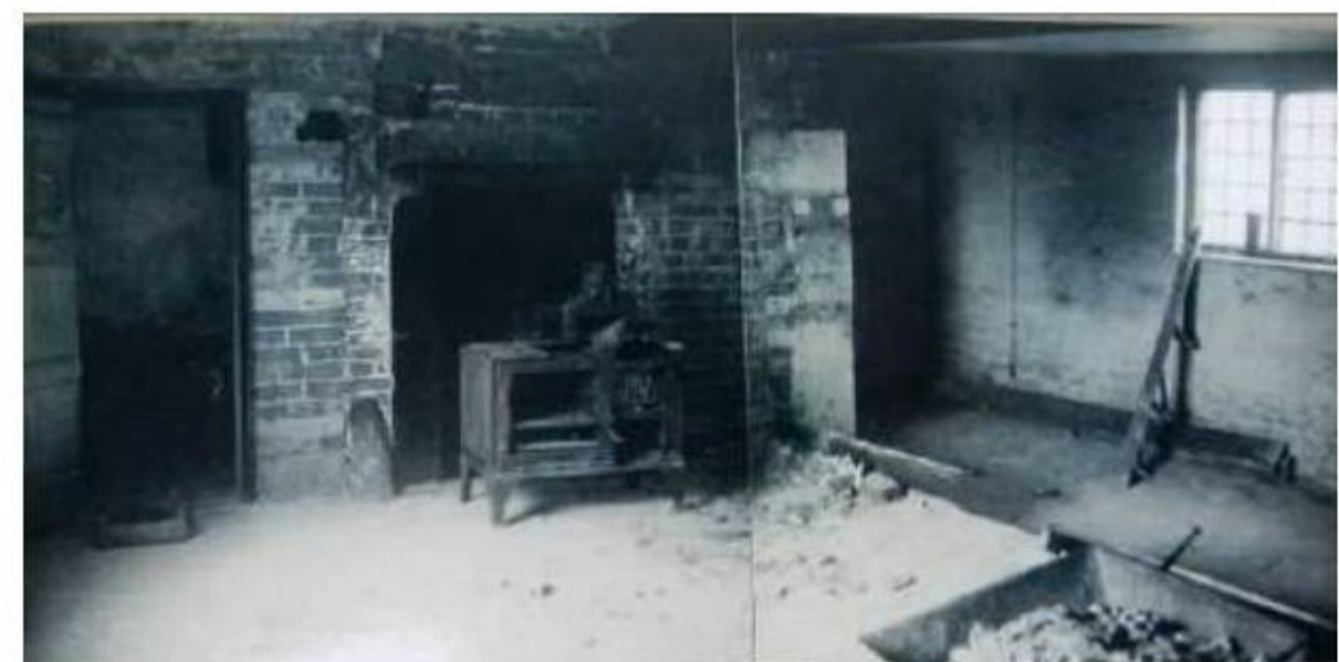
H1: G3, looking SW to partially bricked-in inglenook
