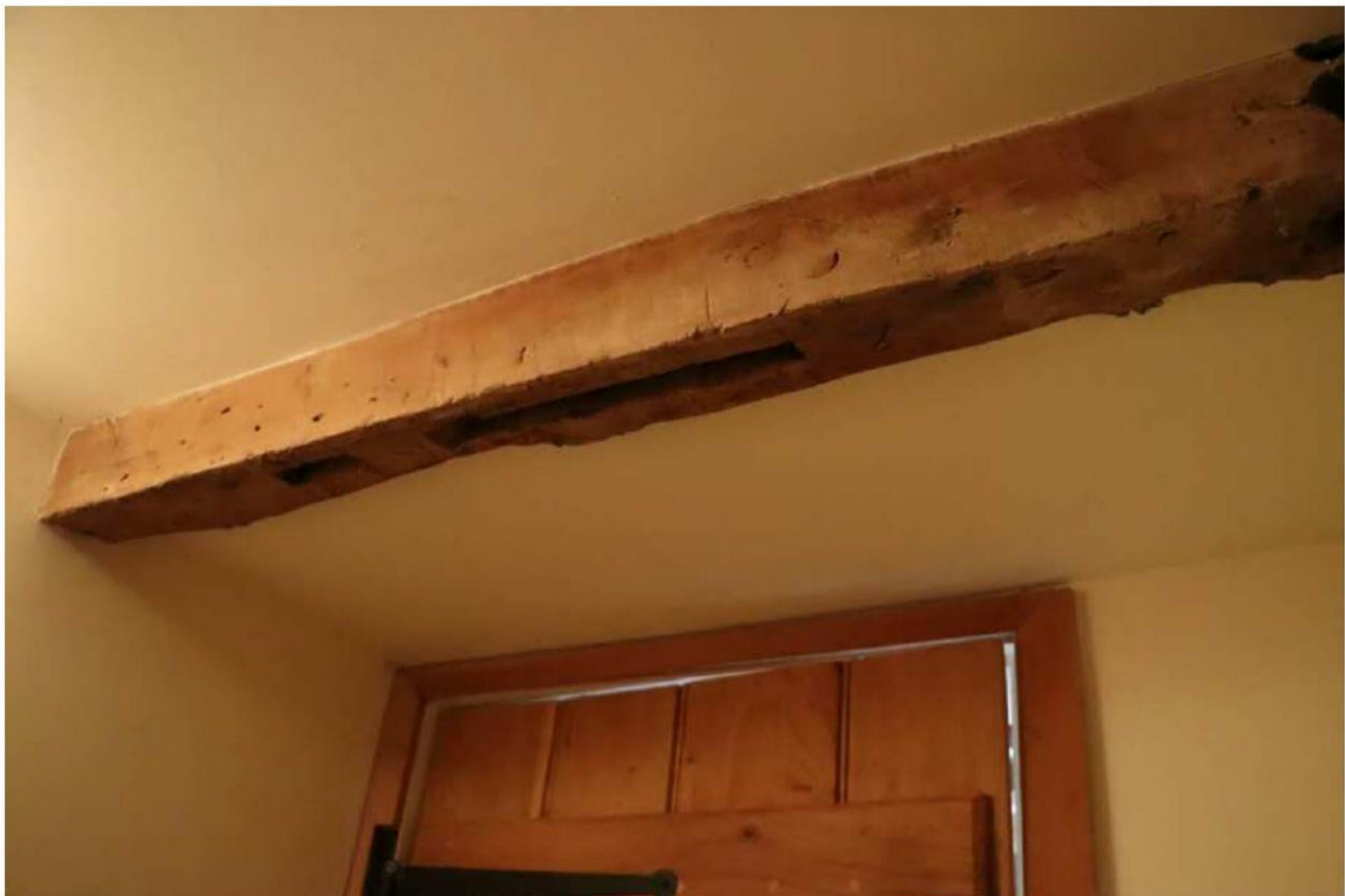
Plate 12: G1: original beam with empty mortises from the removal of the timber-framed wall dividing the northern from the central bay
