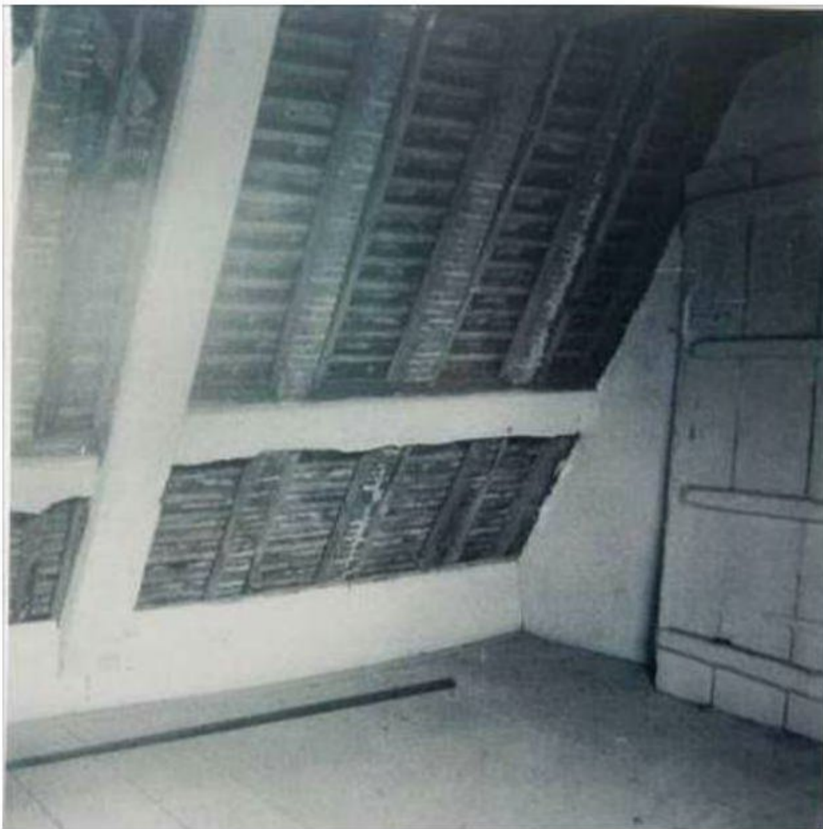
N2: Attic room
