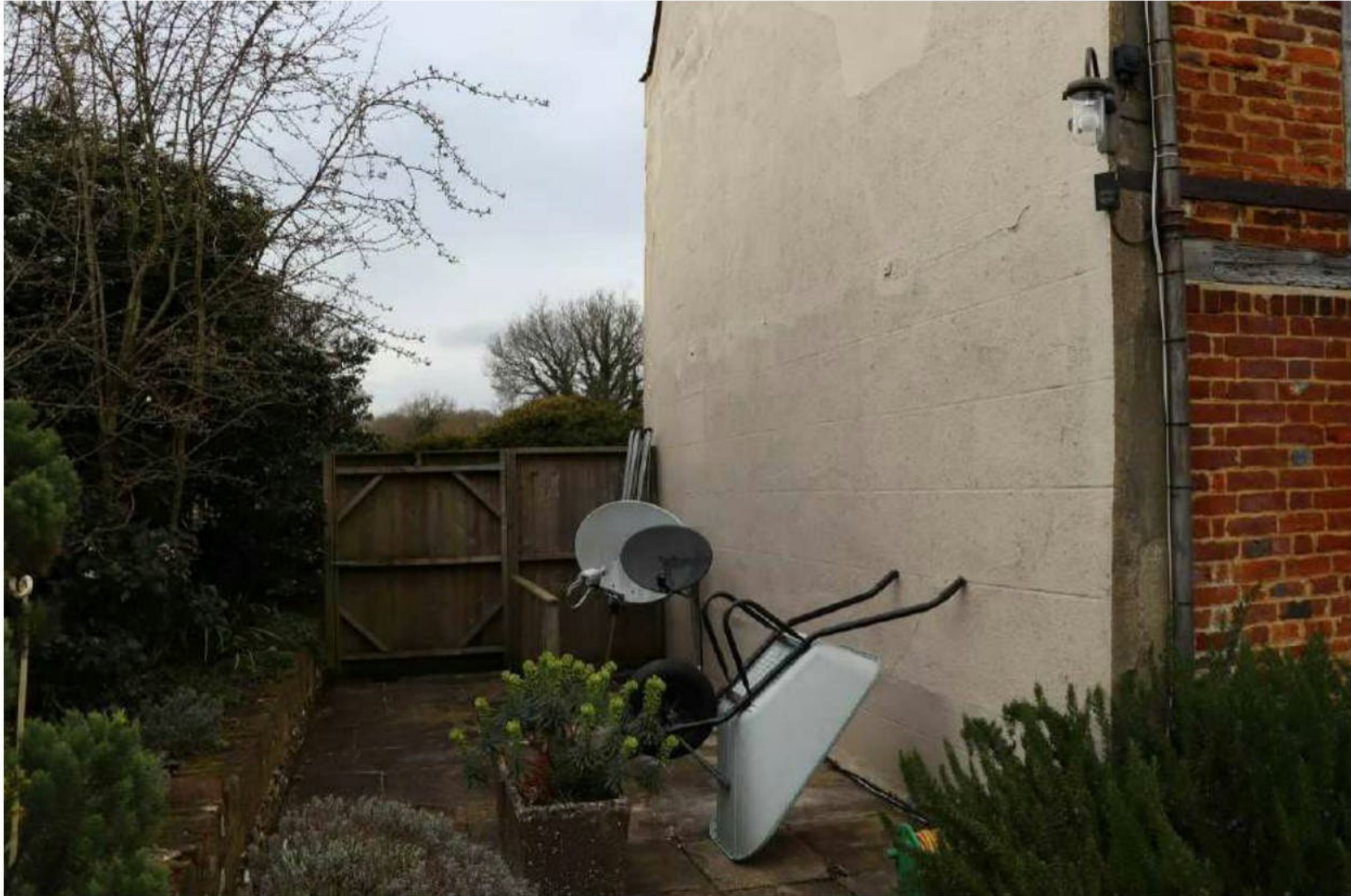
Plate 11: Base of the SW gable end, from where an earth bank was removed in 1957
