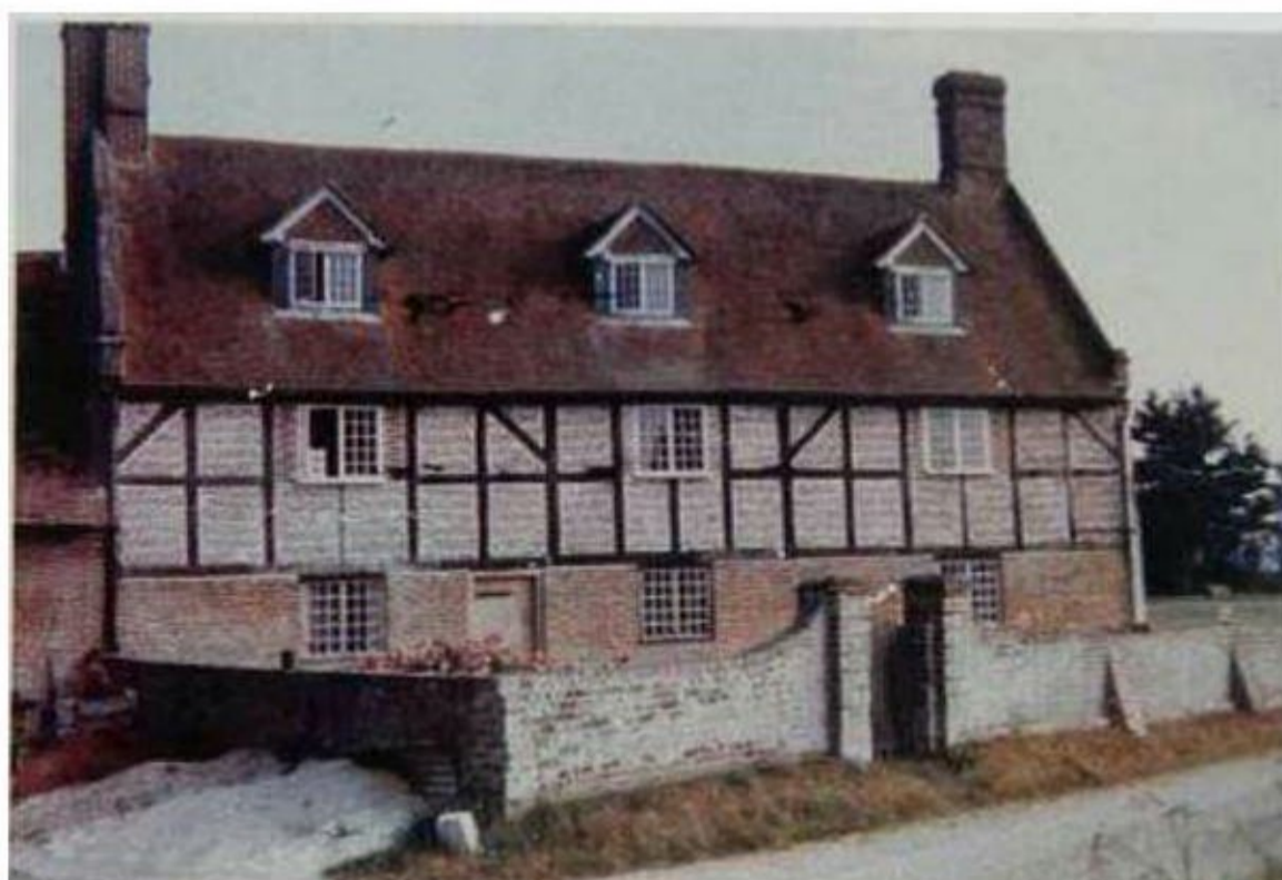
F: Front elevation – September 1959, following works
