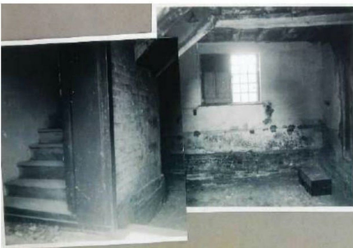
A1: The reverse view of that above: looking NW across rear passage into the central bay
