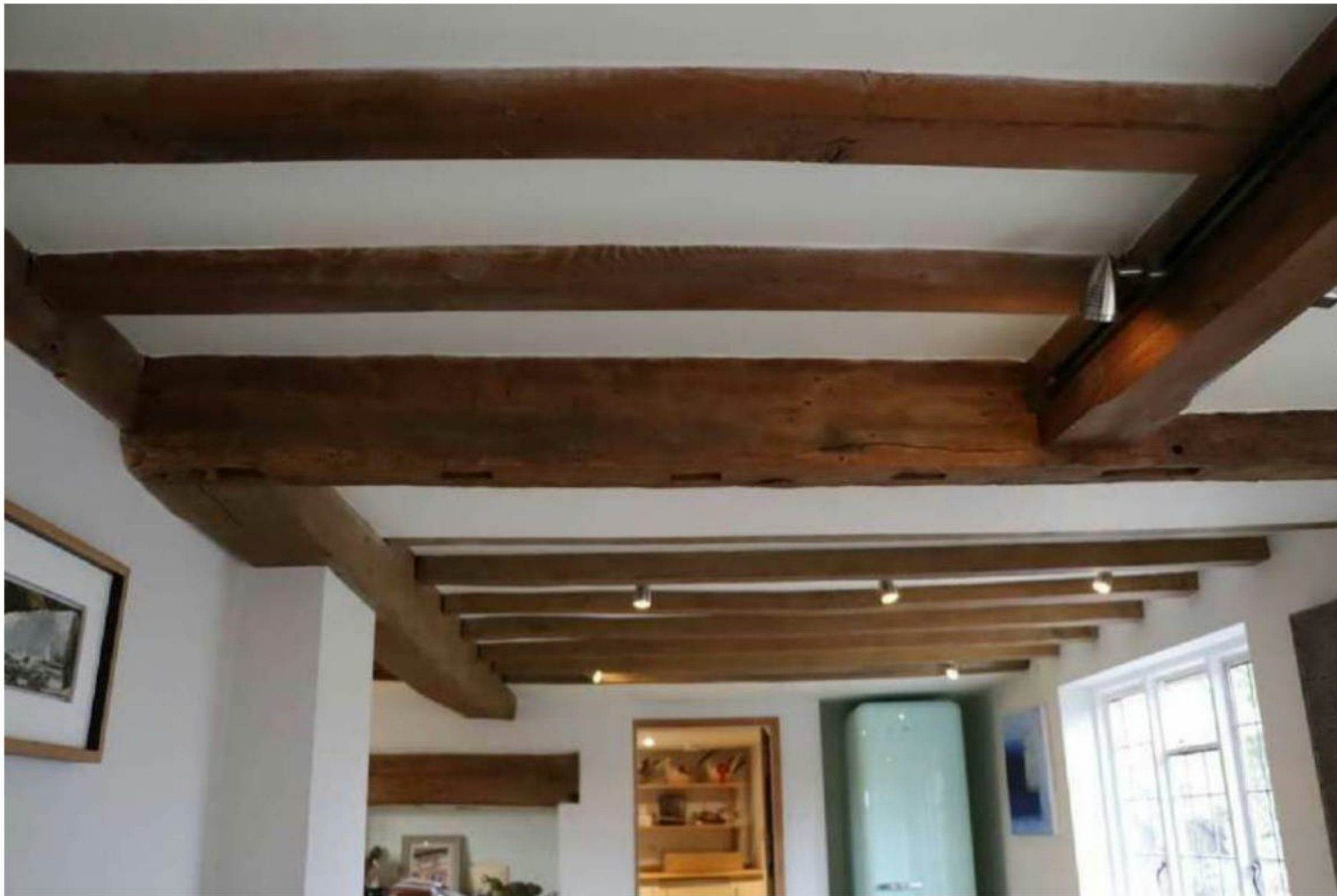
Plate 13: G4, looking NE from central bay into NE bay: the beam with empty mortises across the centre of the image marks the position of the original timber-framed wall dividing the bays; the chamfered and stopped beam joining it to left marks the original extent of the space in the NE bay, while the chamfered beam to right was inserted in the 1950s
