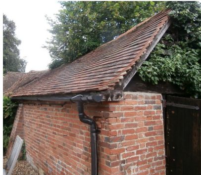
Outbuilding to be demolished
