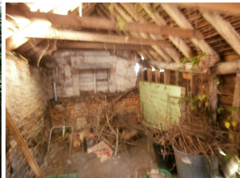
Interior of outbuilding
