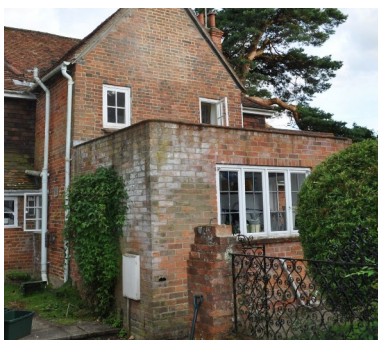
Extension to be demolished
