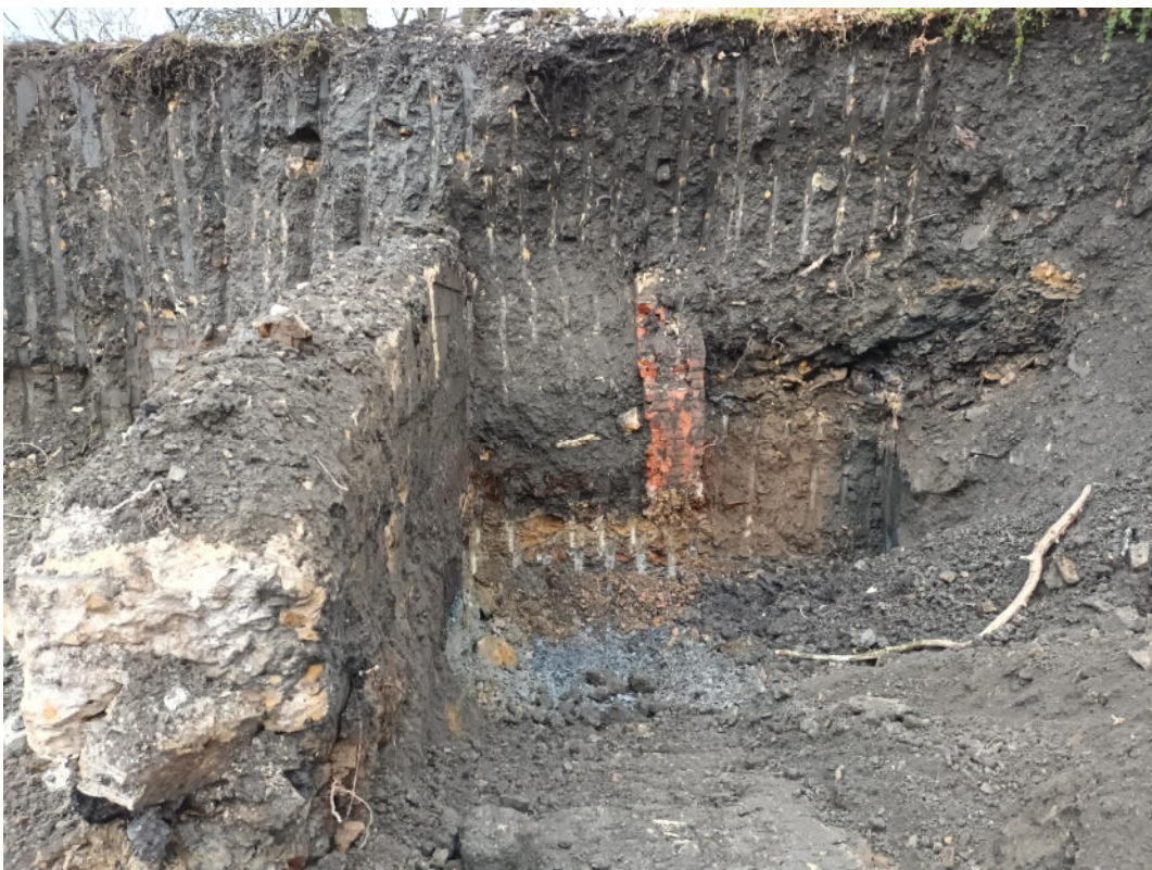
Plate 2: View NNW of adit entry. Note brickwork wall and presence of natural soils and rock at base.
