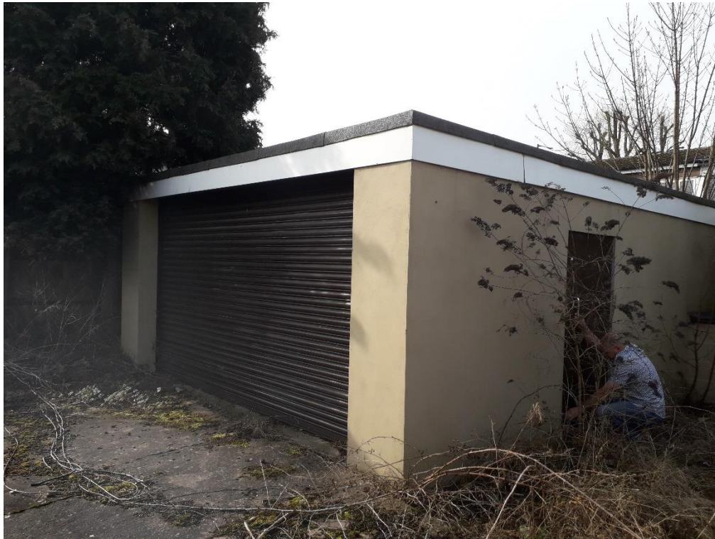
Image 1: Building viewed from North
