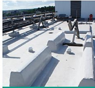
LIQUID APPLIED WATERPROOFING
