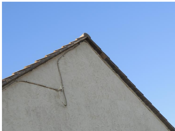
Photo 5: Note tight seal to gable wall
