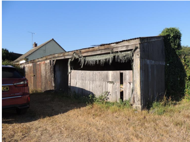
Photo 13: Eastern and northern elevations of shed
