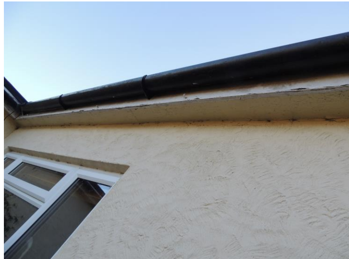
Photo 7: Typical section of eaves showing tight seal
