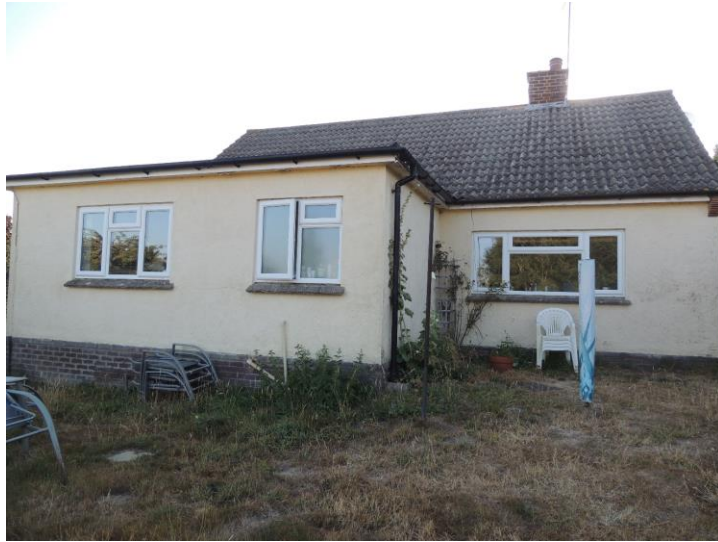
Photo 3: Western elevation. There was a tight seal to the flat-roofed extension
