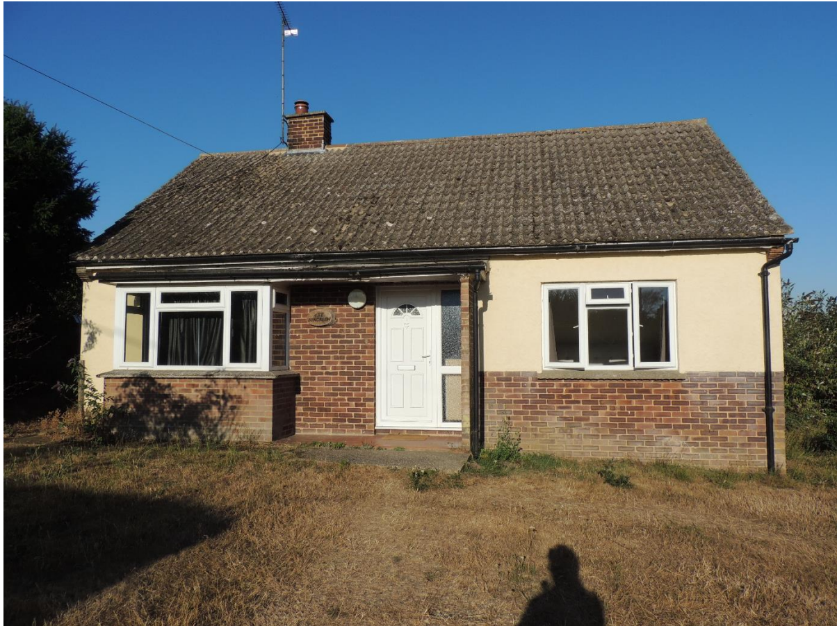
Photo 1: Front (eastern) elevation. Note tight seal to roof tiles
