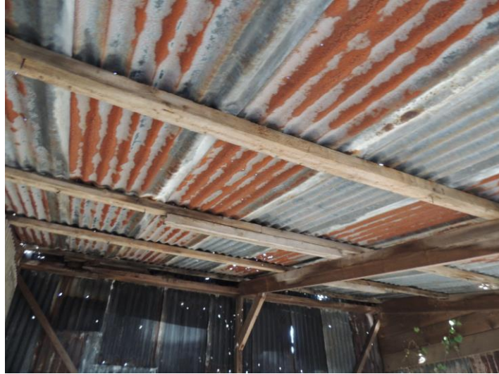
Photo 16: The roof of the shed had no features that might be occupied by bats
