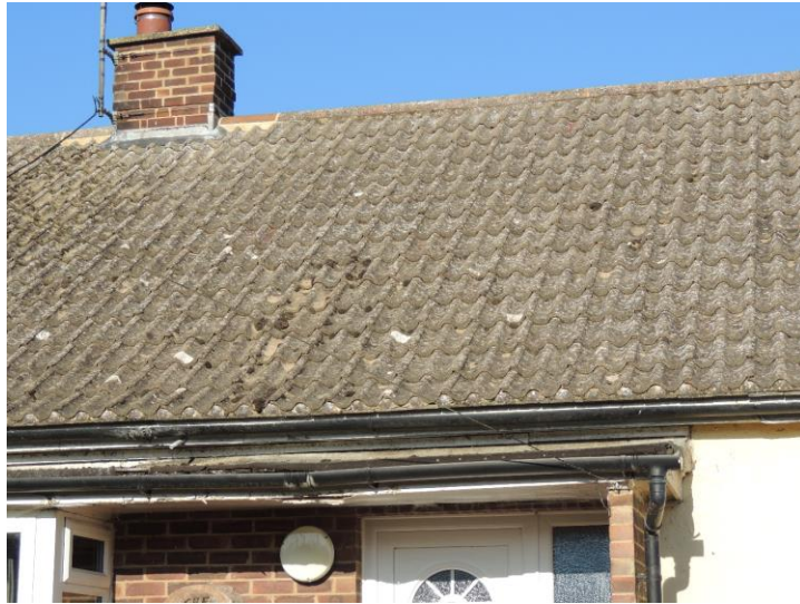
Photo 6: Note tight seal to roof tiles
