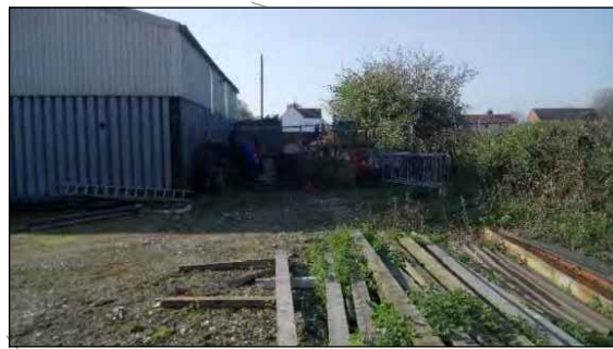
VIEW ON EXISTING BUILDING
