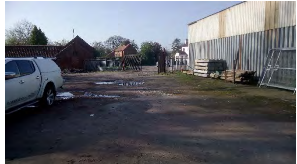
Plate 4: The central area of the site and the eastern elevation of the agricultural building
