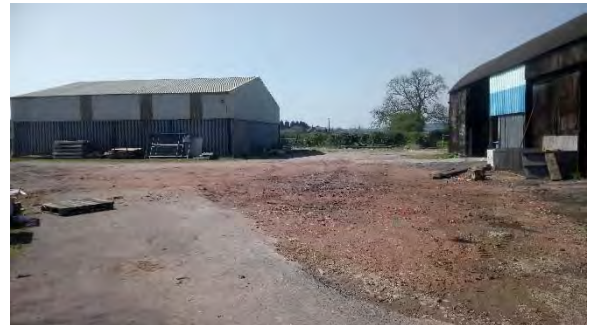
Plate 6: The northern part of the site viewed from the east
