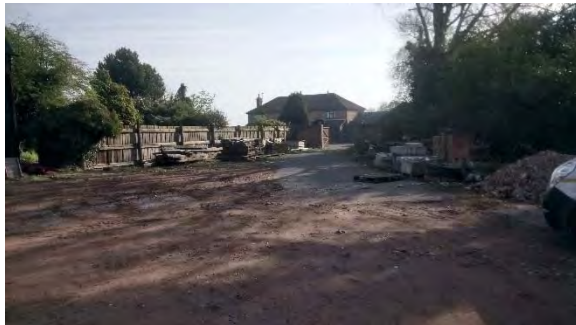
Plate 5: The north-eastern area of the site
