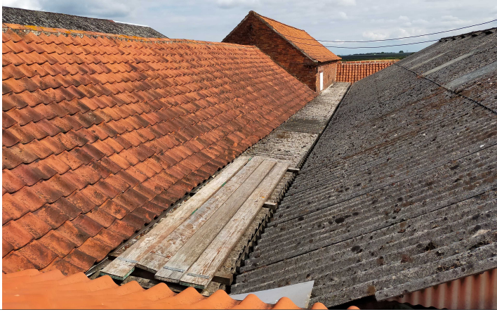
Photo 7 – Aerial photo from northeast corner of site looking due southwest.
