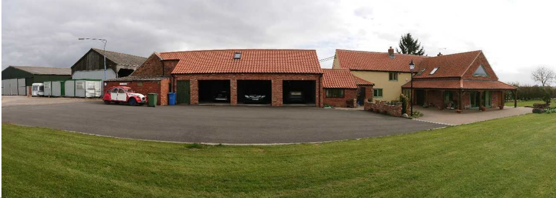
Photo 6 – South west elevation over enclosed yard shed roof.
