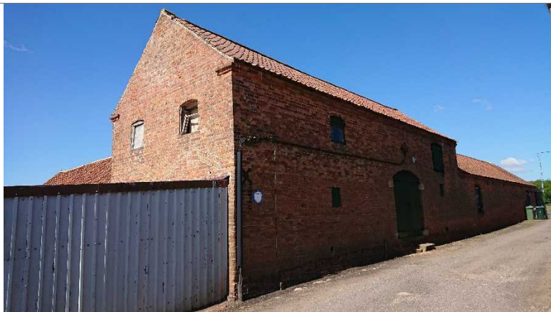
Photo 3 – South east elevation of Unit 1.
