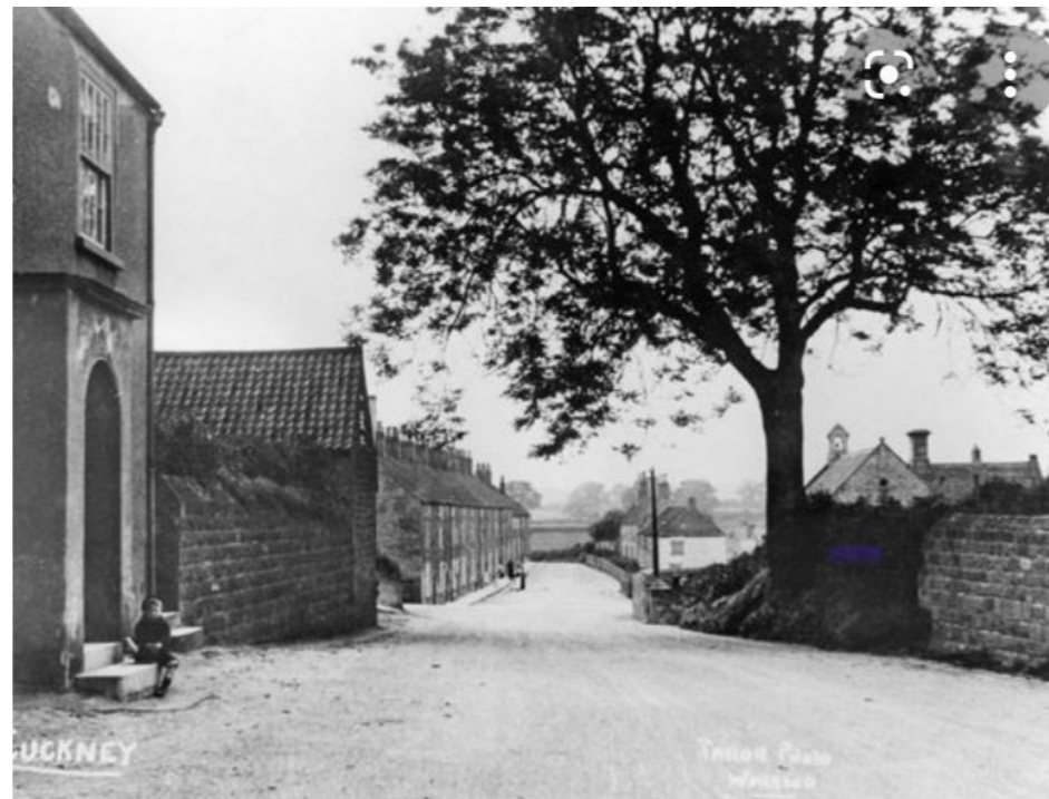
1900 View towards the Cottage from the A60 showing hipped roof and additional window to gable elevation of the cottage. (Source : Picture Nottingham)
