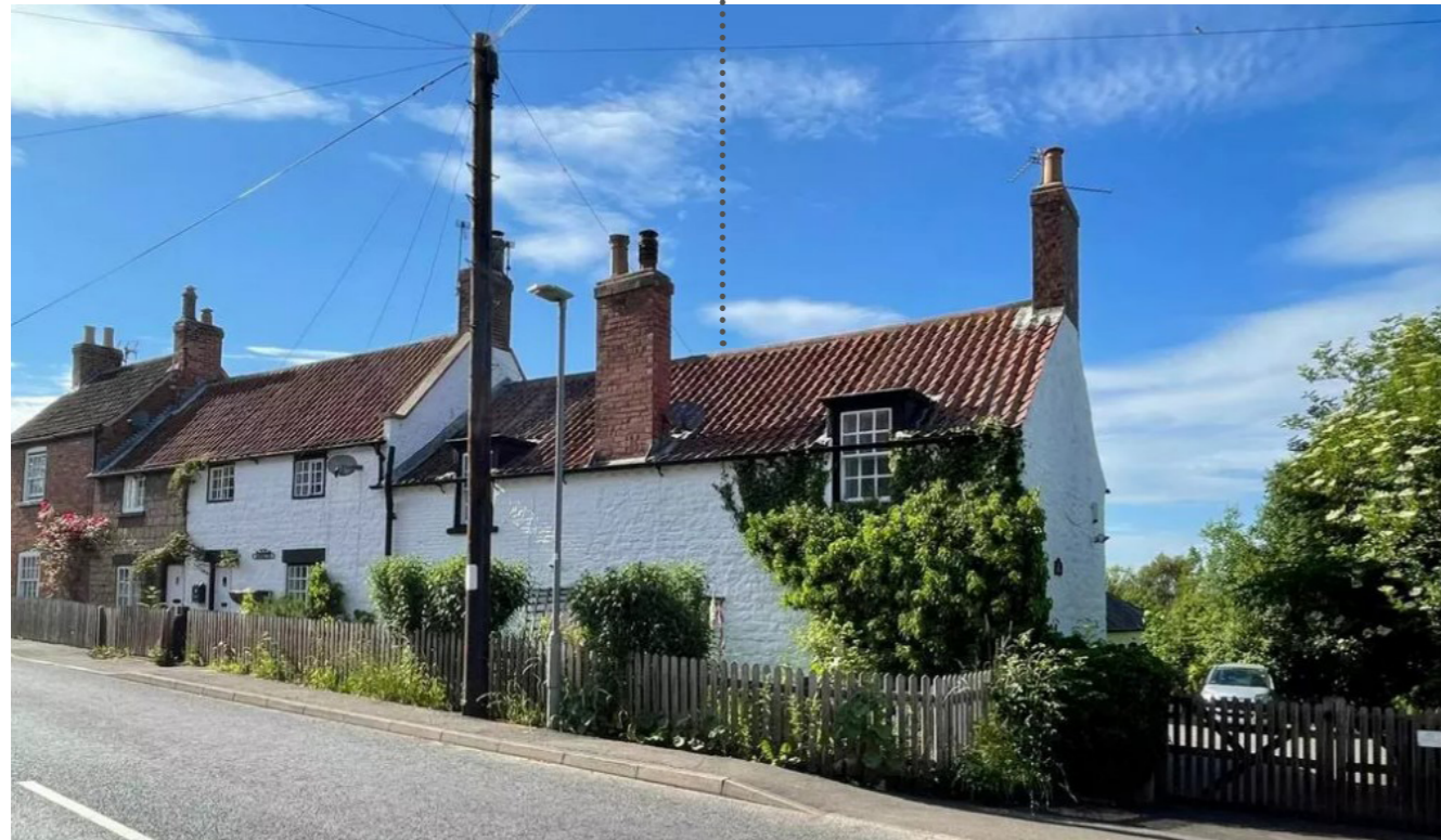
1 View looking north from Creswell Road
