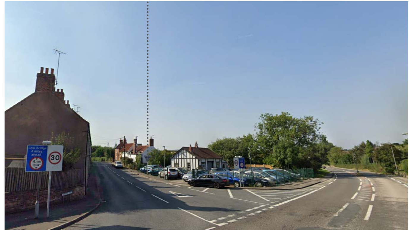
2 View looking west from crossroads of A60 and Creswell Road
