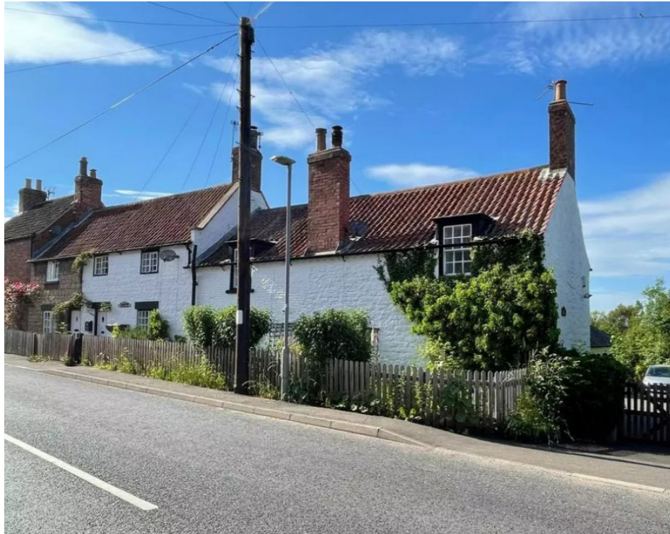
1 Front elevation of The Cottage from Creswell Road
