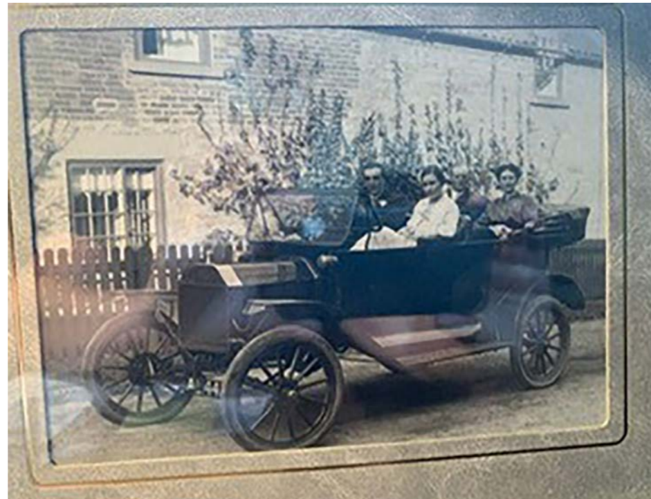
Date unknown possibly 1900s View of front of the Cottage showing combination of brick and stone walling prior to painting (Source : Unknown via the property owner)
