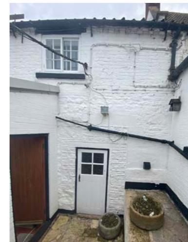
2022 Rear of The Cottage showing varying infill areas of stone and brickwork. (Photograph: Author's own)
