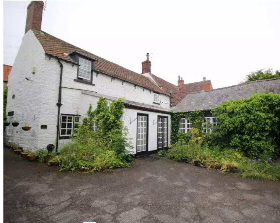
2 View of 2001 addition from side/rear driveway
