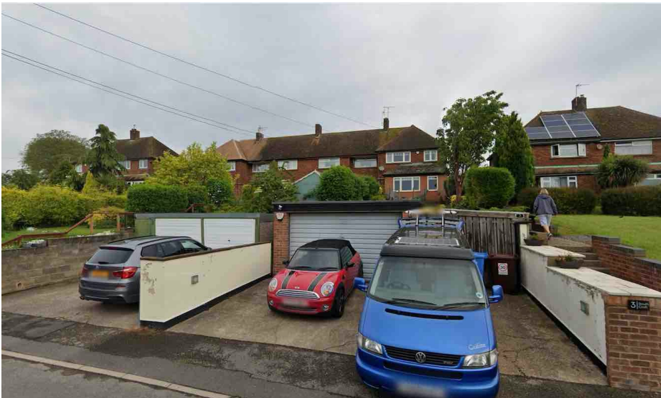
Top Street houses – two storey located on the upper terrace with garaging on the lower level below.
