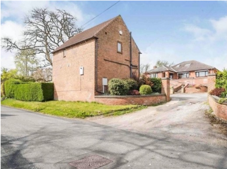
View from Top Street towards the existing house
