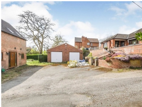
View of sloping drives.
