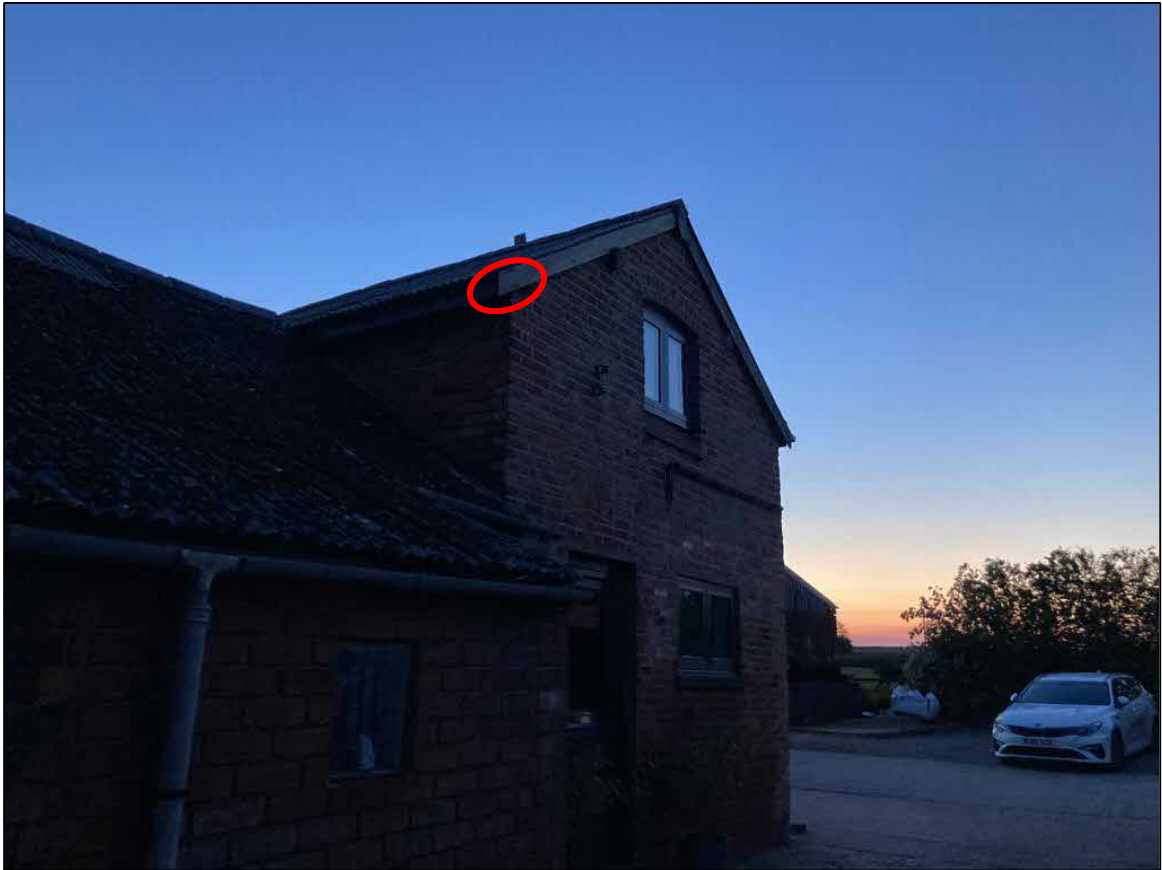
Figure 3. Roost Location 1 circled in red. Pertaining to a cavity within the brickwork behind the barge board. Following inspection, the cavity does not allow access into the interior of the building.
