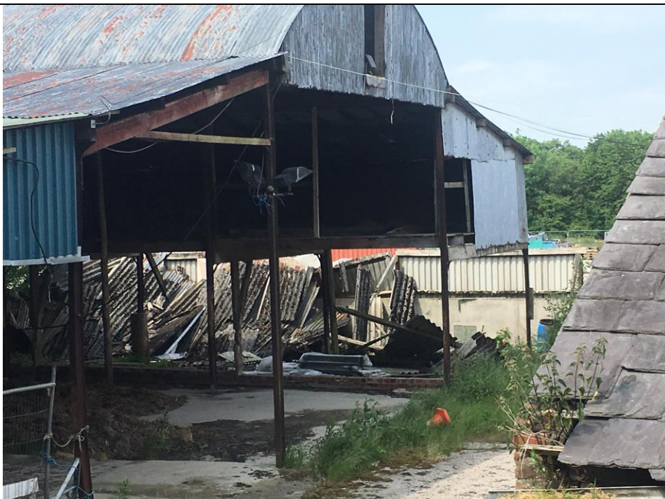
Looking east into the central area of the farm buildings, showing construction debris and a mix of corrugated iron, plastic and asbestos cement roofing. Unidentifiable agricultural waste observed within the building structure.
