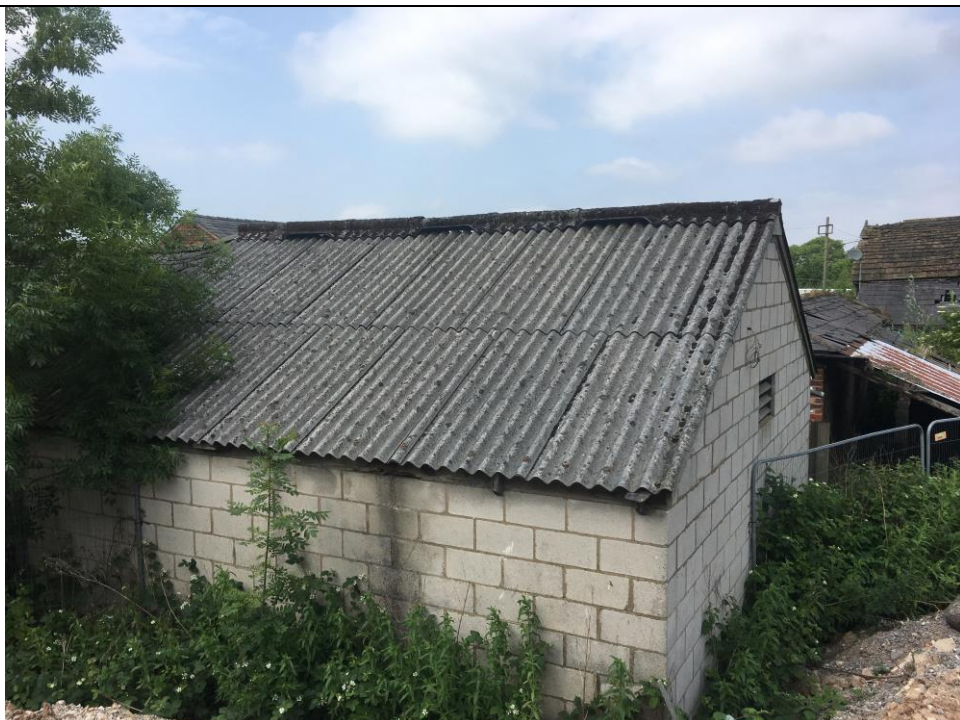
Looking south west towards the previous farming buildings, showing vegetation out-break and potential asbestos cement roofing.
