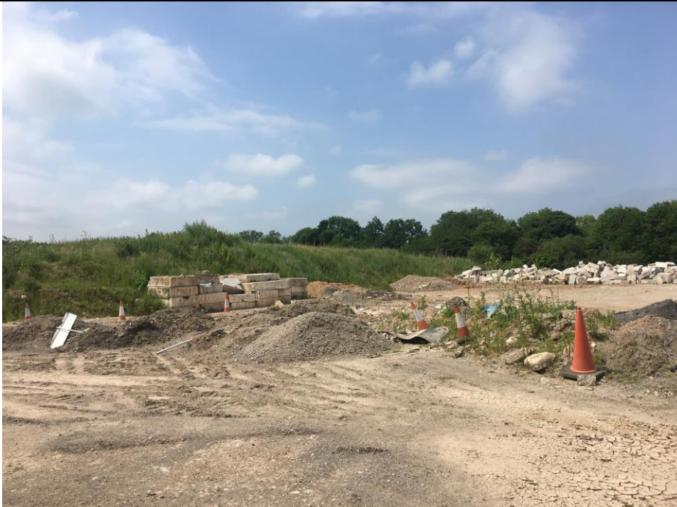
No 8 | Stockpile of unidentified waste on south west boundary of listed farm house. Material has been previously sorted, however evidence of broken tarmac and mixing is present. Grass mound is previously covered construction waste (No 10), looking west.
