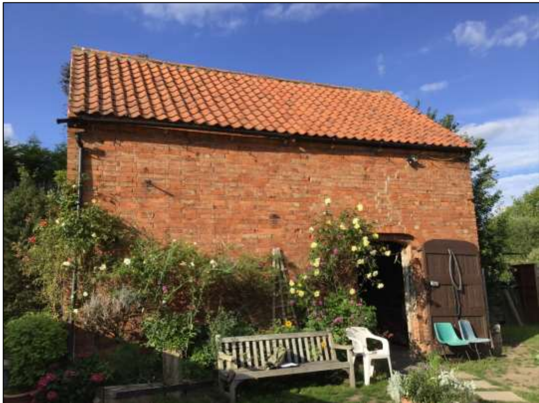
Photograph 1.1 : The southern elevation of the surveyed barn viewed from the driveway.
