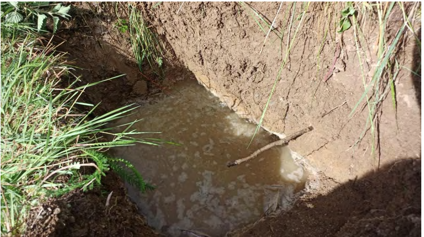
Photo 4 – Test hole 2 – 800mm deep. Water level at 300mm
