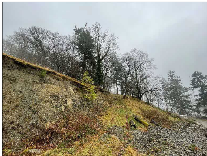
Plate 9. Disturbed ground and scree at south-eastern corner of site
