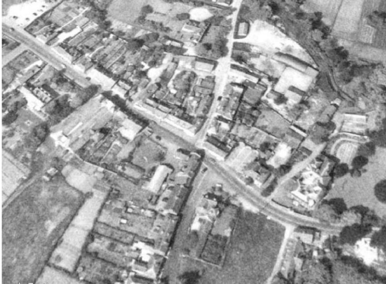
1952 Photograph of the Anchor Inn (source: Historic England)
