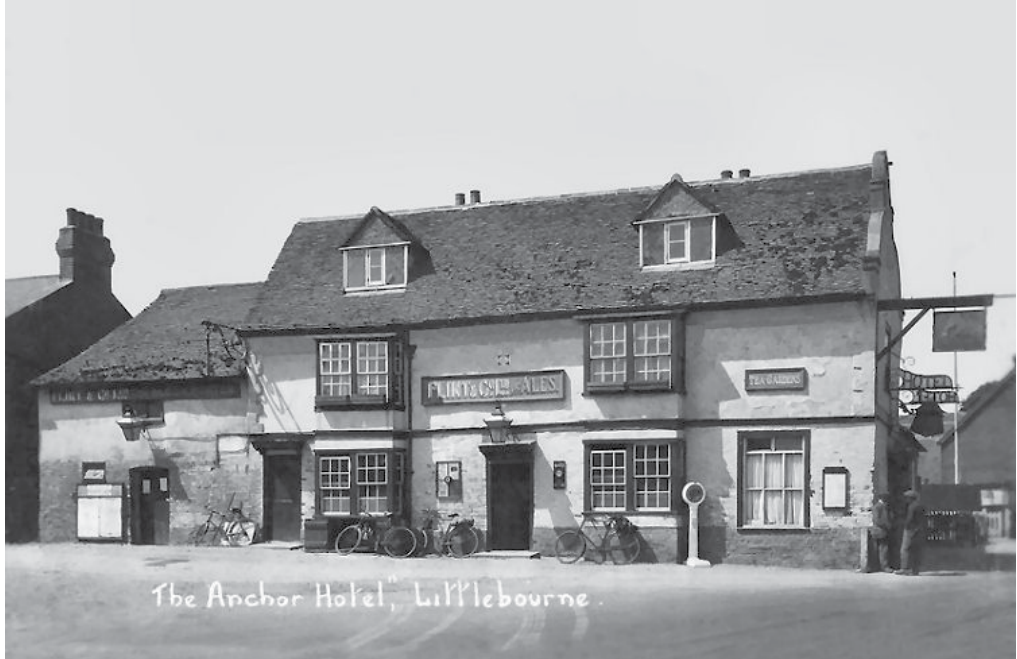
1910 Photograph of the Anchor Inn (source: http://www.dover-kent.com/Anchor-Littlebourne.html )
