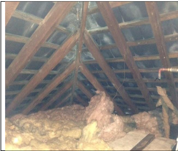
Photograph 1: Loft void showing cobwebs and internal roof structure
