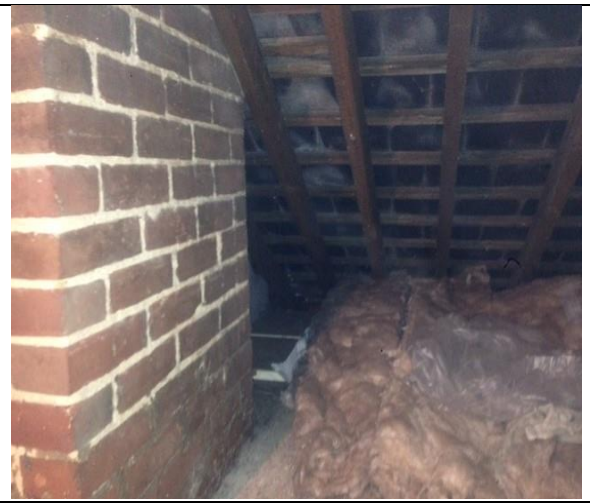
Photograph 2: Internal chimney – well-sealed
