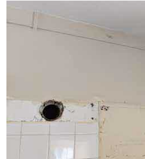
General maintenance and repair.
