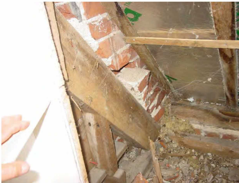
Photo showing lack of support to dormer cheek
