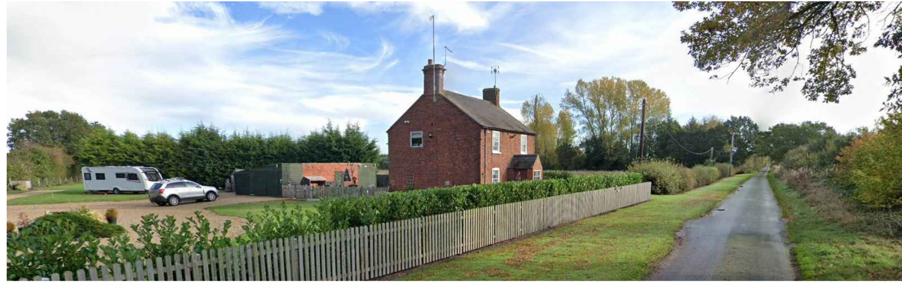
Existing view from Church Lane, West approach
