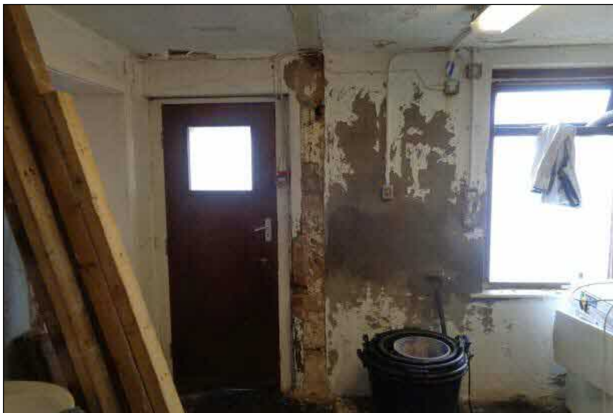
12. Late 20 th century door and window to number 1
