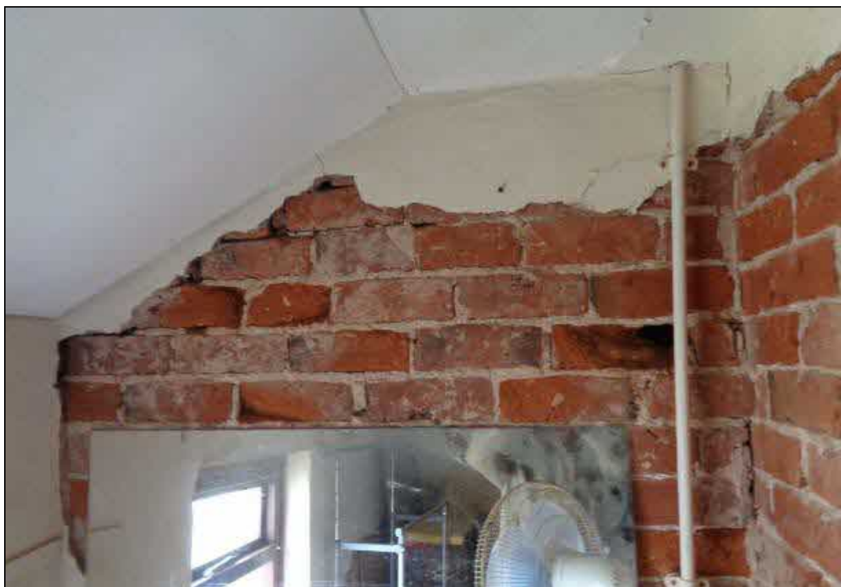
11. Exposed brickwork in number 2 appears early 19 th century
