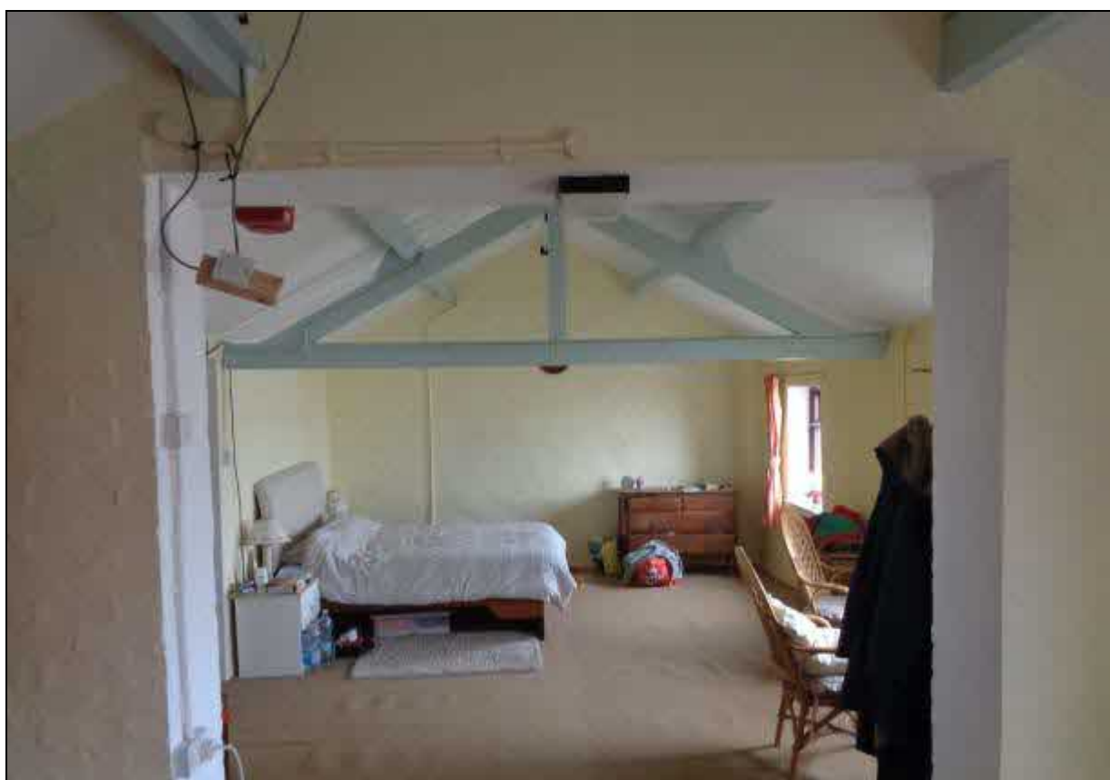
9. First floor also opened up; truss probably early 20 th century
