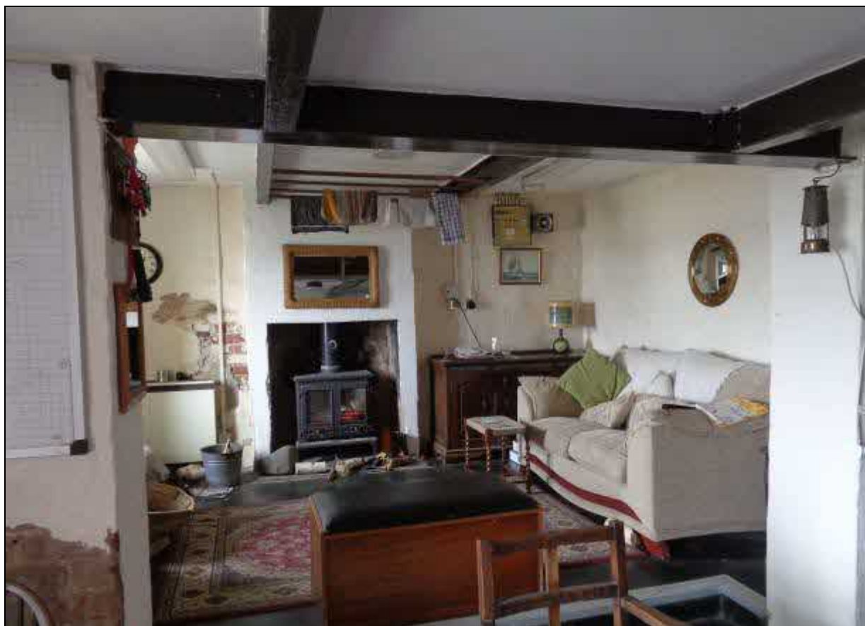
8. Number 2 has been opened up between first and second bays
