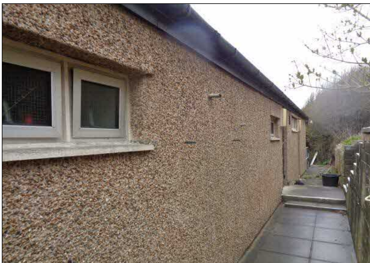
7. Extension is largely blank and has an institutional appearance
