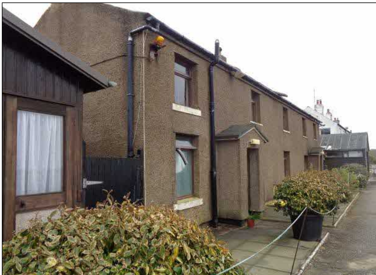
1. The application site comprises a pair of semi-detached cottages
