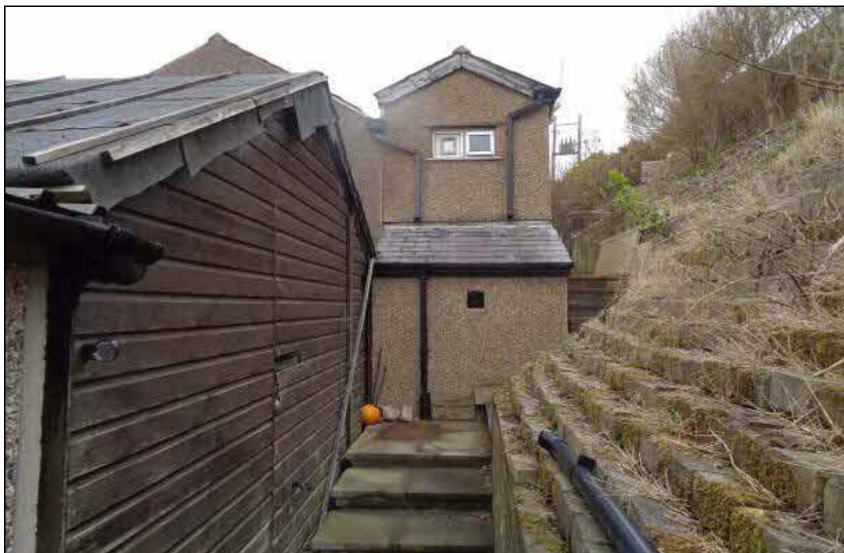
6. Rear view showing the extension
