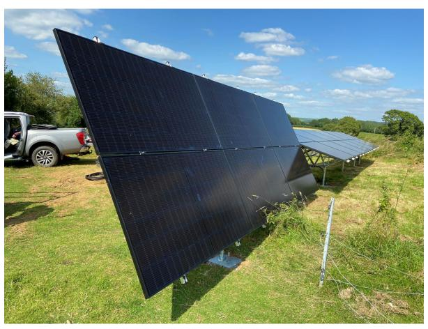
The photo shows an example of what is being proposed at Cleave House using similar black framed solar panels. The 2 frames will be approximately 100mm apart from each other in one rows of 16 panels. They are going to be in South orientation as per the scale drawing so the array will not be seen from the main house. No concrete will be used at all in the installation and this British system can be easily dismantled and recycled at the end of its useful life.
