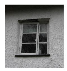
Upper left hand window to rear elevation serving bathroom. Window constructed in softwood with timber cill. Single opening casement with fixed panes glazed directly into frame jambs. Opening light fits poorly and has been poorly modified since installation leading to significant draughts. Despite ongoing repairs, there is rot to the inside of the frame due to continuous condensation.
