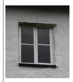
Upper right hand window to rear elevation serving bedroom. Window constructed in softwood with timber cill. Single opening casement with fixed panes glazed in to matching fixed light. Due to historic building movement there are large gaps around the opening light which fits poorly. Regular condensation necessitates regular ongoing maintenance. This is the pattern of window it is proposed to use for the 3 replacement windows.
