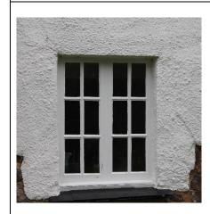
Lower right hand window to rear elevation serving kitchen. Window constructed in softwood with tile cill. Both lights fixed as window inaccessible from inside of property due to kitchen worktop and reveal depth. Most recent localised repairs to window undertaken in 2018. Magnetic secondary glazing fitted to internal frame to reduce heat loss and condensation.
