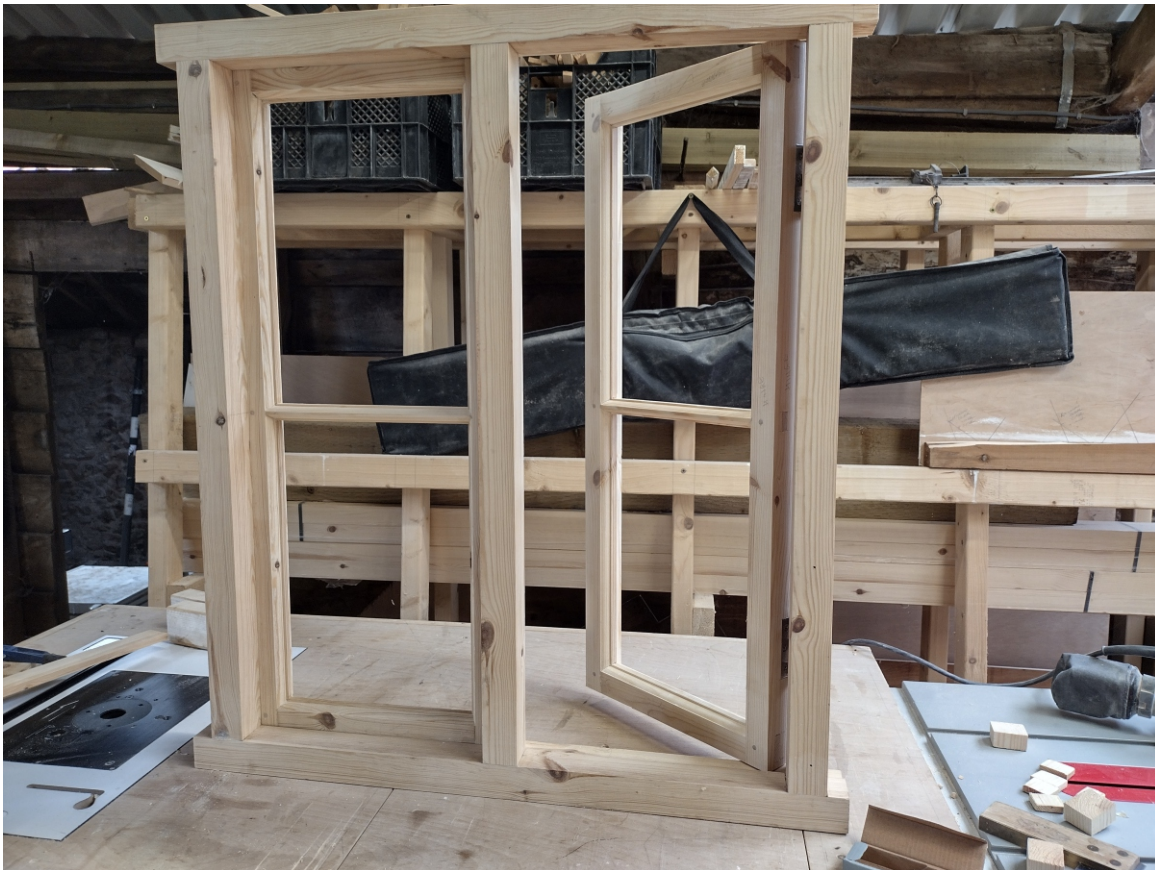
Interior view showing ovolo moulding to match existing
