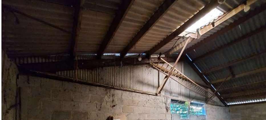
7.7 Internal view of West gable elevation showing original opening partially infilled
