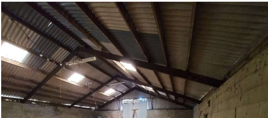
7.6 General internal view of barn structure looking East
