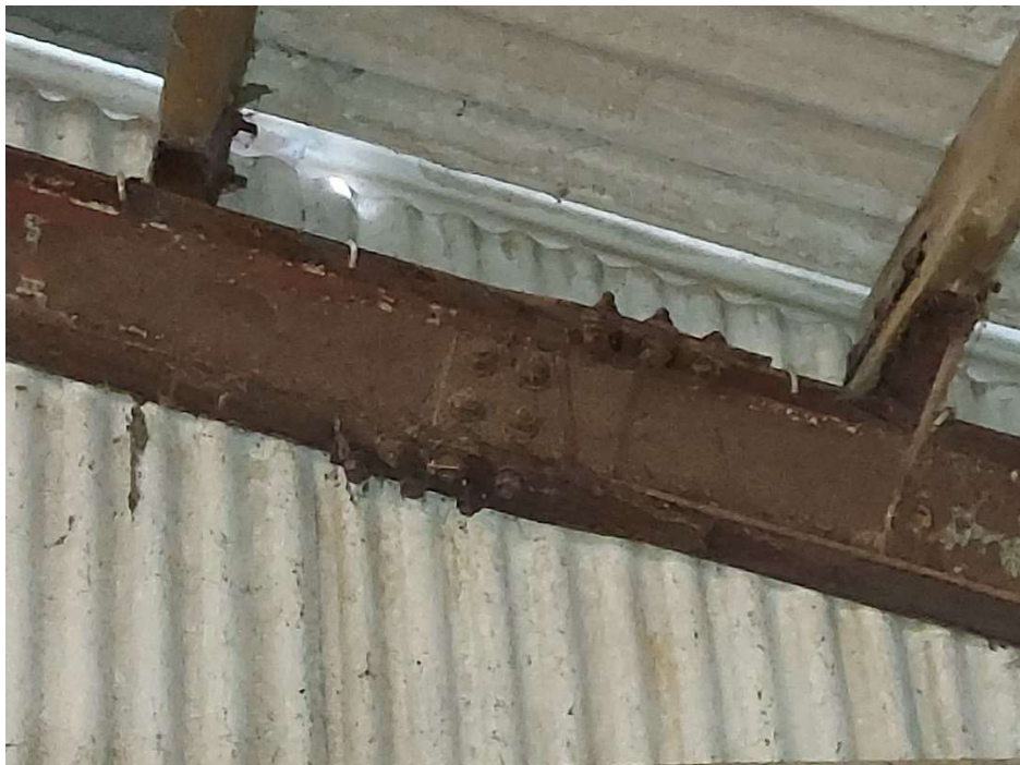
7.8 Detail of existing splice to steel rafters
