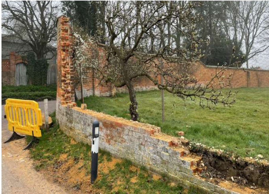
Fig 2. Collapsed wall.
