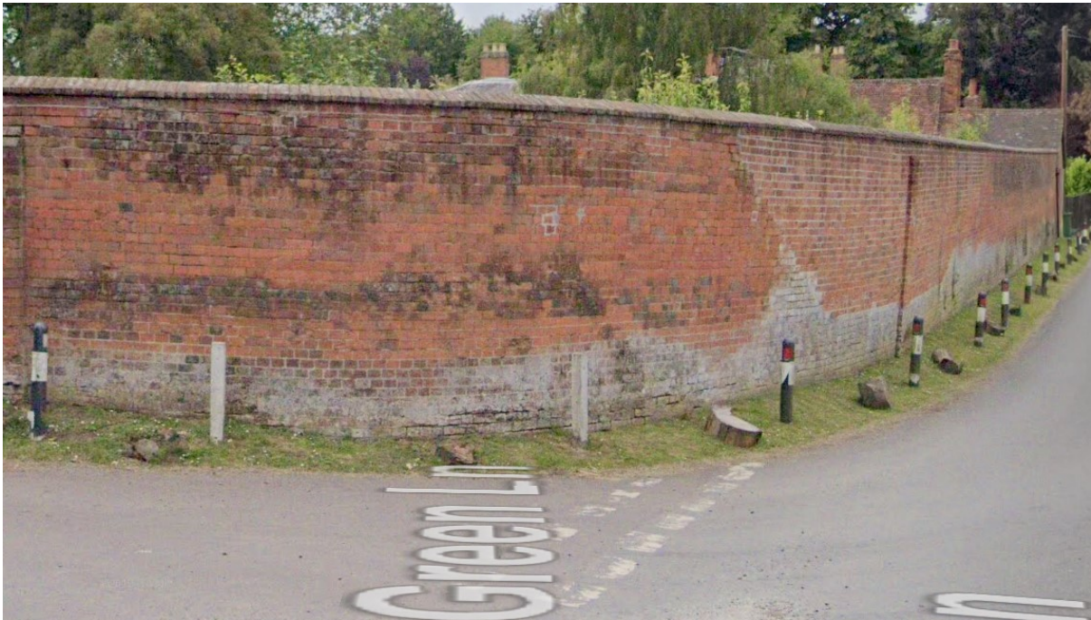
Fig 1. External elevation to original perimeter wall of Hartley House, RG27 0AJ
