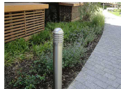
Bollard lighting is bat friendly
