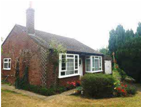
Photo 1. View north of front elevation of bungalow. Most windows on these sides are uPVC framed. Tarmac drive and slabs next to house. Conifer and small shrub bed in front of house
