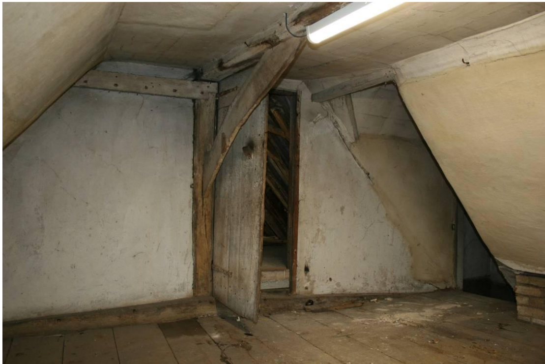
Looking S in the Attic Room. Note the crown post roof.
