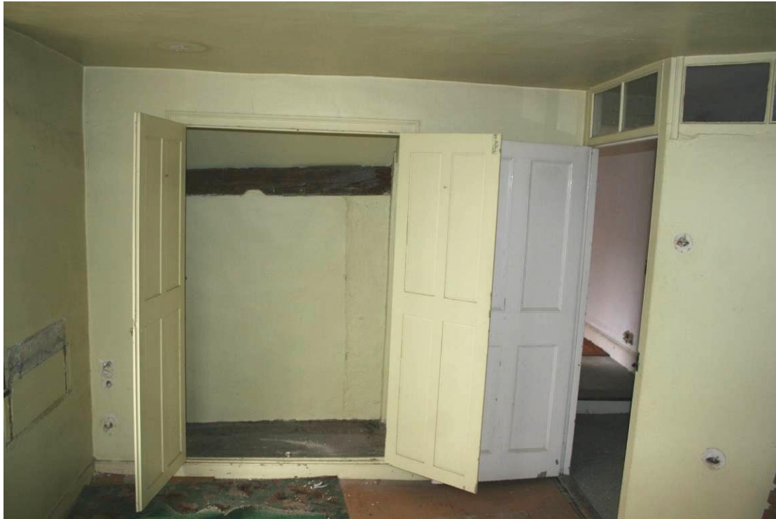
Looking N at the built in 1950's style closet.
