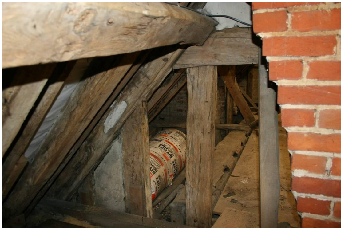
Looking E in the roof over the Rear Cross-wing Bedroom 5.
