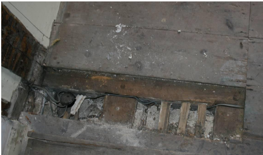
The first floor frame by the storey post.
