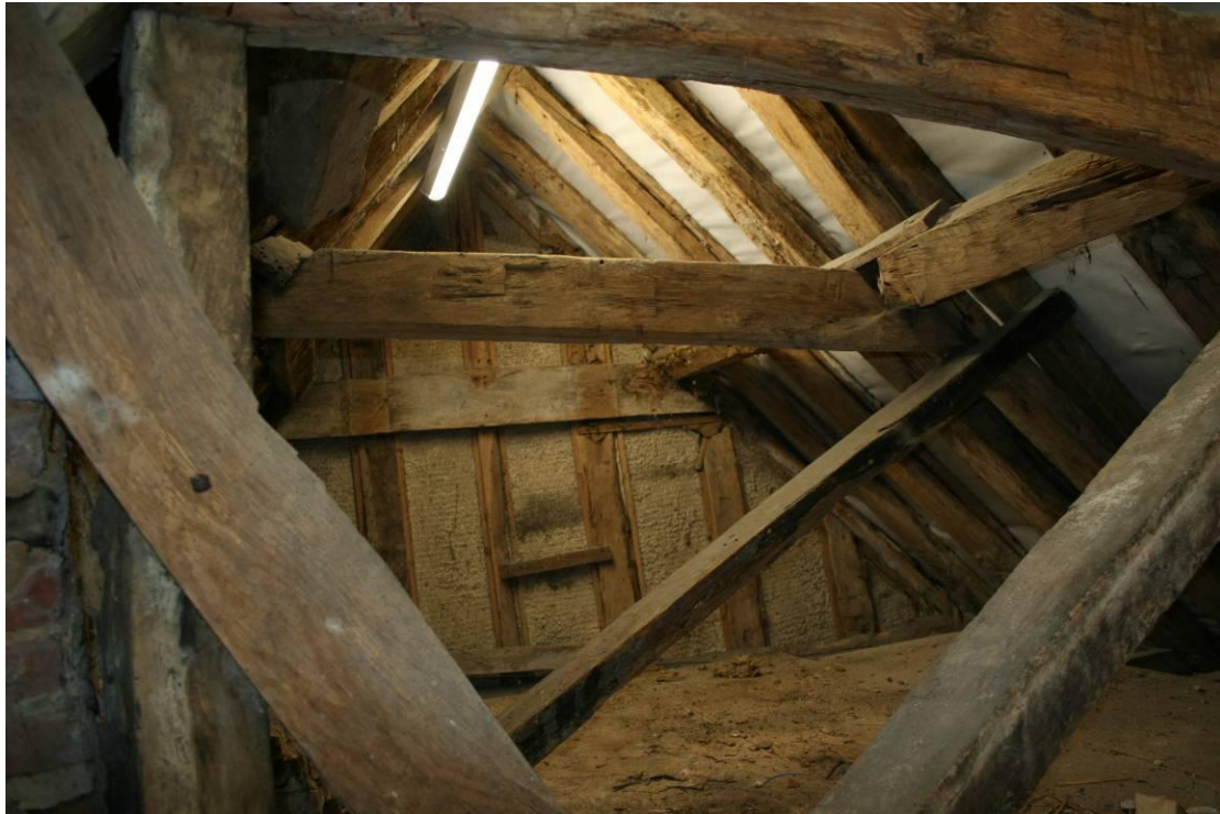
Looking NE in the Cross-wing over Bedroom 5.
