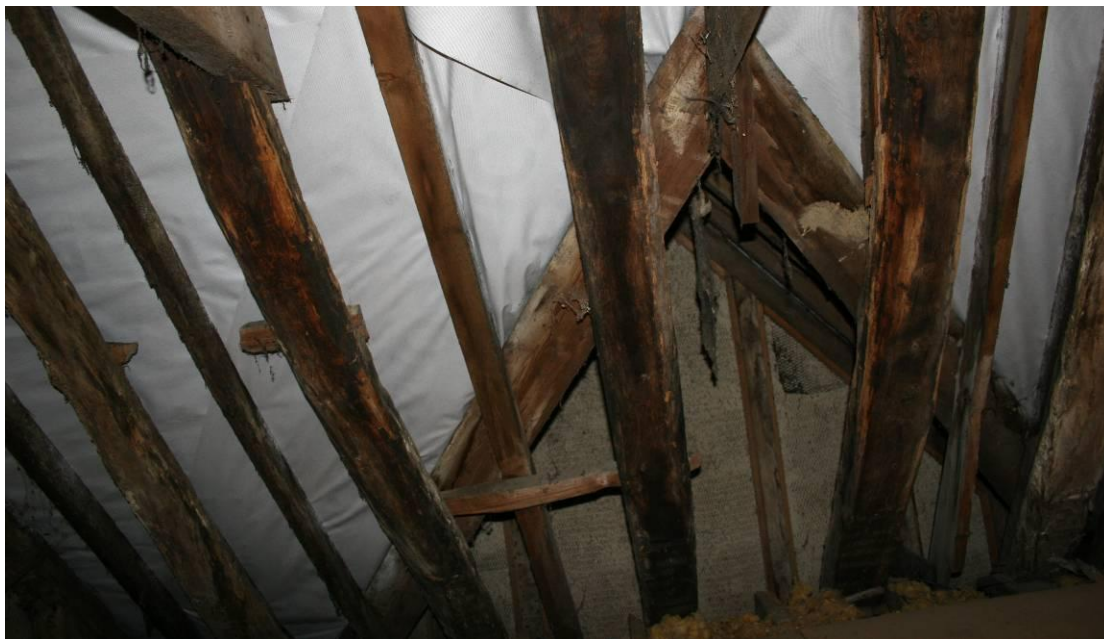
Original flat rafters with C20th gable beyond.
