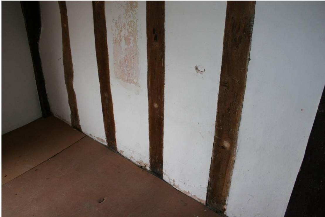
Fixture holes and multiple taper burns.
