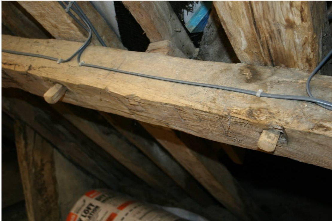
Bolt headed pegs in the purlin.
