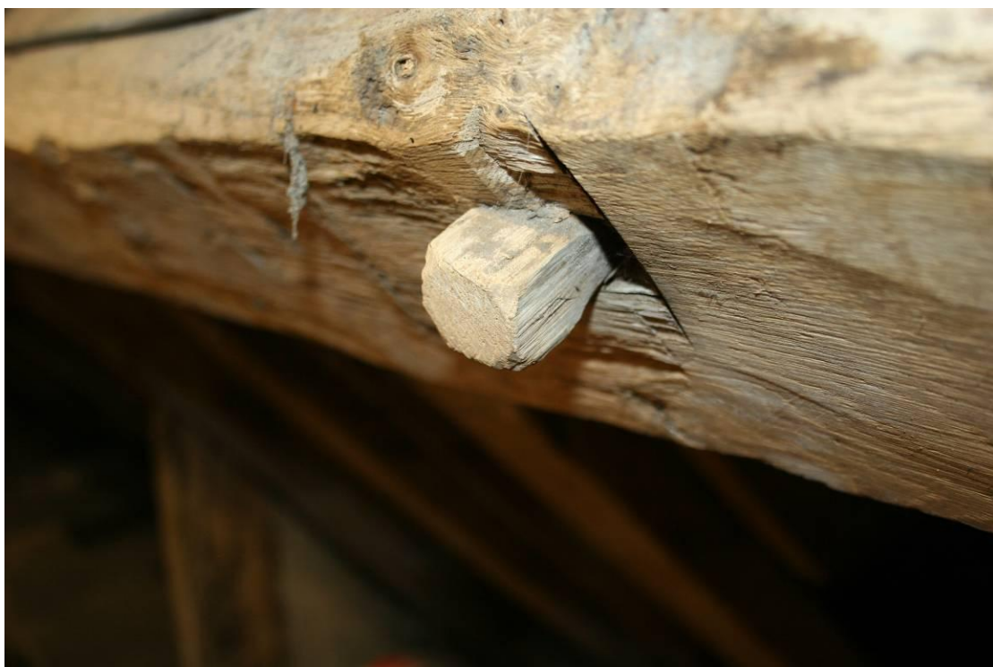
Detail of a bolt headed peg.
