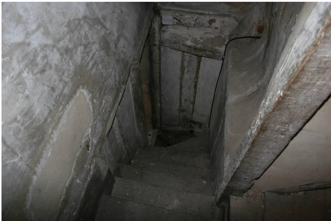
Looking down the attic staircase.
