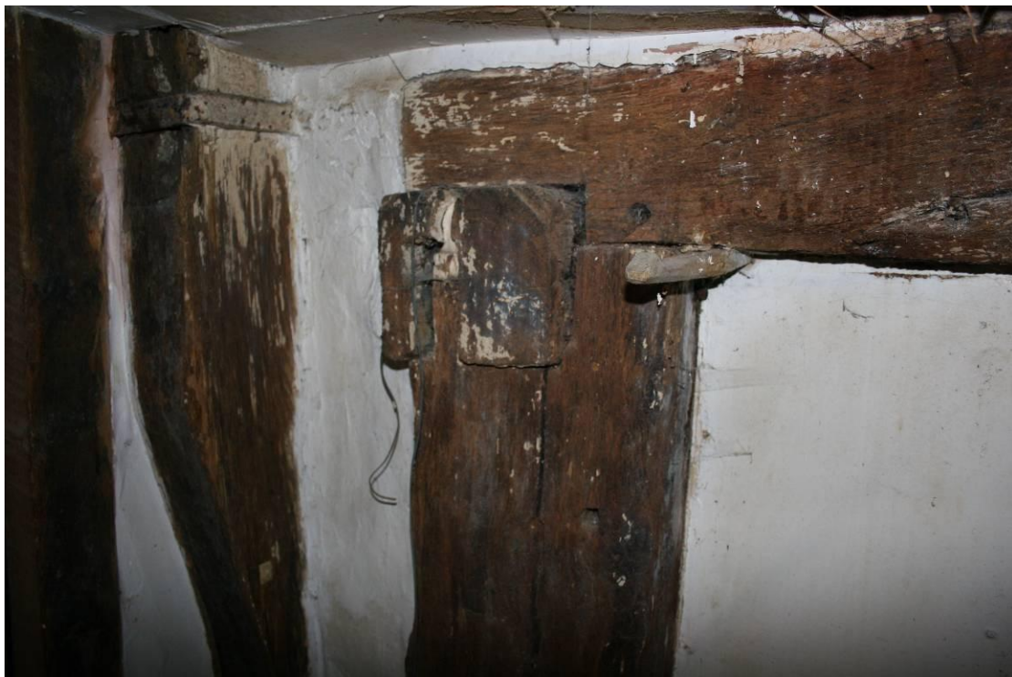
The cross-wing frame has been sawn off to insert the firestack.
