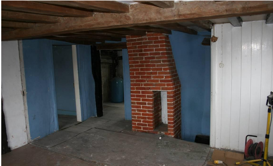
Looking W in the North Bedroom 1.
