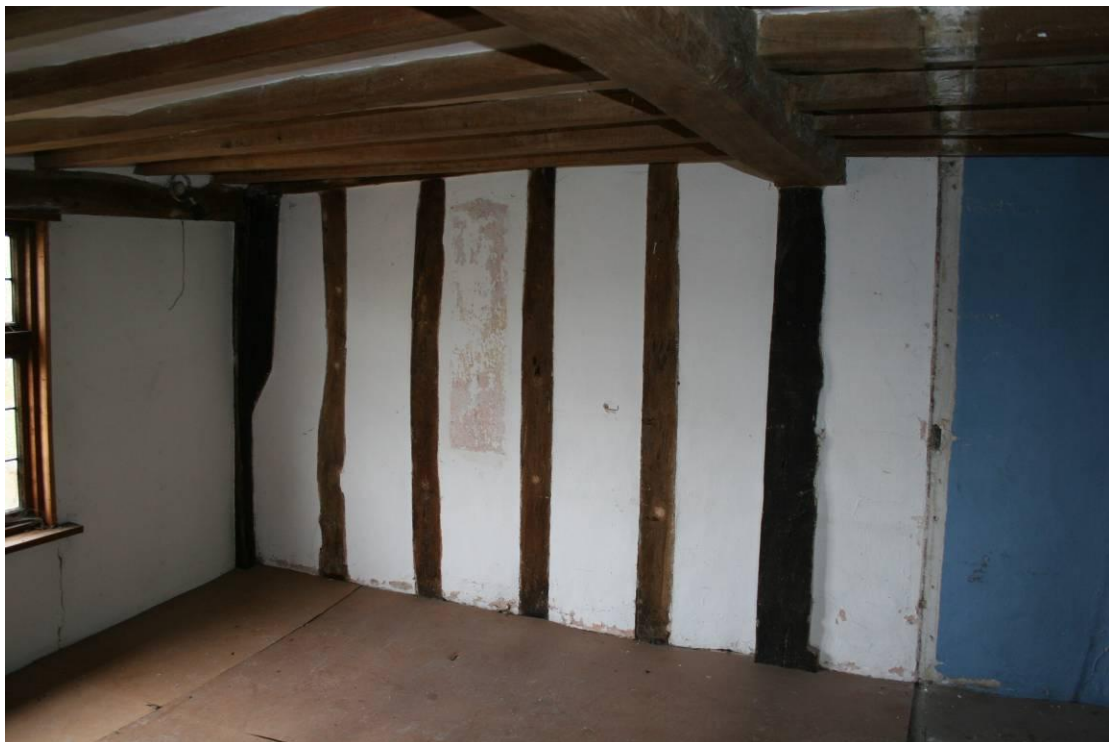
Looking SE at the partition wall in North Bedroom 1
