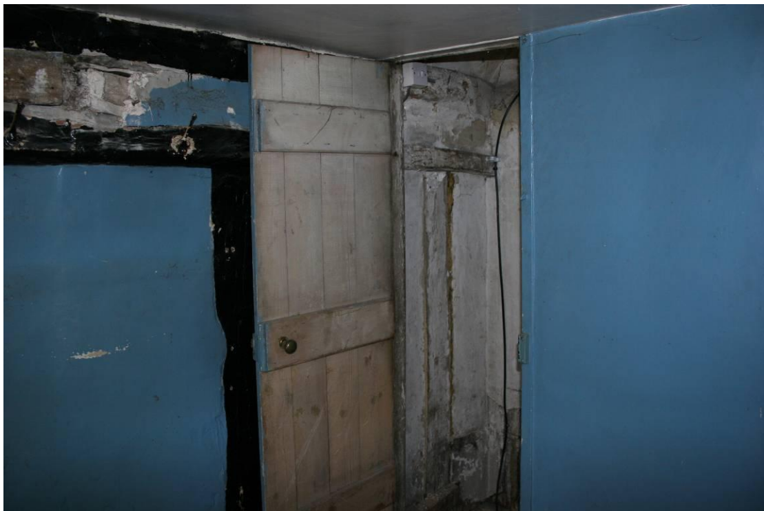
The exposed frame in the attic staircase. Looking NE.
