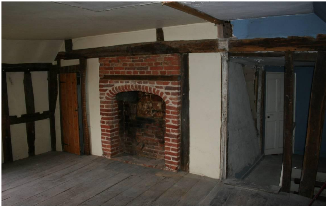
Looking SE in Central Bedroom 2 .
