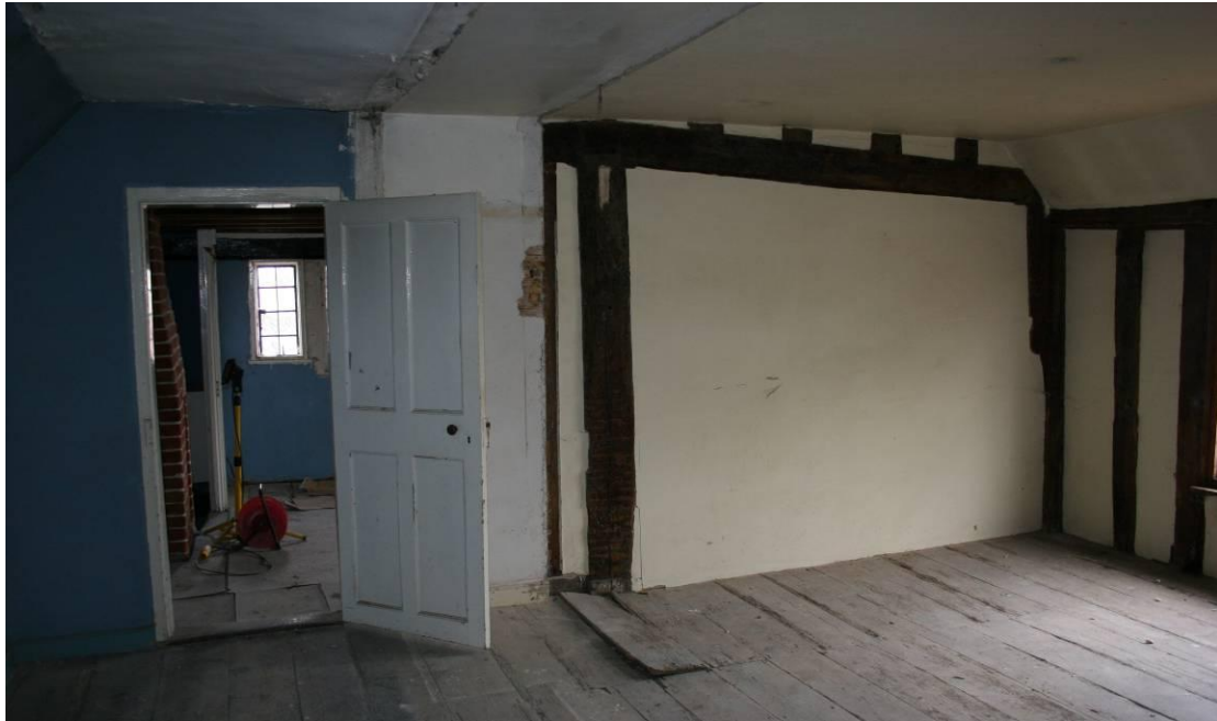
Looking NE in the Central Bedroom 2 from the main staircase.
