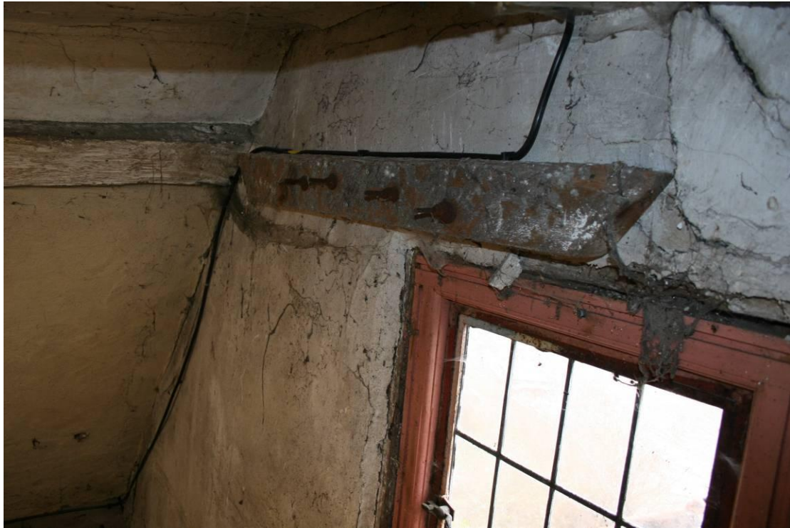
Historic repairs to the north wall.
