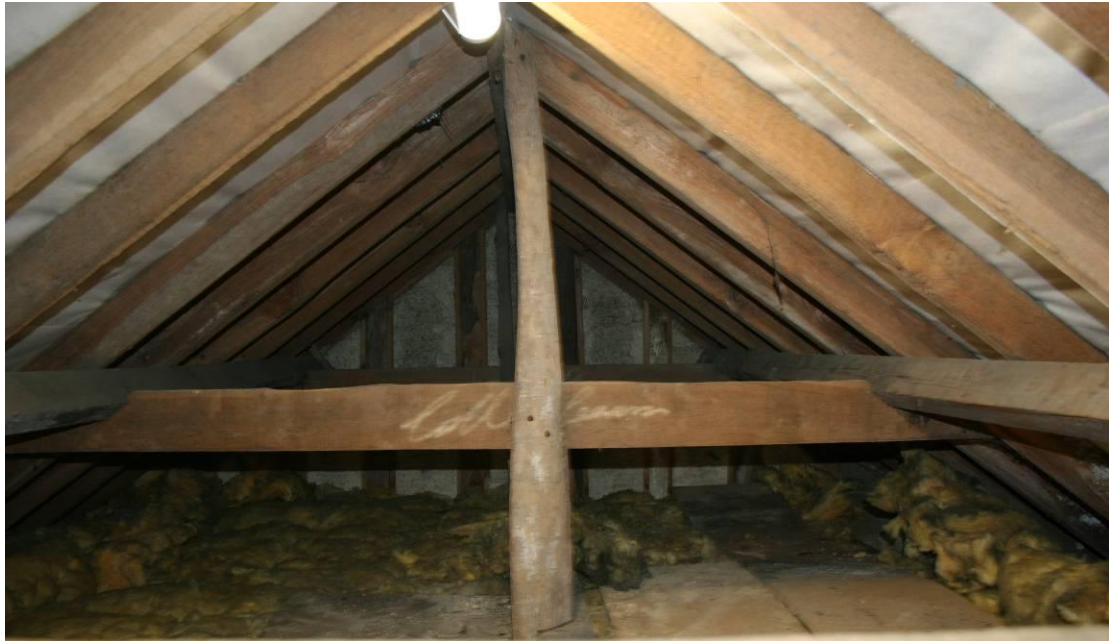
Looking W in the roof over the central extension.
