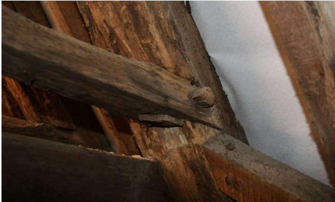
Detail of one of the side lapped collar purlins.
