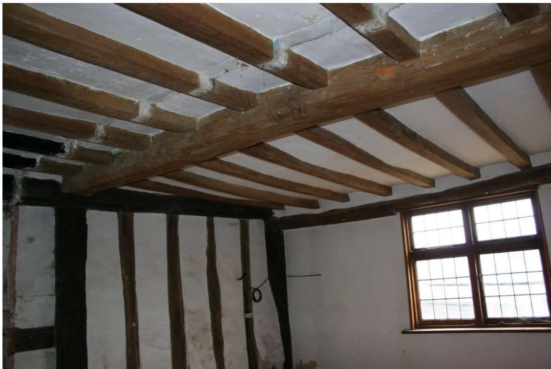
Detail of the attic floor frame.
