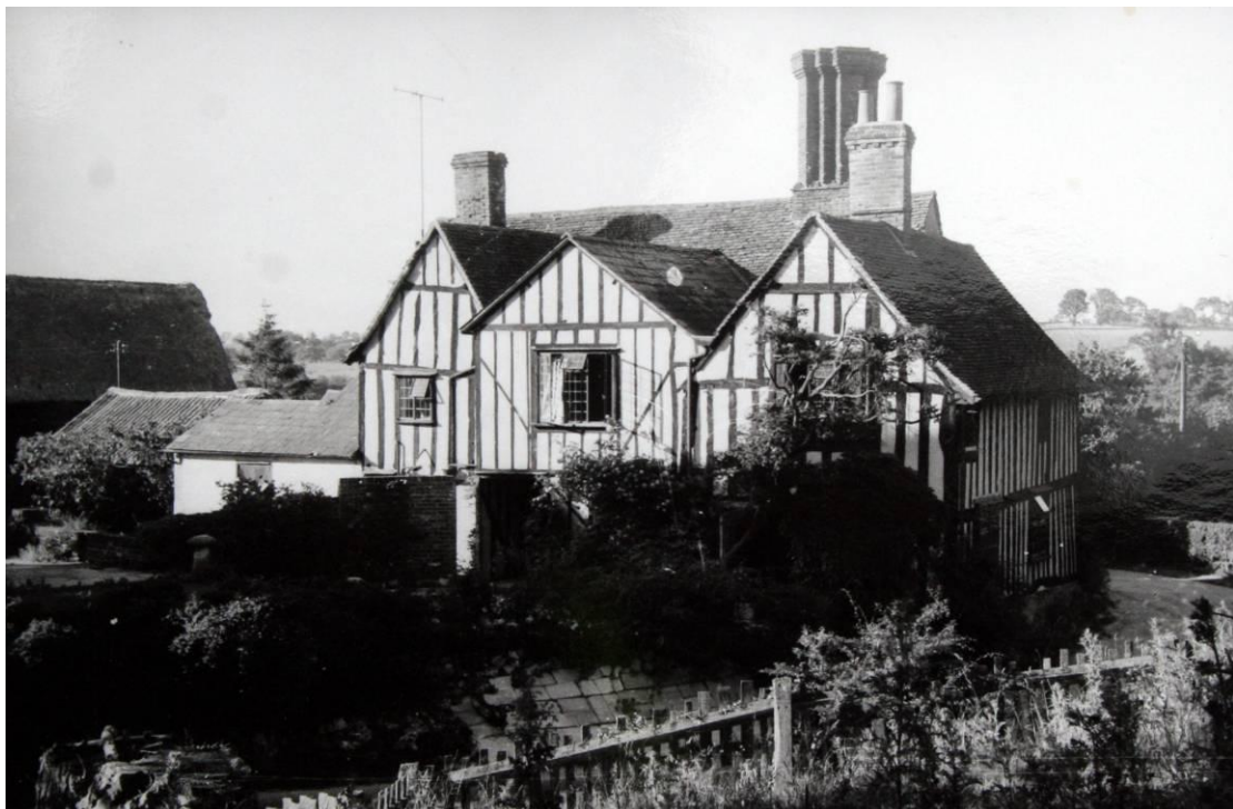
1960's (undated). Ancells, Barn and Garage from the SW.
