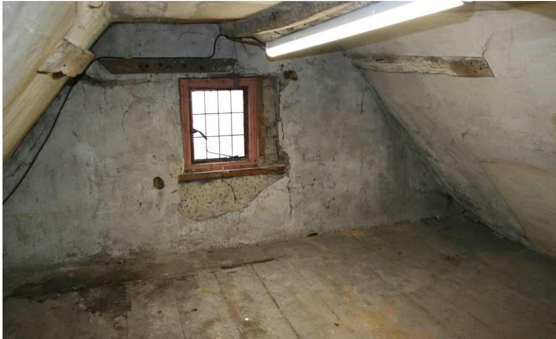
Looking N in the Attic Room.
