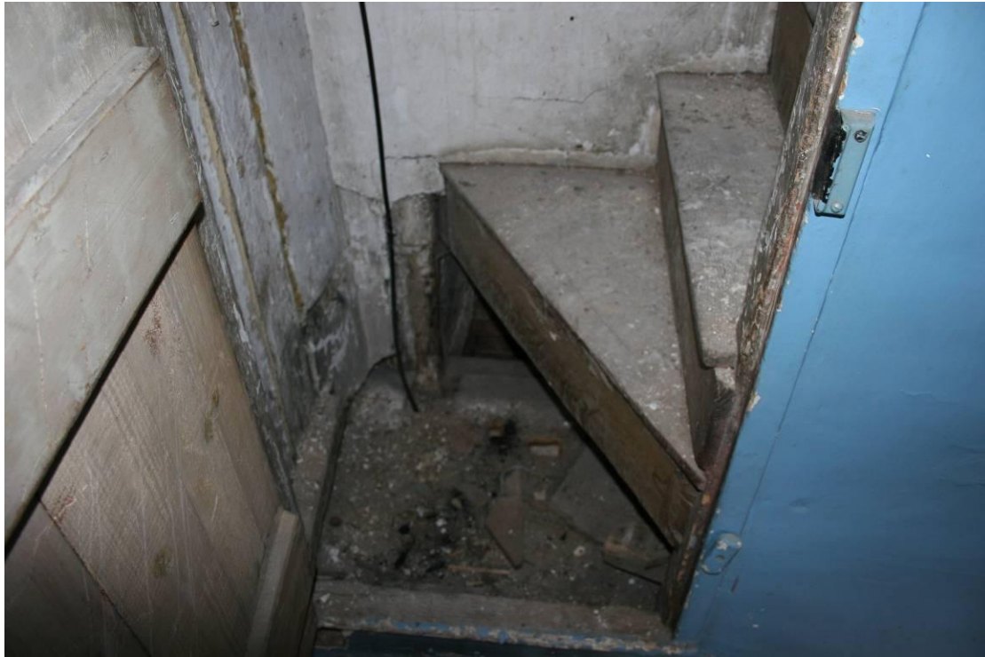
The attic staircase.
