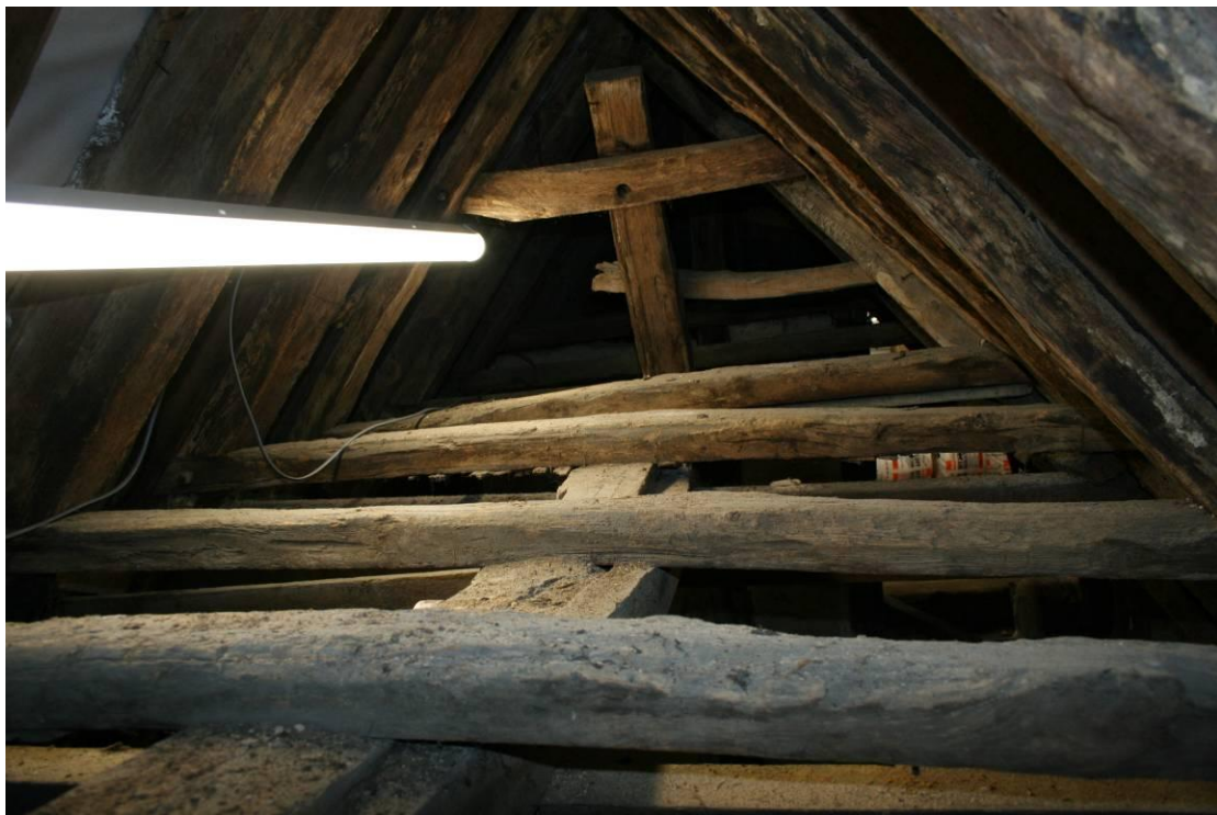
Looking S over the collar purlins. The upright is part of a hipped reinforcement.
