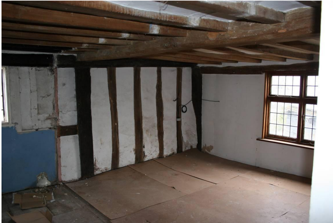
Looking NE in the North Bedroom 1.
