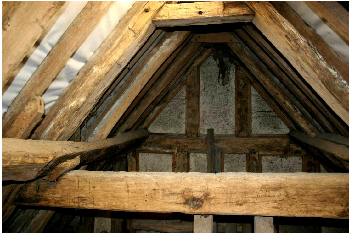
Looking W in the roof over the Rear Cross-wing Bedroom 5.
