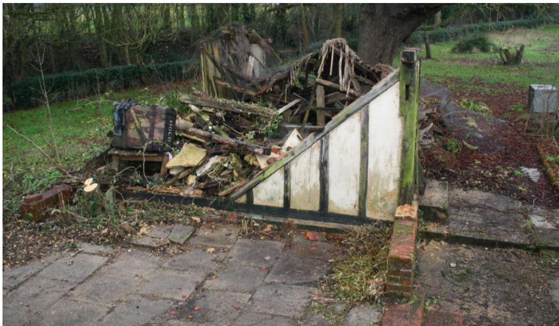
2021. The east elevation of the Summer House.
