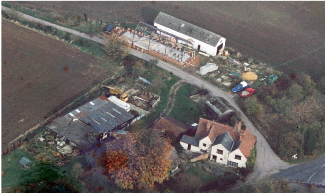
2000's (undated). Ancells from the SW. The Summer House has deteriorated.
