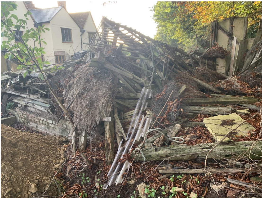
2022. Looking SE at the Summer House. Andrew Stevenson Associates.
