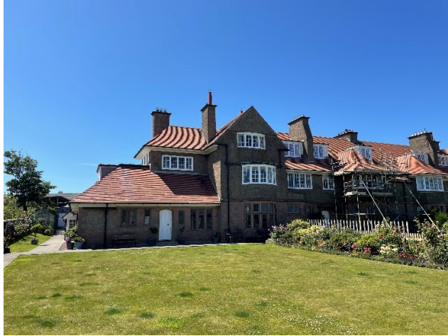
Property from front (West)
