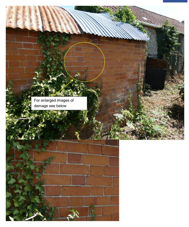
Photo 5 - South west corner - Stair stepped cracking
