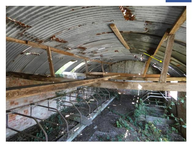
Photo 10 – Interior view – Damaged / missing roof sheets and sagging beams
