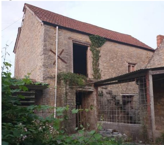
Figure 4 Photos of barn 'B'
