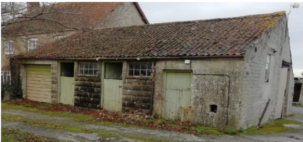
Figure 3 Photos of barn 'D'
