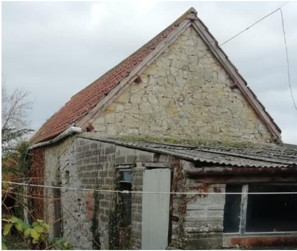
Figure 5 Photos of barn 'C'
