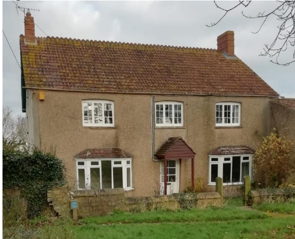
Figure 2 Photos of house 'A' from south and east
