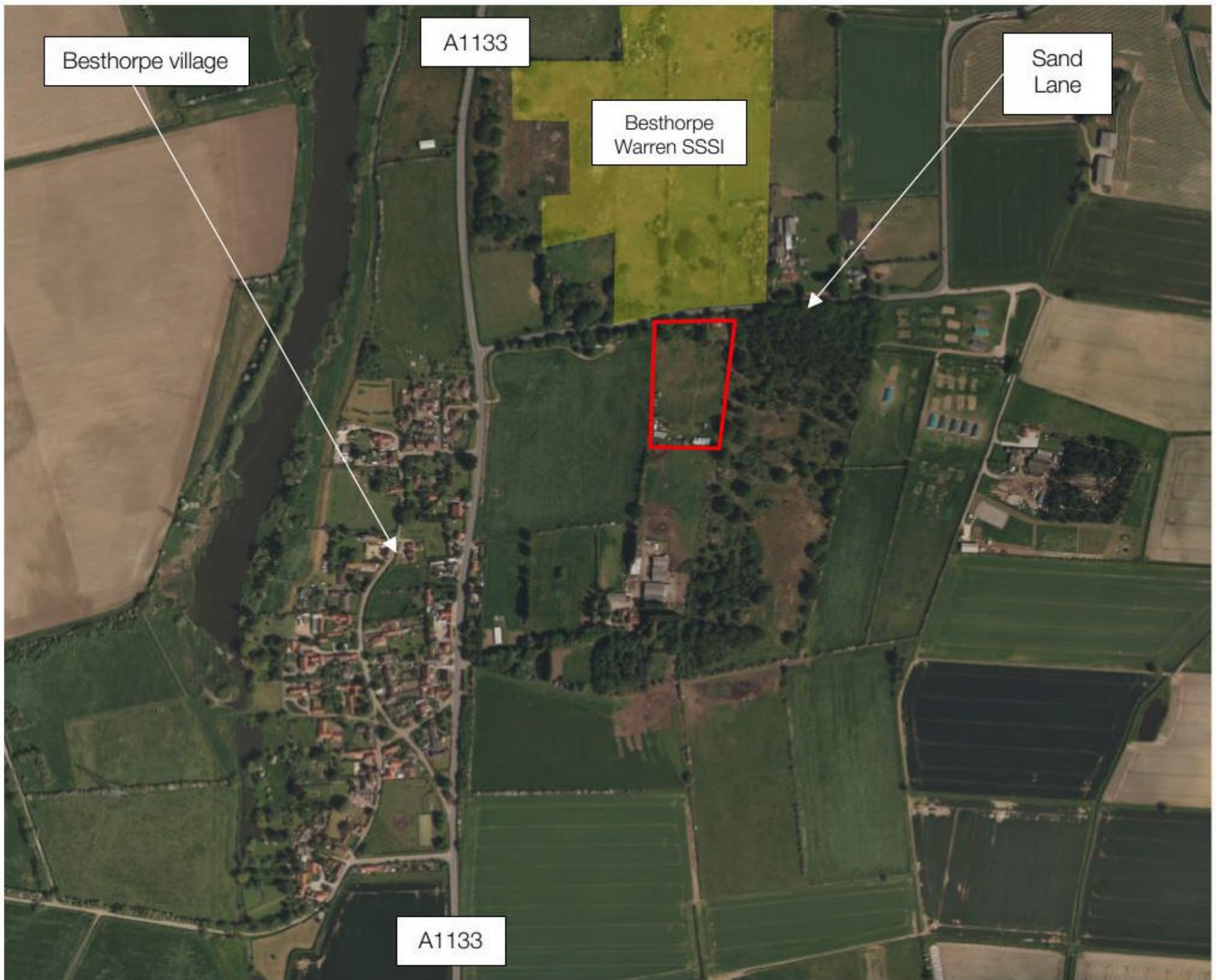
Aerial photograph identifying the location of the application site
