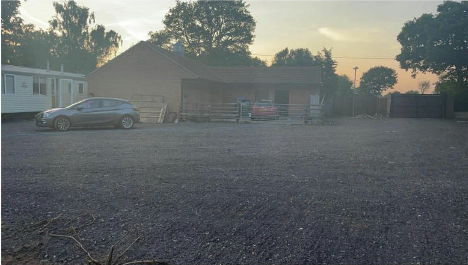
The stable building (looking from within site towards Sand Lane)
