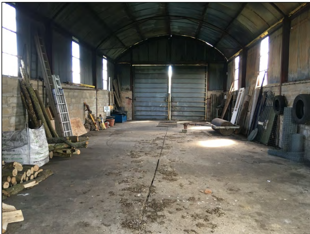
Photograph 10: Inside Harleston Hall Barn, from the western end.
