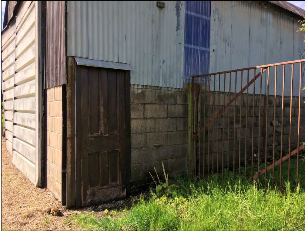
Photograph 5: A door on the north-eastern corner of Harleston Hall Barn.
