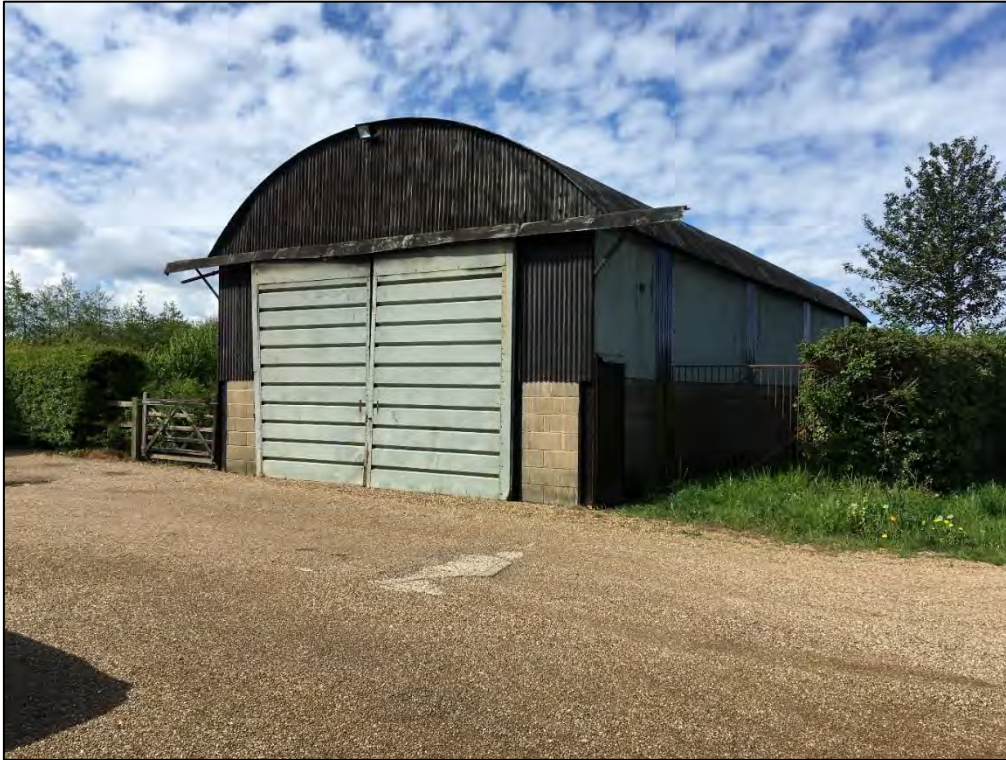
Photograph 1: Harleston Hall Barn from Haughley Road.
