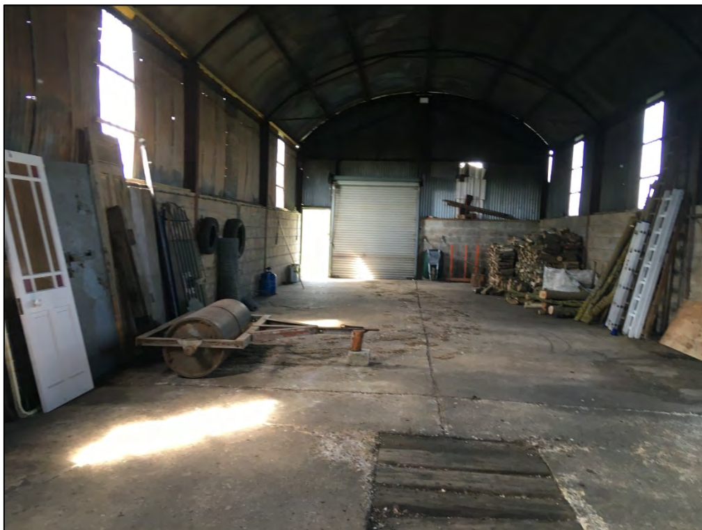
Photograph 12: The inside of Harleston Hall Barn, from the eastern end.
