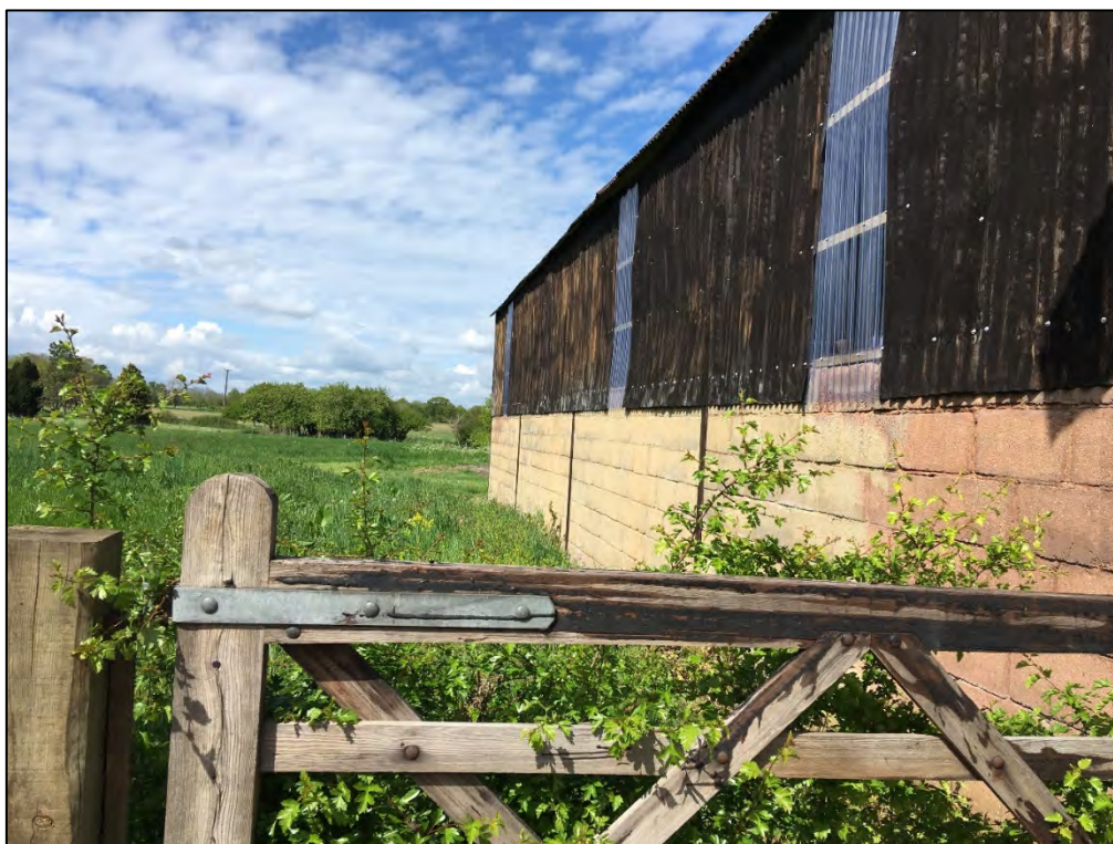
Photograph 6: The southern side of Harleston Hall Barn.
