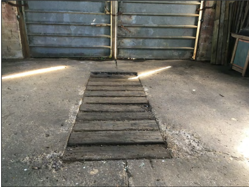
Photograph 11: The inspection pit (infilled) at the eastern end of Harleston Hall Barn.
