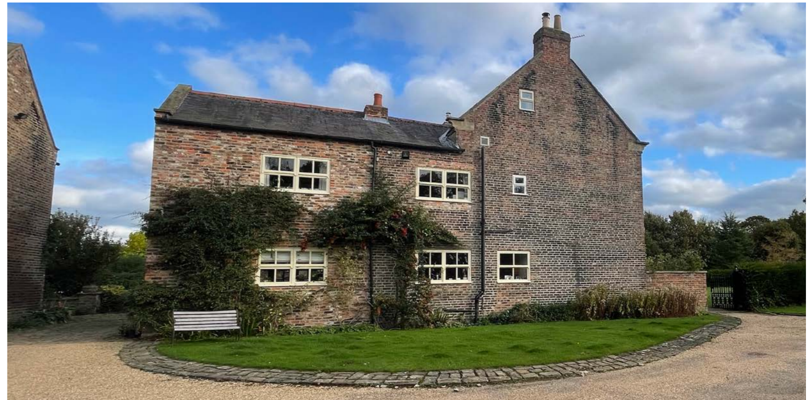
View 2 - looking towards the side gable of the farm house on approach from Grange Lane
