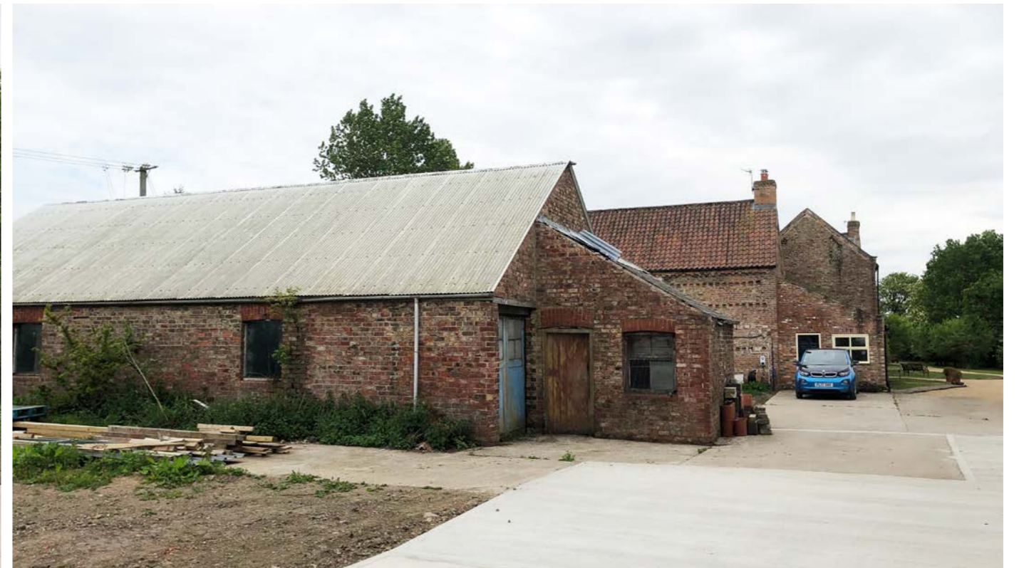
View 6 - the former unused Agricultural Barn (B5)
