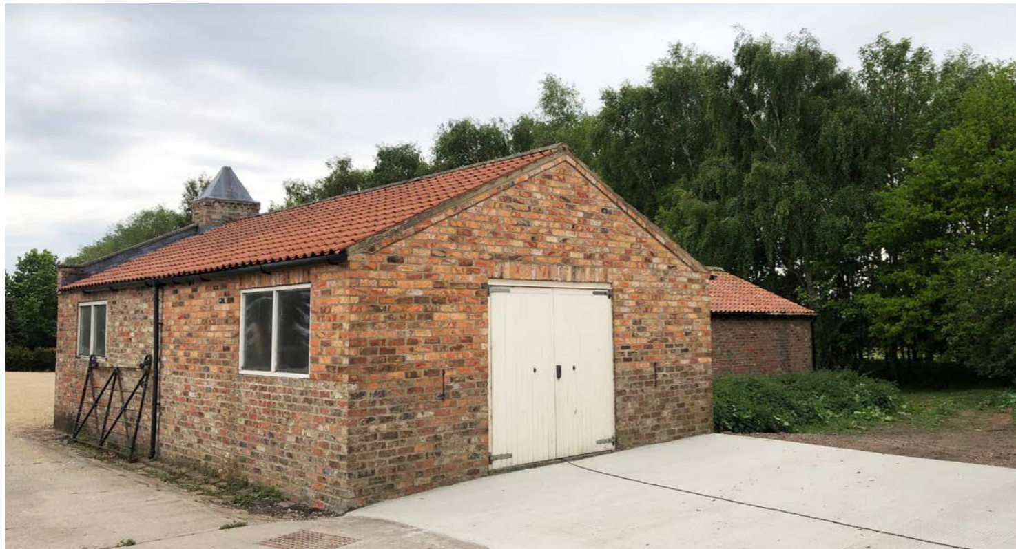
View 3 - looking towards the existing garages (B4)
