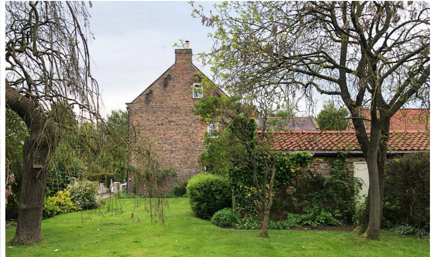
View 4 - View looking towards the low quality lean to (barn 3d)
