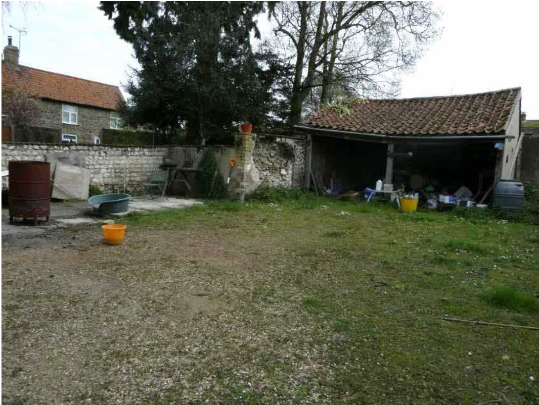
Photo 1, looking northeast across the site towards the western boundary wall.
