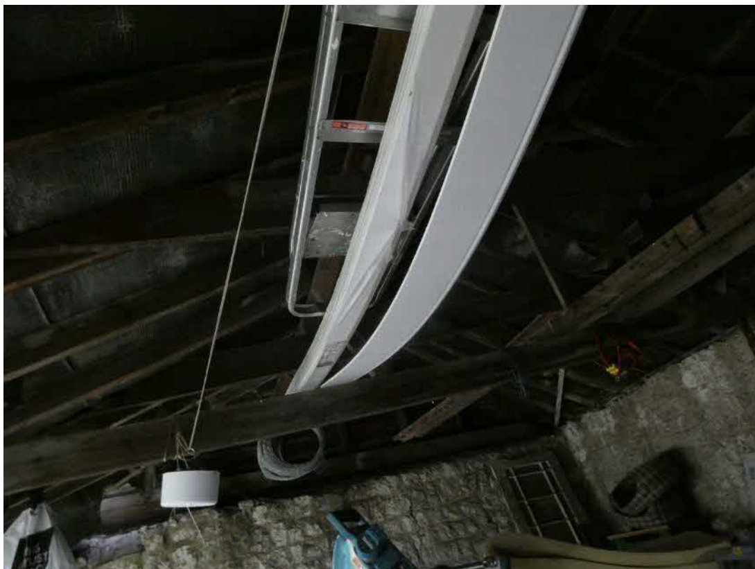
Photo 13, internal view of the carport.
