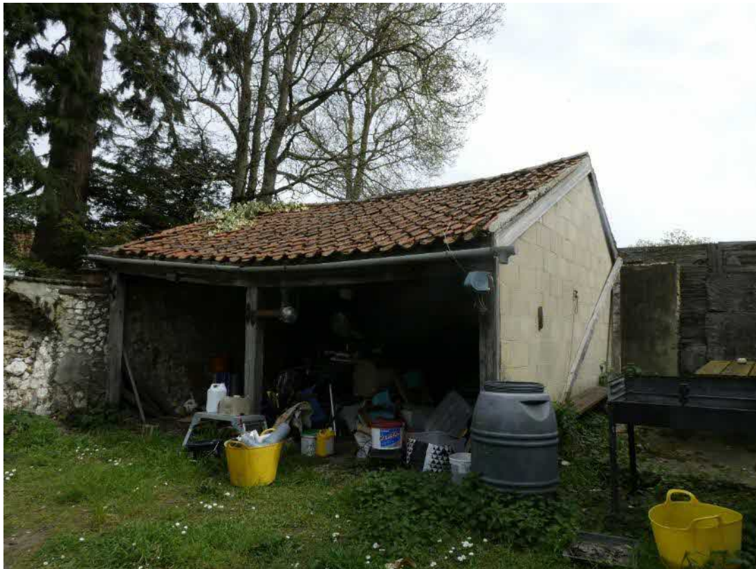
Photo 12, west and south aspects of the car port, looking northeast.
