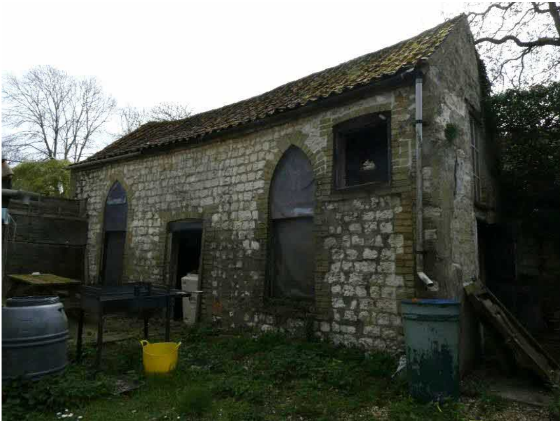
Photo 5, north and west aspects of the outbuilding, looking southeast.
