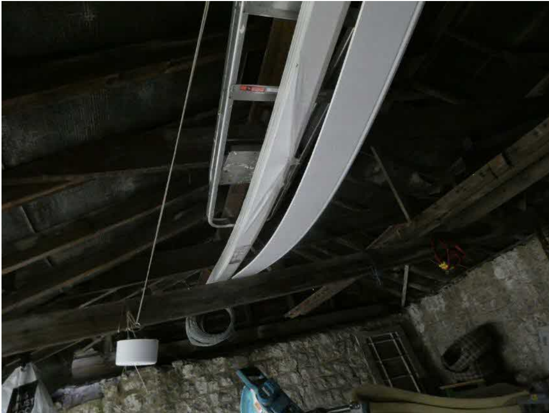
Photo 13, internal view of the carport.
