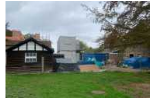
East Elevation – garage to the right
