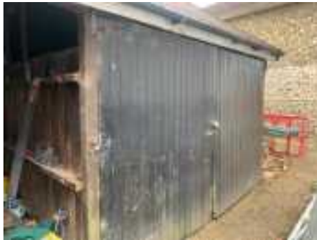
Part North Elevation – flint outhouse beyond
