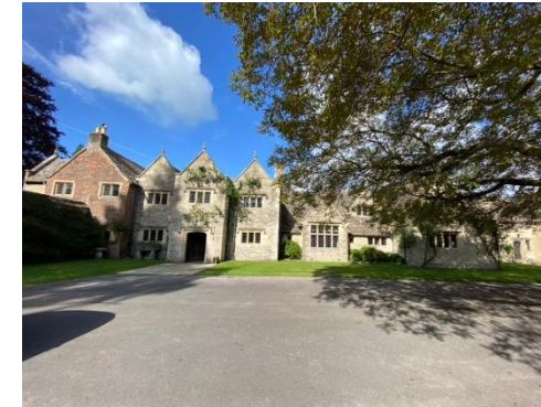
Photo P1.1 Rossley Manor House
