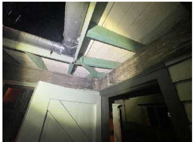
Image 6: Gaps present between the roof perlin. These are blocked with wire mesh.
