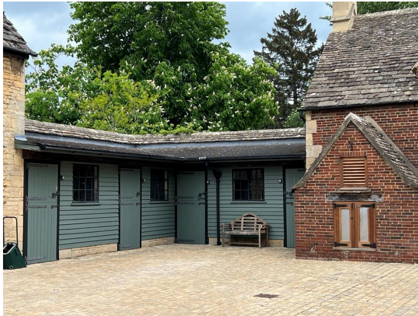
Figure 7. The existing lean-to southern stable block which will be rebuilt in timber weatherboarding to match the existing.
