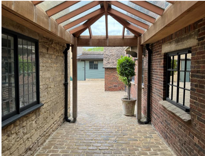
Figure 8. The glazed, covered entry passage.
