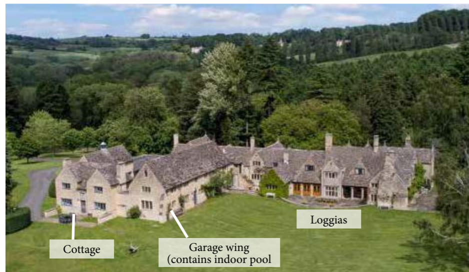
Modern view towards the western elevation with its two loggias, leading onto a terrace. The cottage and garage range can be seen to the left of the photographs.
