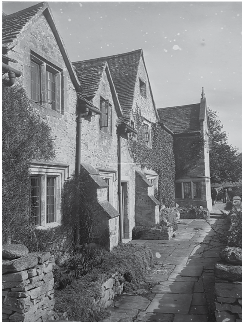
RIGHT: View of the southern elevation, taken by W. Dennis Moss, probably in the early 1920s. A terrace has been laid out along the elevation, and the new bay window is clearly shown projecting from the earlier wing.
