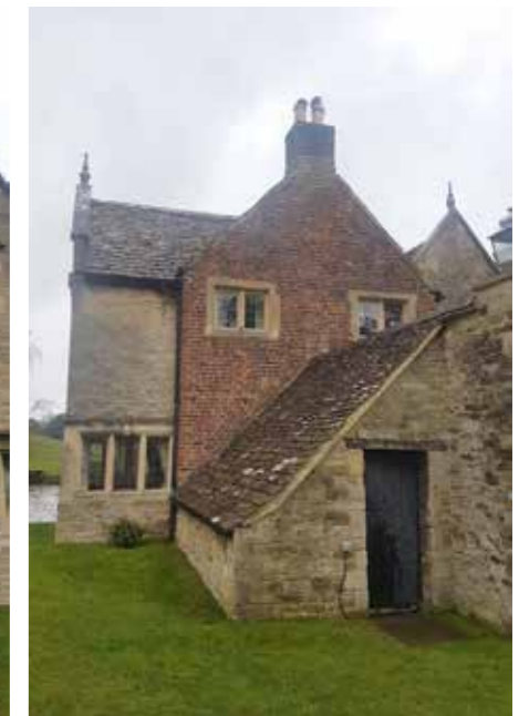
RIGHT: View of the eastern elevation where the extent of the eighteenth century brick wing can be clearly seen. The single-storey woodshed and two-storey wing both date from the early twentieth century.
