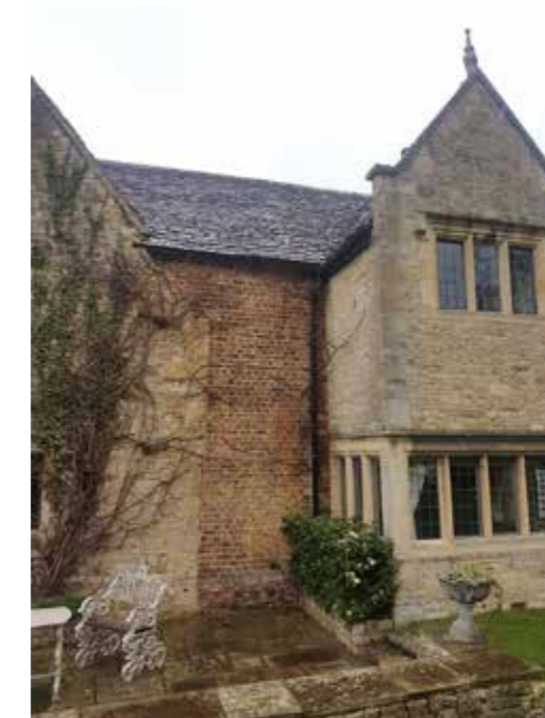
LEFT: Modern view of the eastern end of the southern elevation. The eighteenth-century extension can be seen to the right of the earlier core, and was constructed in brick. It is now largely obscured by the early-twentieth century, two-storey gabled projection, seen to the right.
